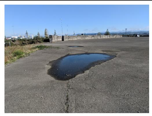
Photograph 1. Crack in asphalt and ponding on northwest side of the cap (looking north).
