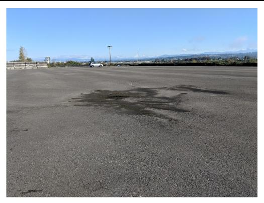
Photograph 3. Settled area with deposited dust and debris (looking northeast).
