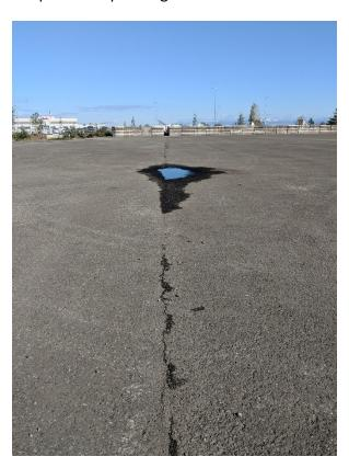
Photograph 2. Crack in asphalt through the center of the cap and ponding (looking north).
