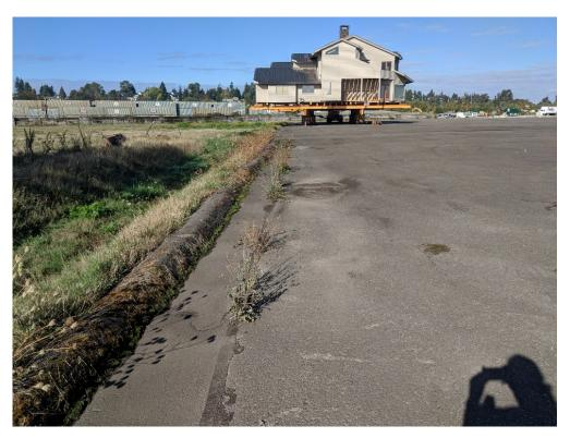
Photograph 4. Crack in the asphalt with growing vegetation along the south edge of the cap (looking west).
