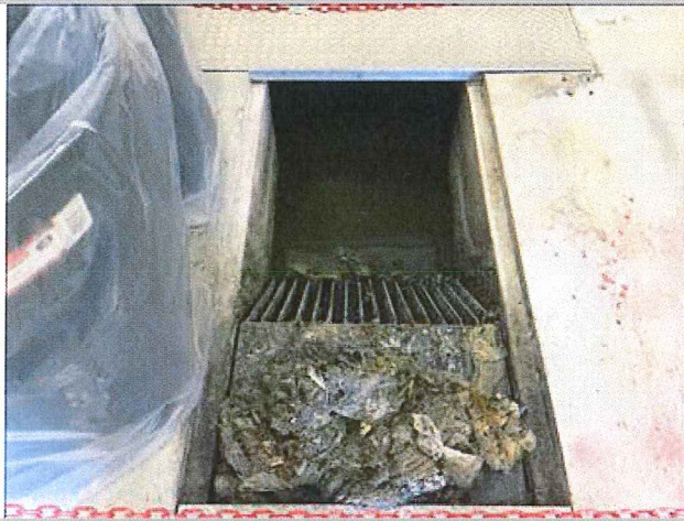
Coarse screen in the headworks.
