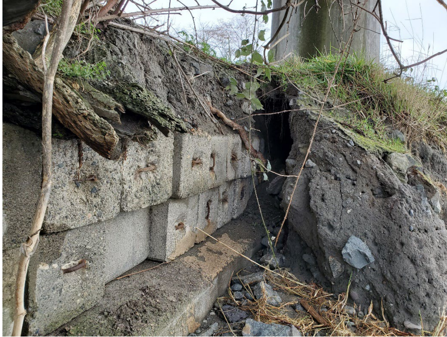
Figure 5. February 2021 damaged section of the levee between the state highway 529 overpasses.
