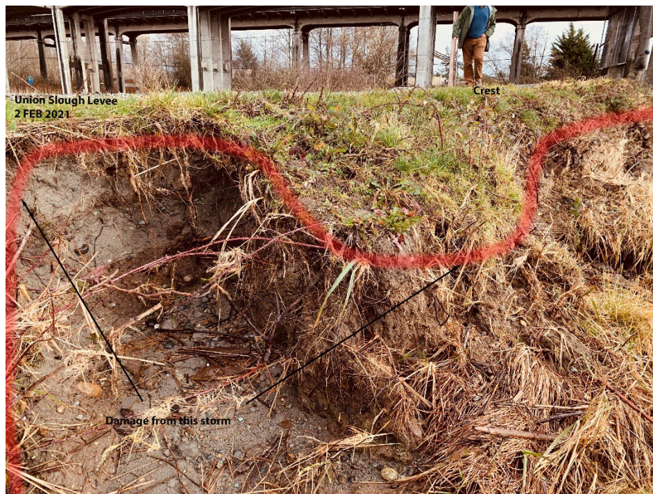
Figure 6. February 2021 flood damage (outlined in red)
