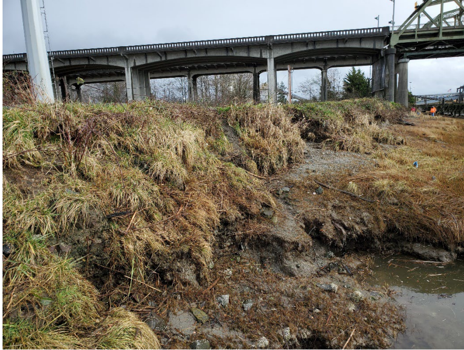
Figure 3. February 2021 documentation of flood-damaged levee.
