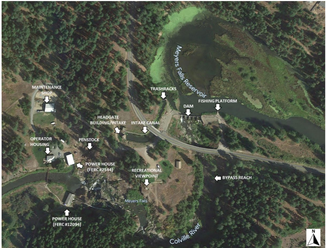
Figure 1. Meyers Falls Hydroelectric Project Facility Layout
