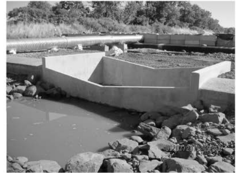
H14 PHOTO: EXISTING DOUBLE NOTCH STRUCTURE
