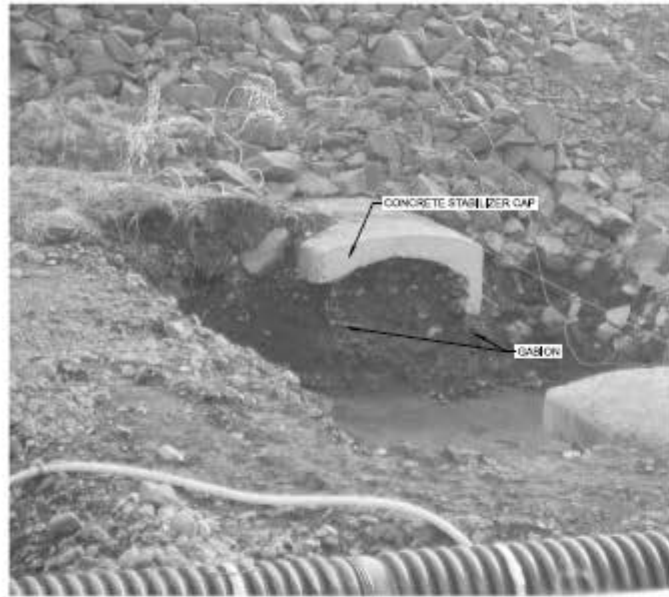
H1 PHOTO: EXISTING STABILIZER AND GABION
