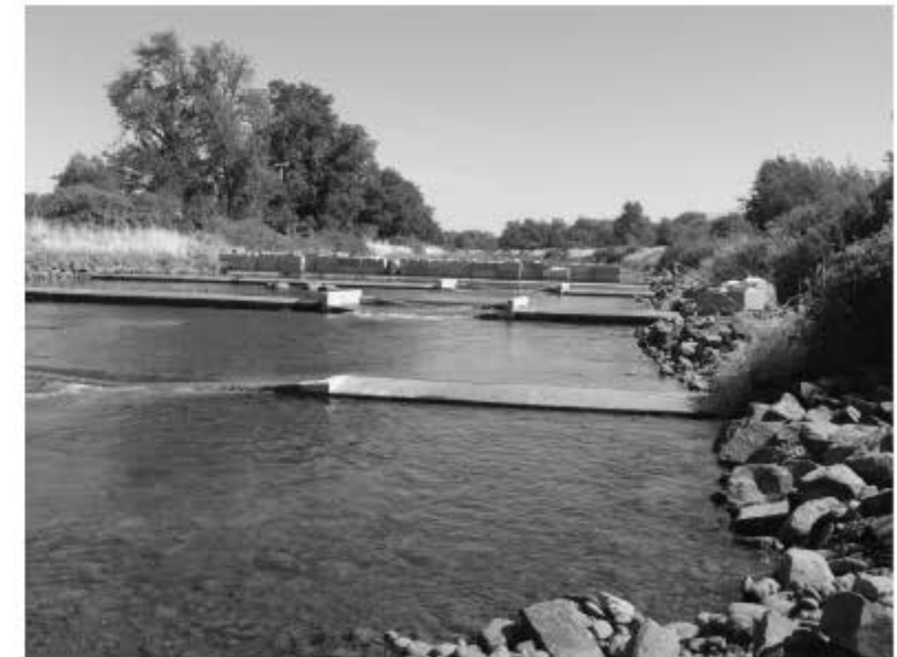
EXISTING NOTCH STRUCTURES WITH FLOW
