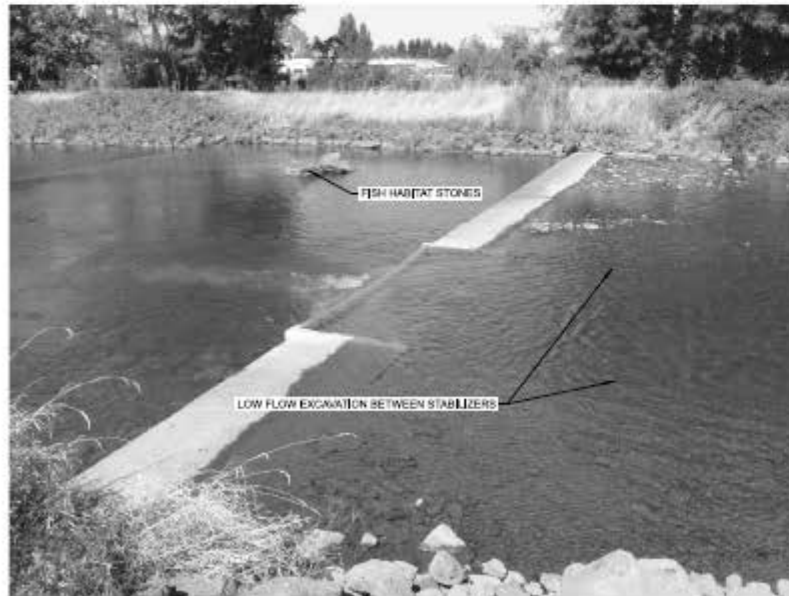
A1 PHOTO: EXISTING SINGLE NOTCH STRUCTURE WITH FLOW
