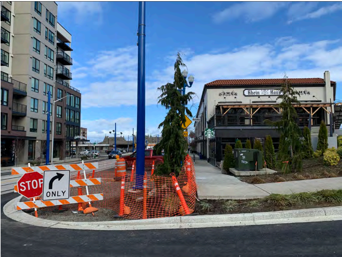
Photograph 12: View looking N along 1 st St.
