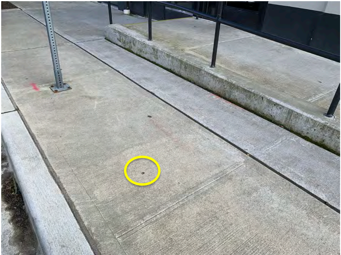
Photograph 1: Pavement Cap Marker "A". View is toward the northeast.
