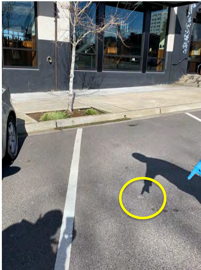
Photograph 3: Pavement Cap Marker "B". View is toward the north.
