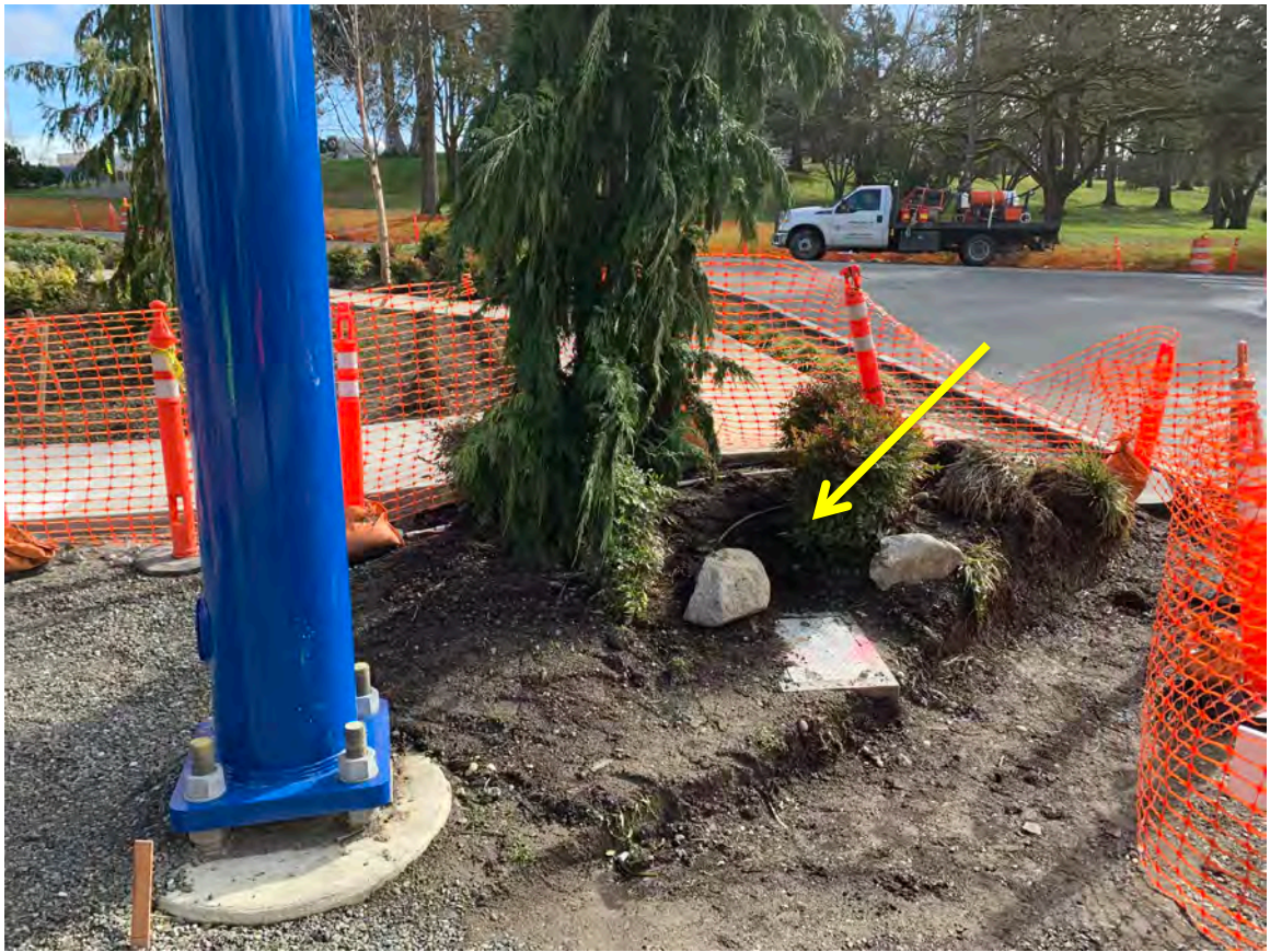
Photograph 7: Pavement Cap Marker "D". View is toward east.
