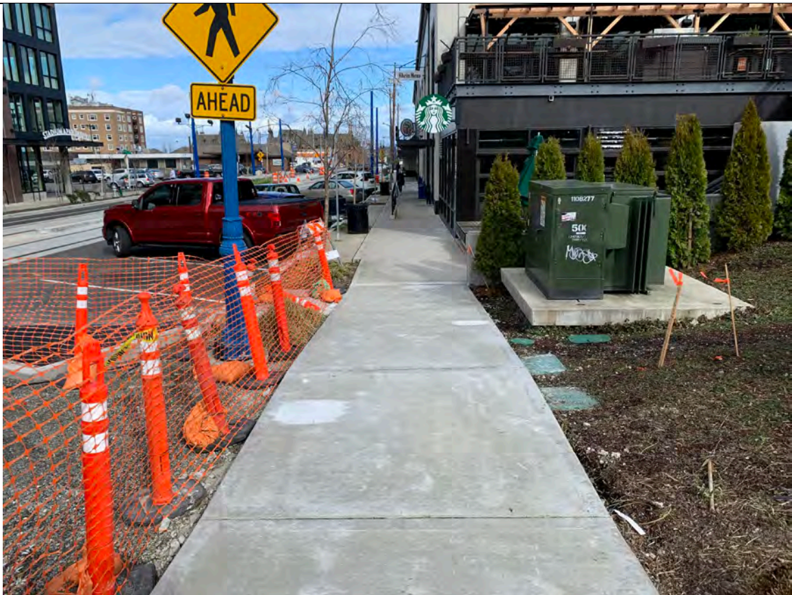
Photograph 10: View looking N along 1 st St.
