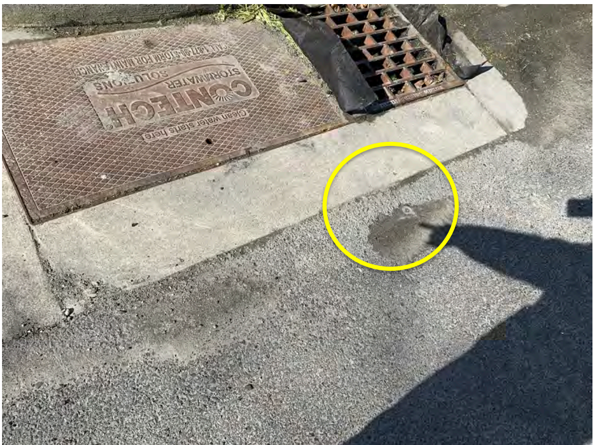
Photograph 6: Pavement Cap Marker "C"
