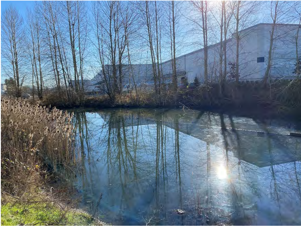
Picture 42 Stormwater pond at south end of 1514 Taylor Way Property
