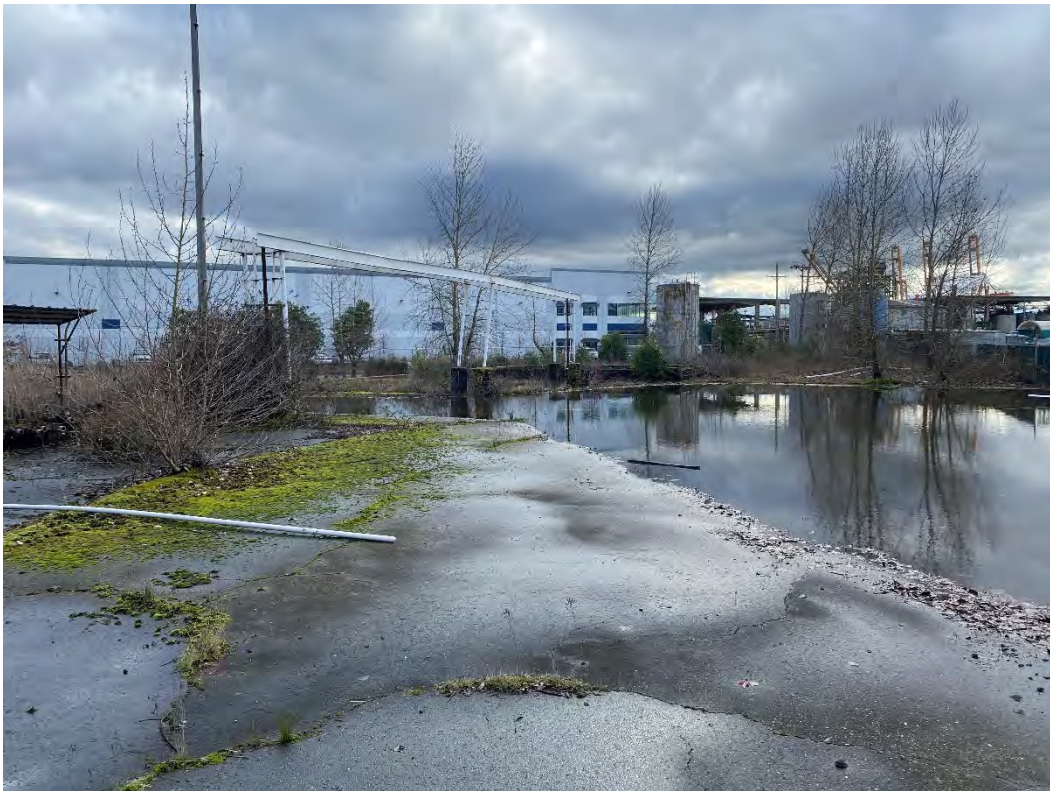
Picture 32 Ponded stormwater southwest of building 1, abandoned tanks in background on CleanCare Property
