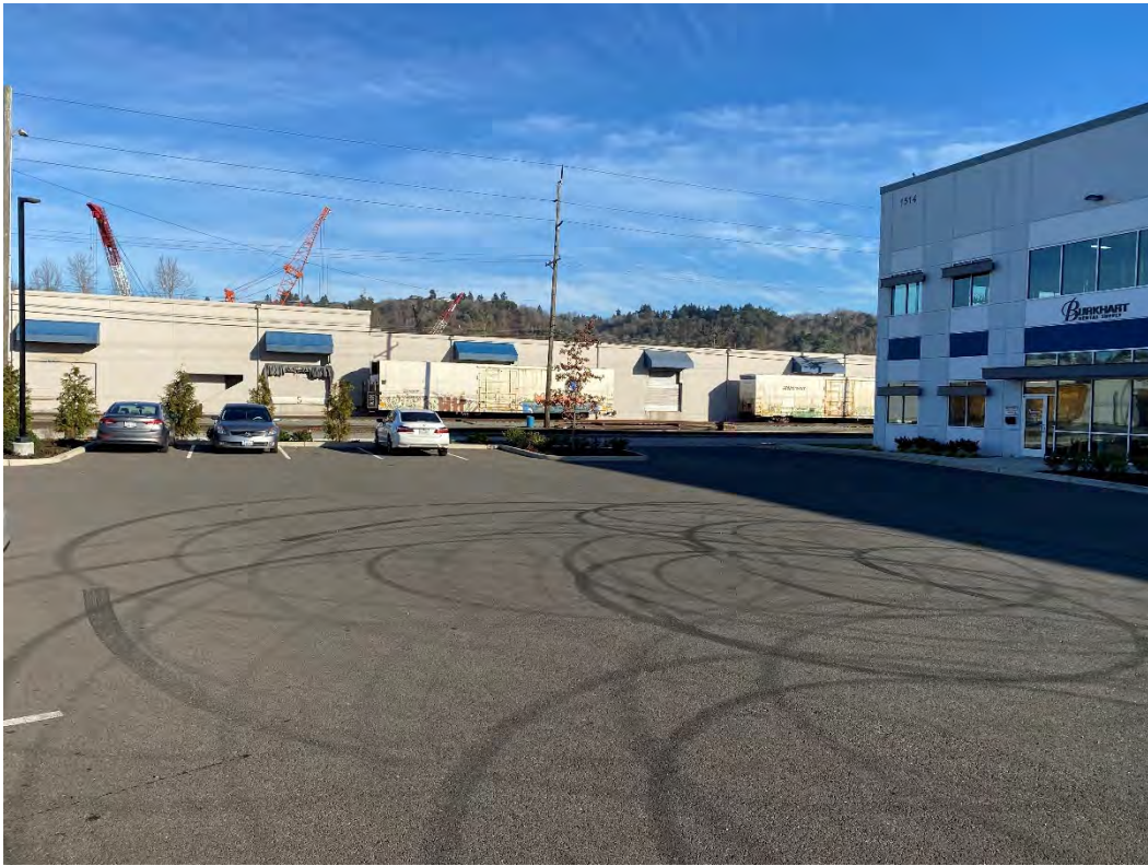
Picture 39 Building A (right) and parking area (left) looking north toward Taylor Way on 1514 Taylor Way Property
