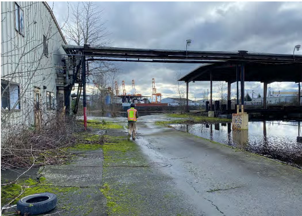
Picture 30 Ponded stormwater and former processing pipe rack overhead on CleanCare Property
