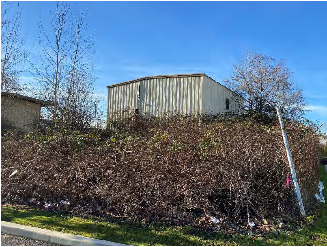
Picture 41 Looking west from 1514 Taylor Way Property toward CleanCare Property, building 3 in background, fencing missing
