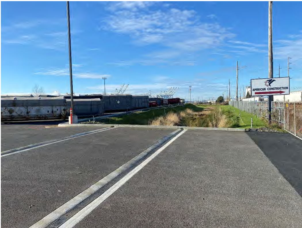
Picture 8 Western Taylor Way stormwater swale on Burlington Environmental Property
