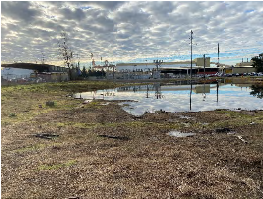
Picture 3 Ponding in southeast corner on 1205 Alexander Ave & 1300 Taylor Way Property
