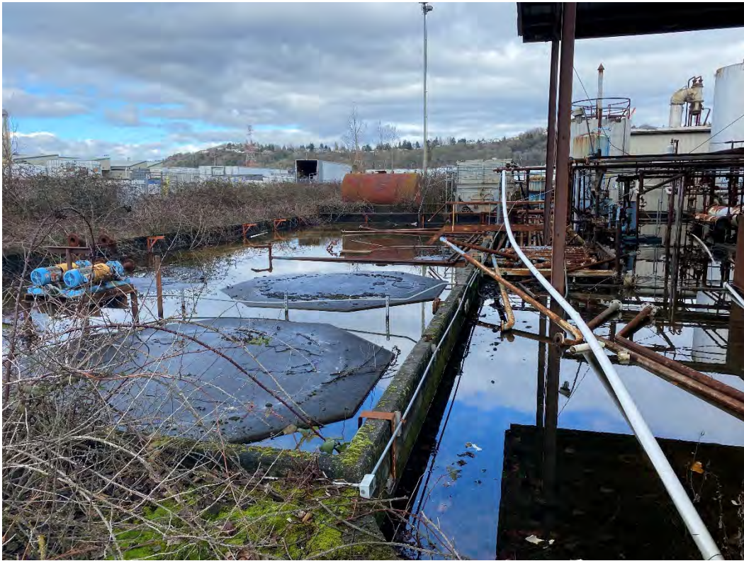
Picture 37 Former process area (containment and abandoned equipment) with ponded stormwater on CleanCare Property
