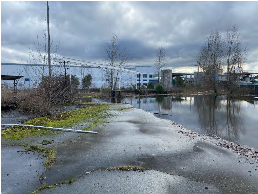
Picture 32 Ponded stormwater southwest of building 1, abandoned tanks in background on CleanCare Property
