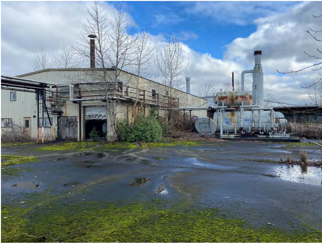
Picture 31 Former process equipment south of building 1 on CleanCare Property
