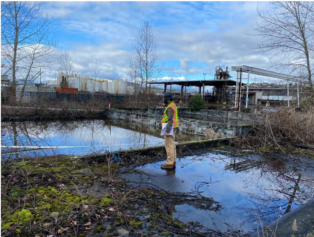
Picture 38 Containment area with stormwater southwest of building 5 on CleanCare Property
