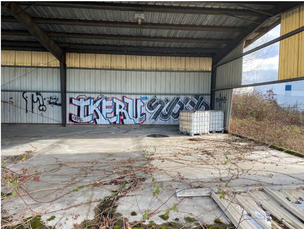
Picture 34 Abandoned totes in building 5 on CleanCare Property
