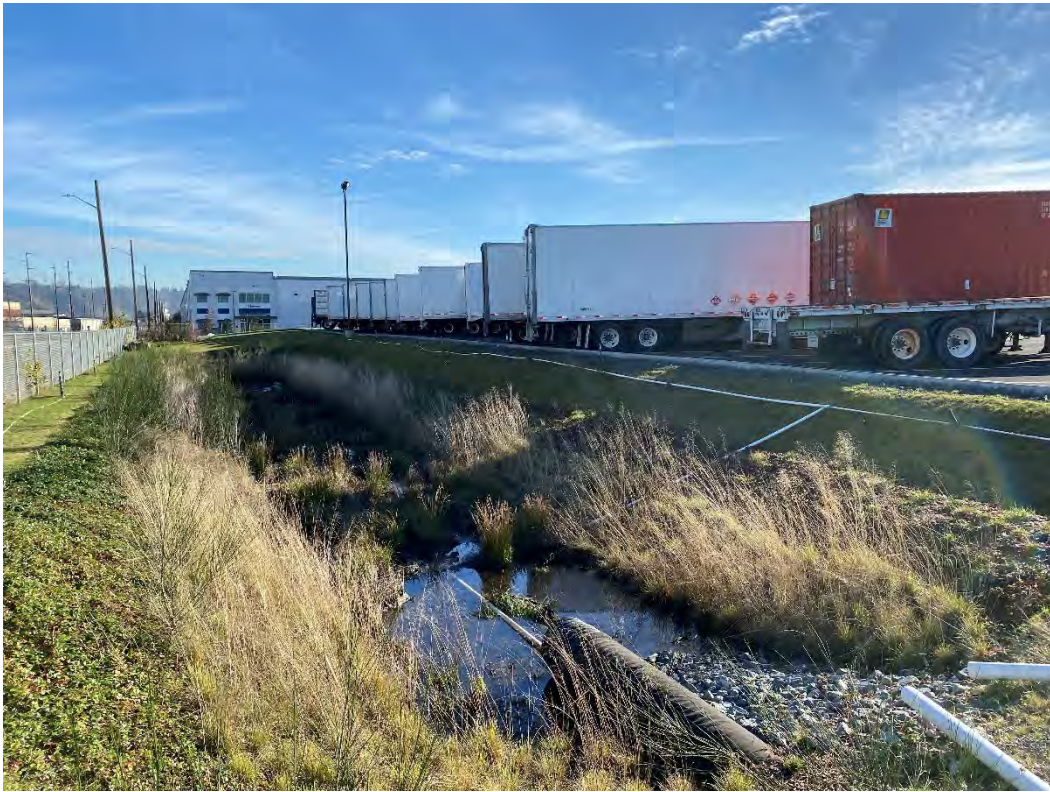
Picture 7 Eastern Taylor Way stormwater swale on Burlington Environmental Property
