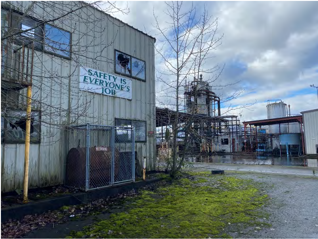
Picture 29 Heating oil tank inside fence on north side of building 1, abandoned process equipment in background with ponded stormwater on CleanCare Property
