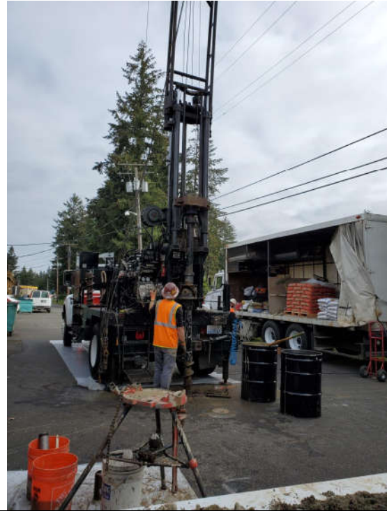
Photo #2: Installation of monitoring well MW-4 facing north.
