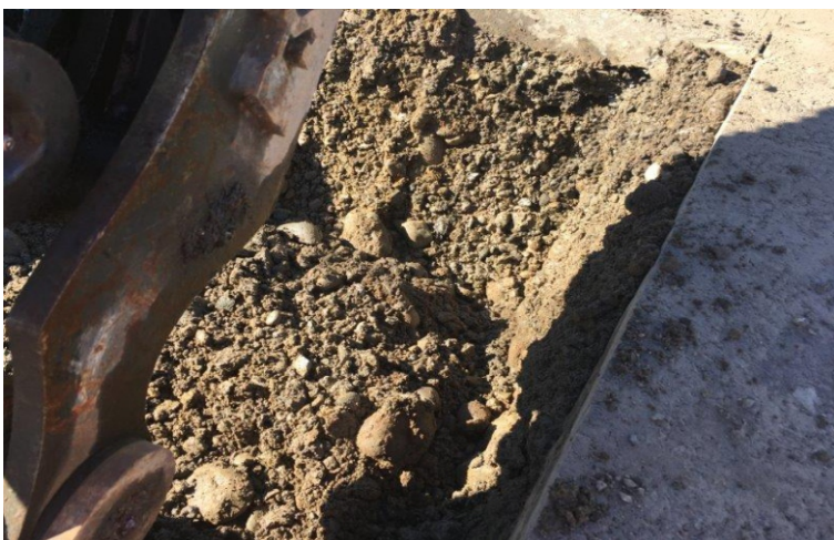
Photograph Five: Gasoline Contaminated Soil Test Pit 3
