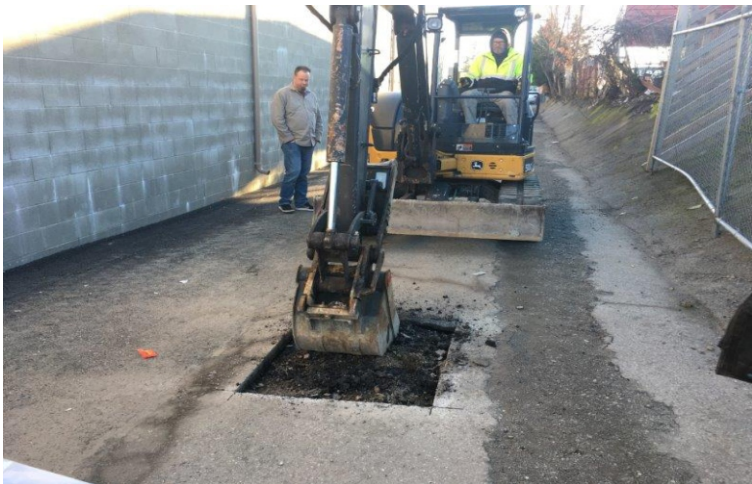
Photograph One: Breaking into Test Pit 1
