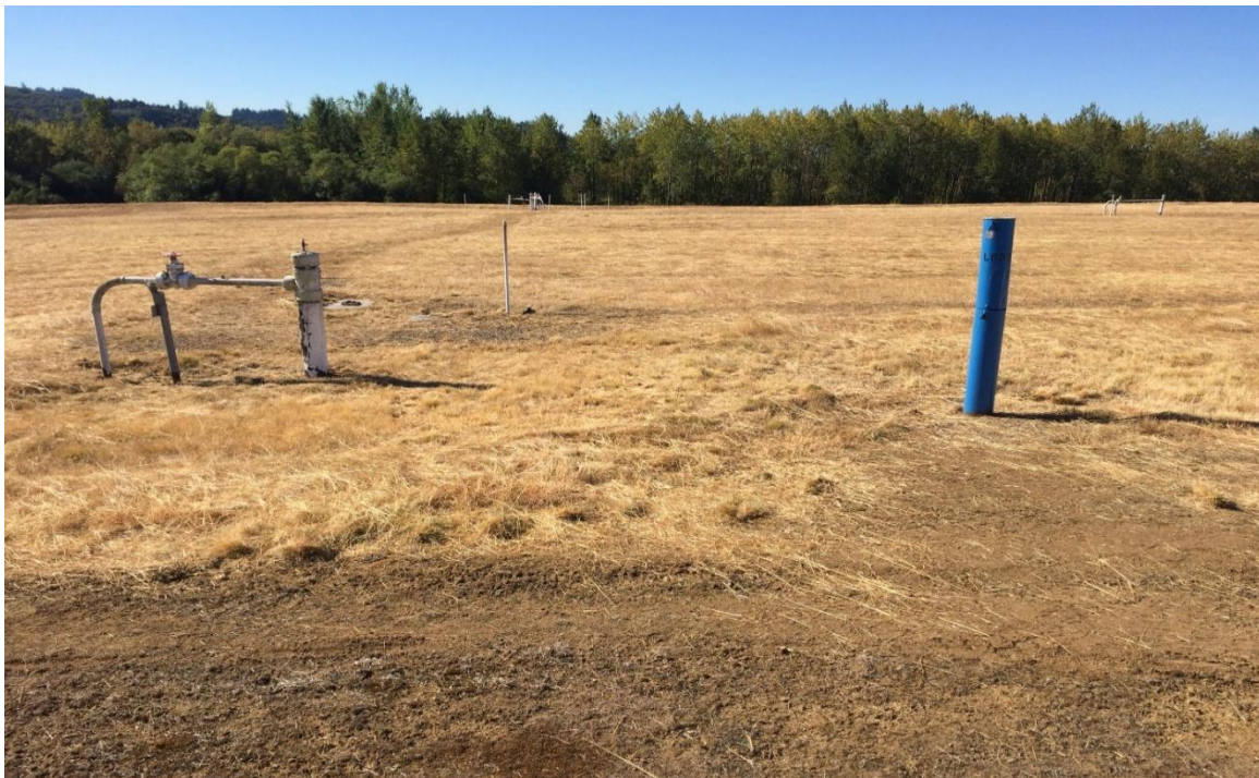
Photo 8: Landfill Gas Extraction Well, Groundwater Monitoring Well and Landfill Cap - From the Southwest
