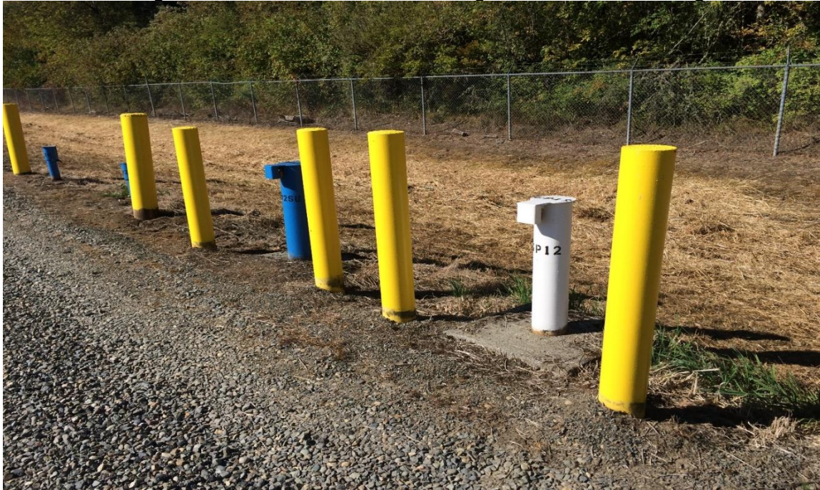
Photo 5: Downgradient Groundwater Monitoring Wells – Western Edge of the Landfill
