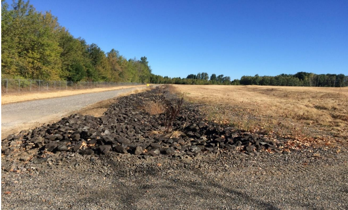
Photo 3: Western Edge of Landfill Cap (Drainage System) - From the South
