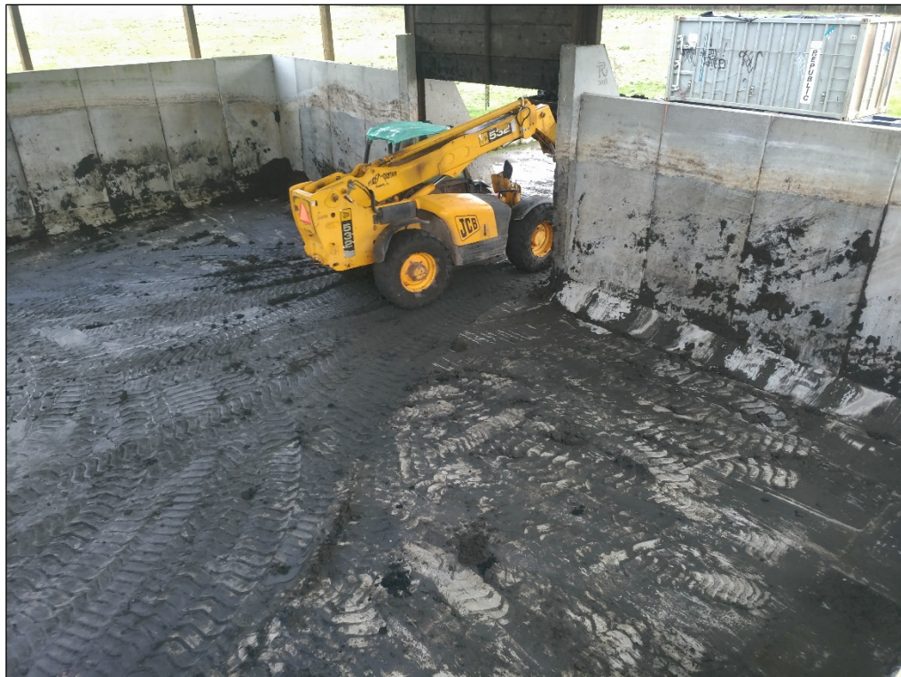
4. Removing mixed material from Big Hanaford (01/18/2021).
