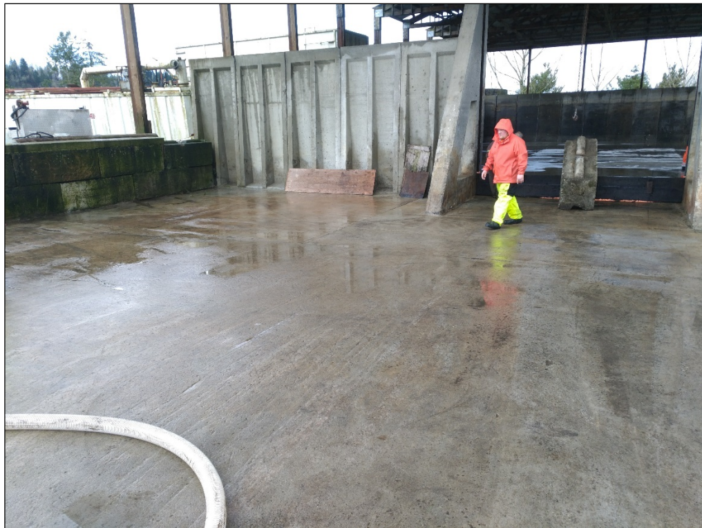
8. Mixed-material removal and decontamination complete (02/5/2021).
