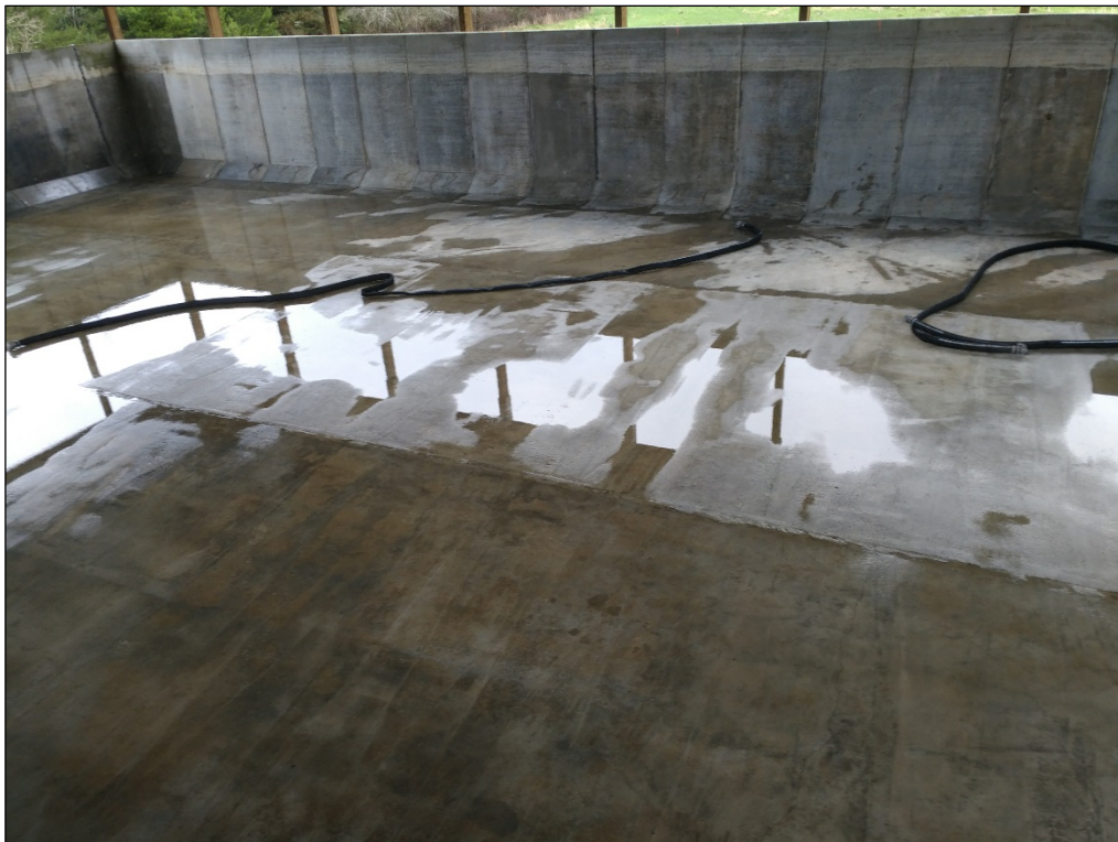
6. Mixed-material removal and decontamination complete (02/05/2021).
