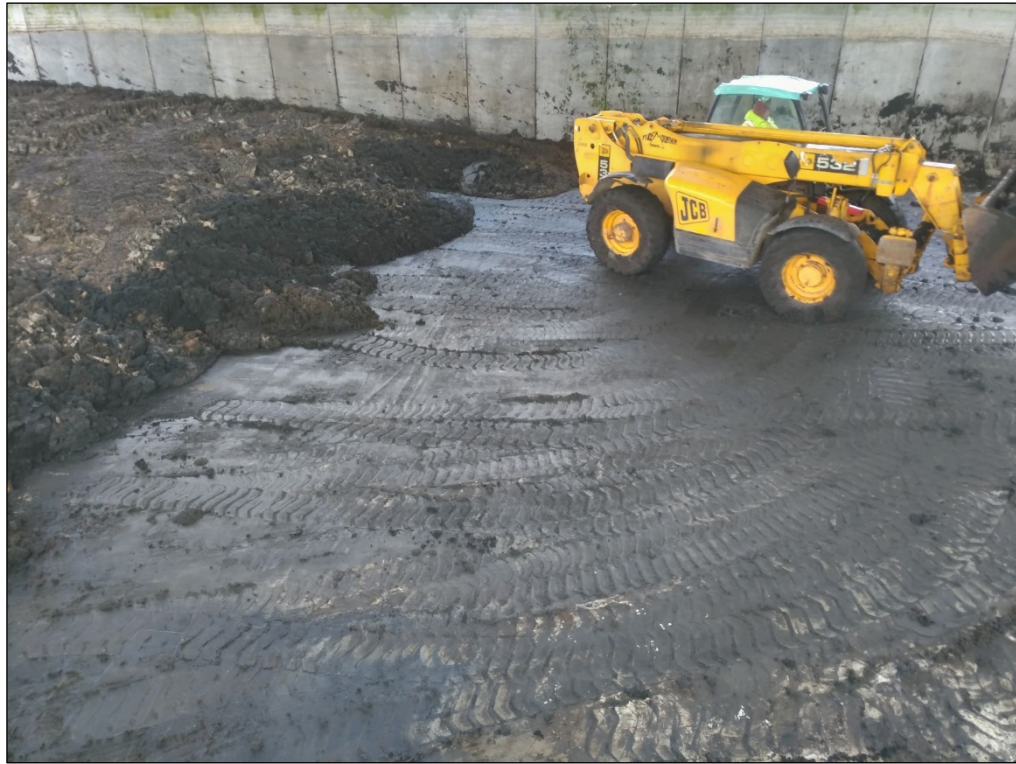
3. Storage unit being emptied (01/18/2021).
