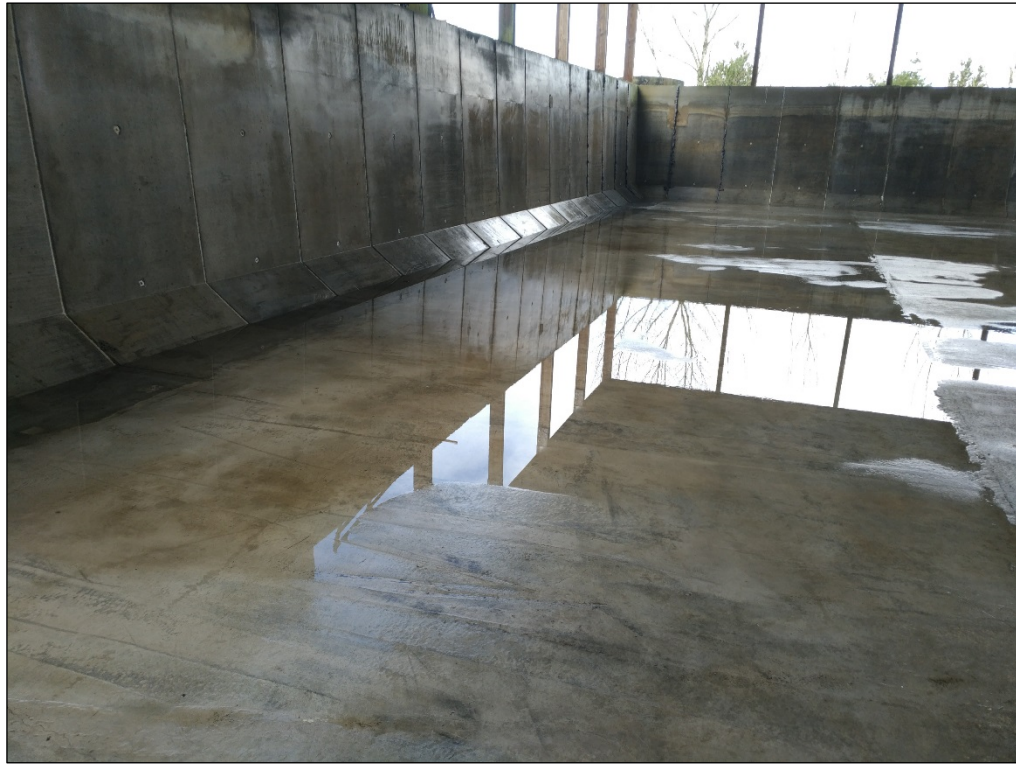
7. Mixed-material removal and decontamination complete (02/5/2021).
