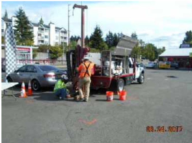
Photograph 7. Installation of soil boring SB-5 within the south-central portion of the Site, associated with the former fueling station UST area.
