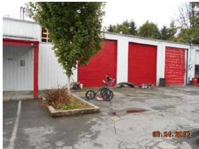
Photograph 2. View of western portion of former site building (automotive repair) prior to demolition, looking south from Pacific Highway South.
