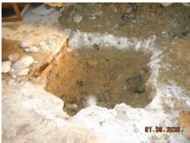
Photograph 11. View of removal of former sump observed within western most automotive bay (Bay 1).
