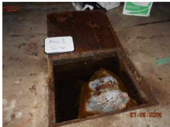
Photograph 4. A former sump as observed within western most automotive bay (Bay 1).
