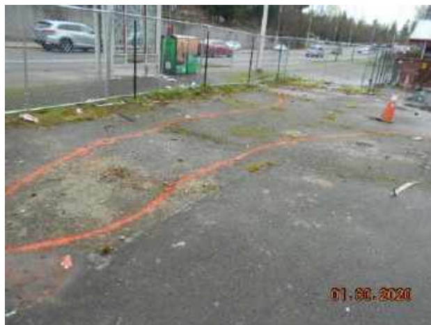
Photograph 12. View of "Plume E" prior to excavation along the eastern Site limits as identified using GPS coordinates from previously completed soil borings.
