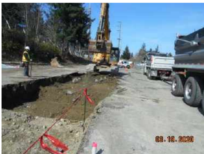
Photograph 17. Loading of hydrocarbon-impacted soil from “Area B2”.
