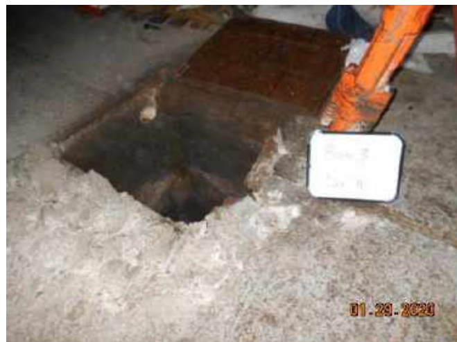
Photograph 6. A former sump as observed within center automotive bay (Bay 3) prior to removal.
