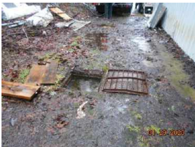
Photograph 5. View of former exterior sump located along western limits of former site building.
