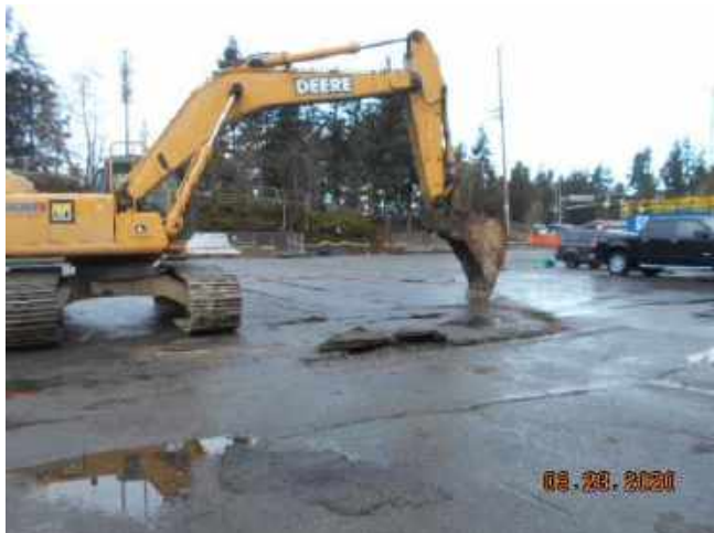
Photograph 13. Impervious surface (asphalt) removal prior to excavation of “Area C4”, looking northwest.
