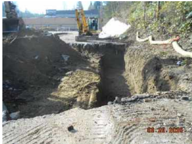
Photograph 14. Excavation of “Area A5” and “Area A2” for removal of arsenic-impacted soil at location of former commercial greenhouse.
