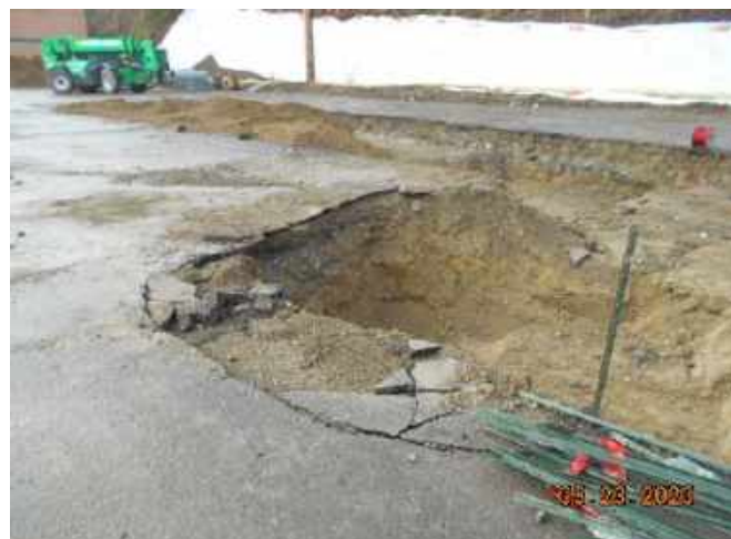
Photograph 16. View of “Area B1” (looking southwest) following over-excavation.
