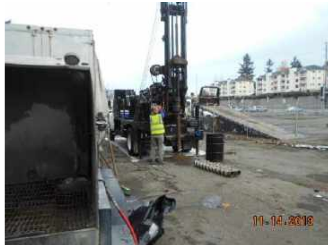
Photograph 8. Installation of soil boring SB-15B, down-gradient of the reported former commercial greenhouse that operated within the northwestern limits of the Site.
