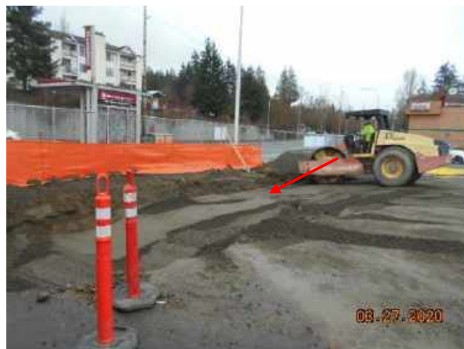
Photograph 18. View of backfilling and compaction of “Area E” following completion of excavation.
