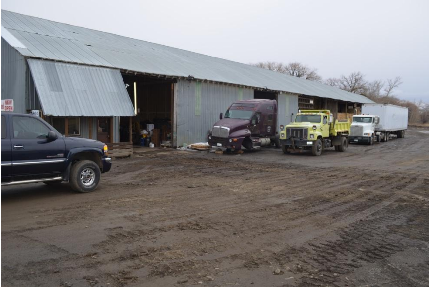
Initial trench excavation was completed between the scale house/residence and the adjunct shop building.
