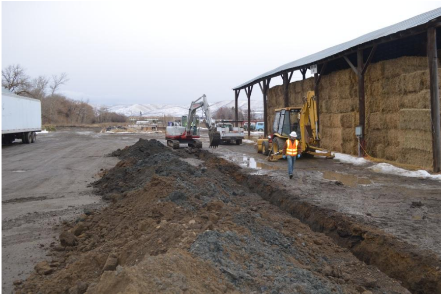
Surface staining was observed to include approximately 1-foot of stained surface soils with underlying clean soil
