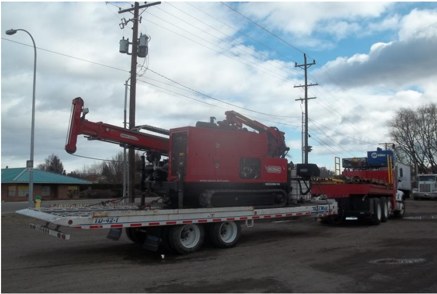
Arrival of the direct-push hydraulic boring machine at the site.
