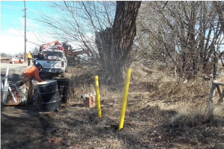
Monitoring Well 07, located immediately adjacent to Wilson Creek, the adjacent surface water and primary influence of site groundwater.
