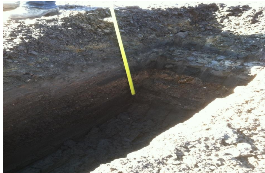
Surface staining was present to a depth approximately 1-foot of with underlying clean soil on the east side of the shop building.
