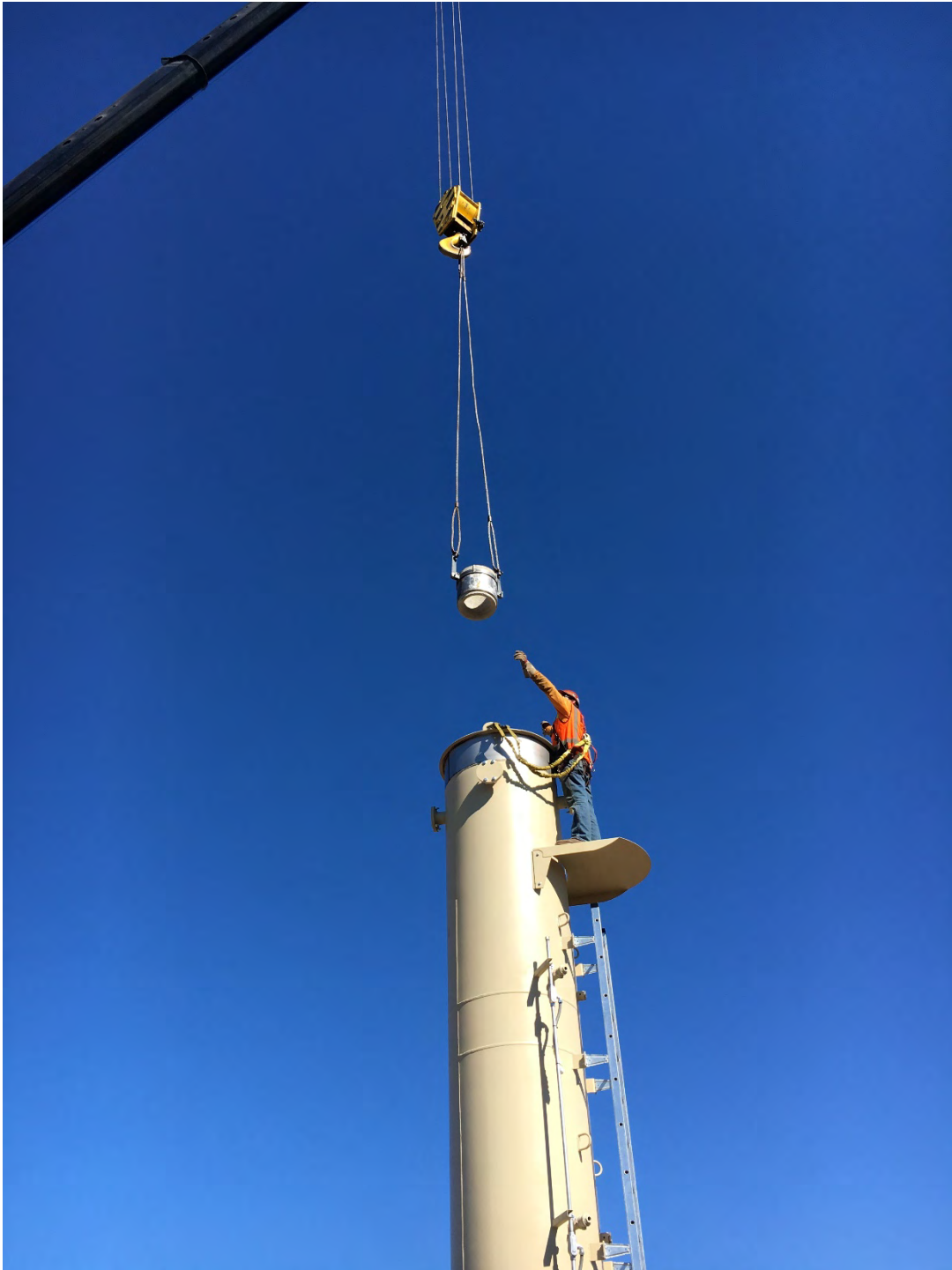
September 28, 2020 – placement of burner pot
