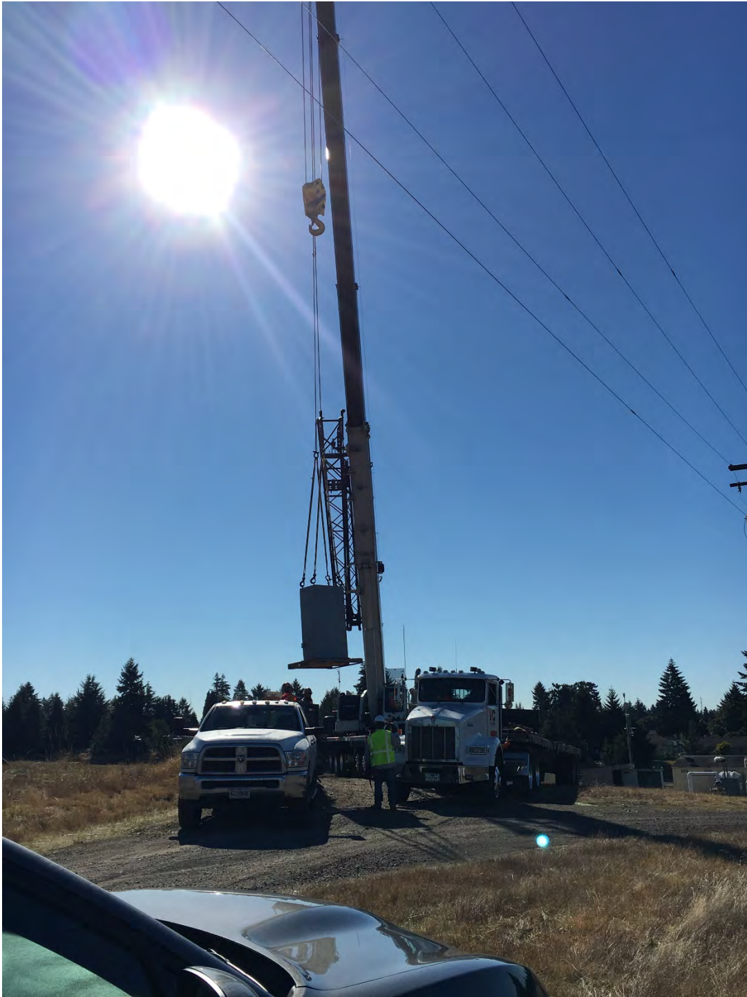
September 28, 2020 – Lift of control panel for placement inside flare compound
