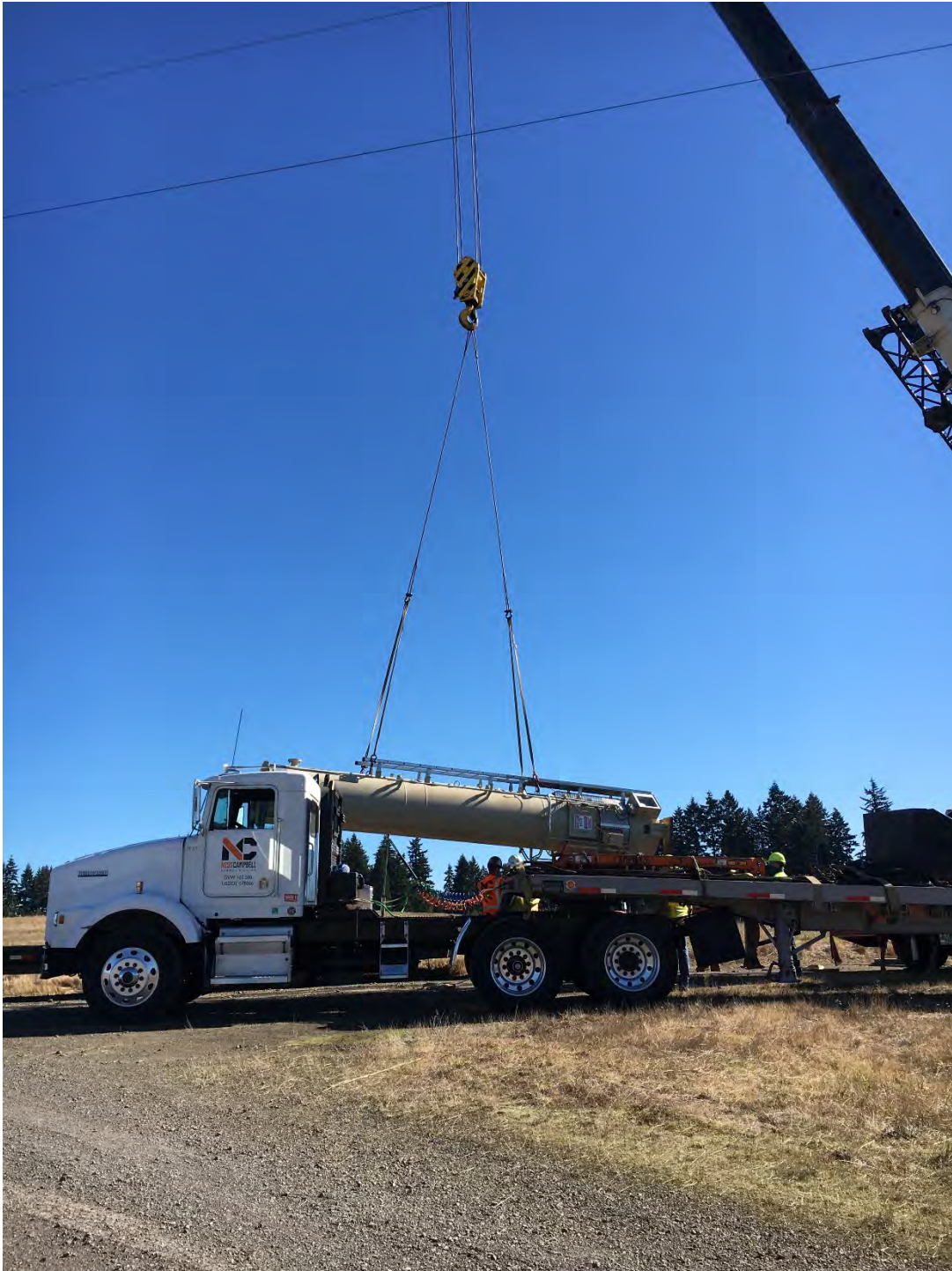
September 28, 2020 – lifting new flare off of truck
