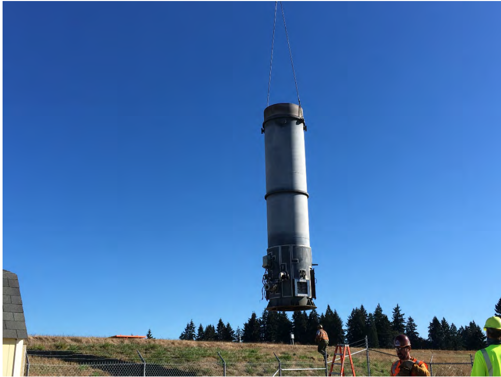
September 28, 2020 – lifting flare off of flare pad
