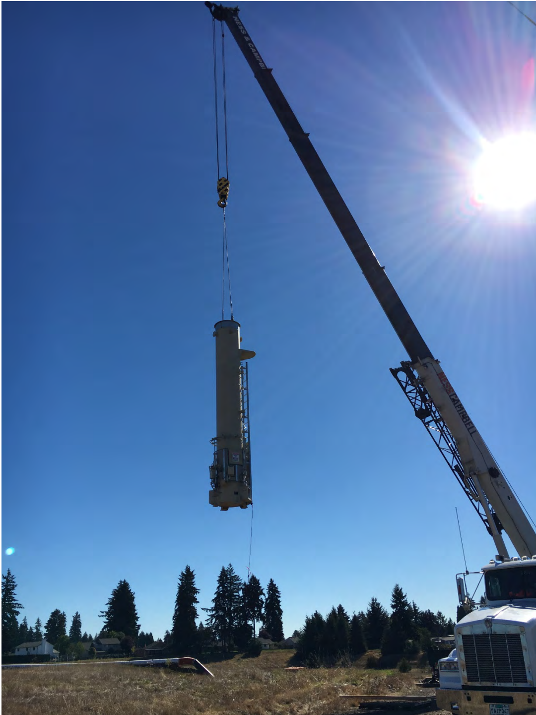
September 28, 2020 – lifting flare to flare pad
