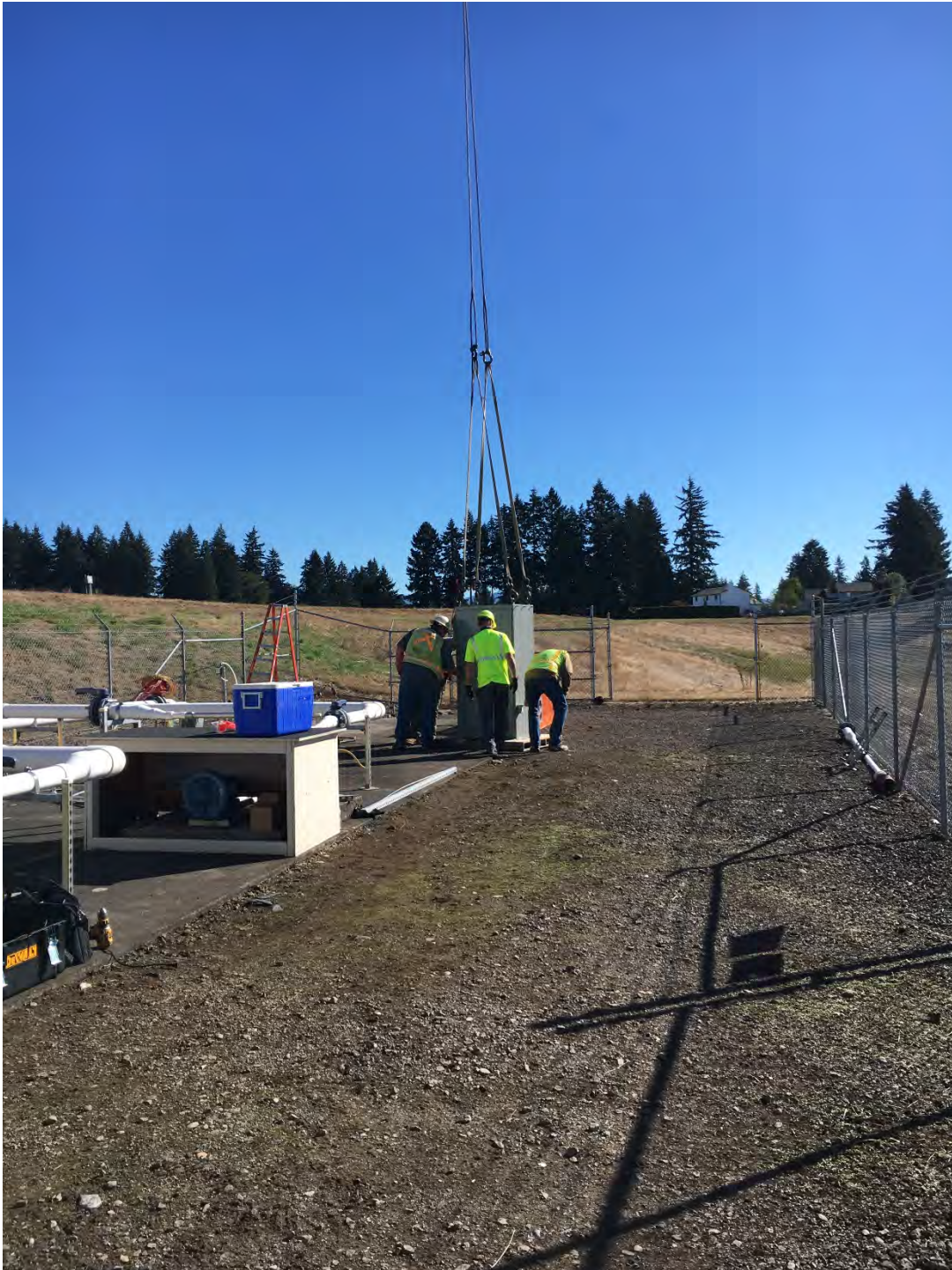
September 28, 2020 – placement of flare control panel inside flare compound
