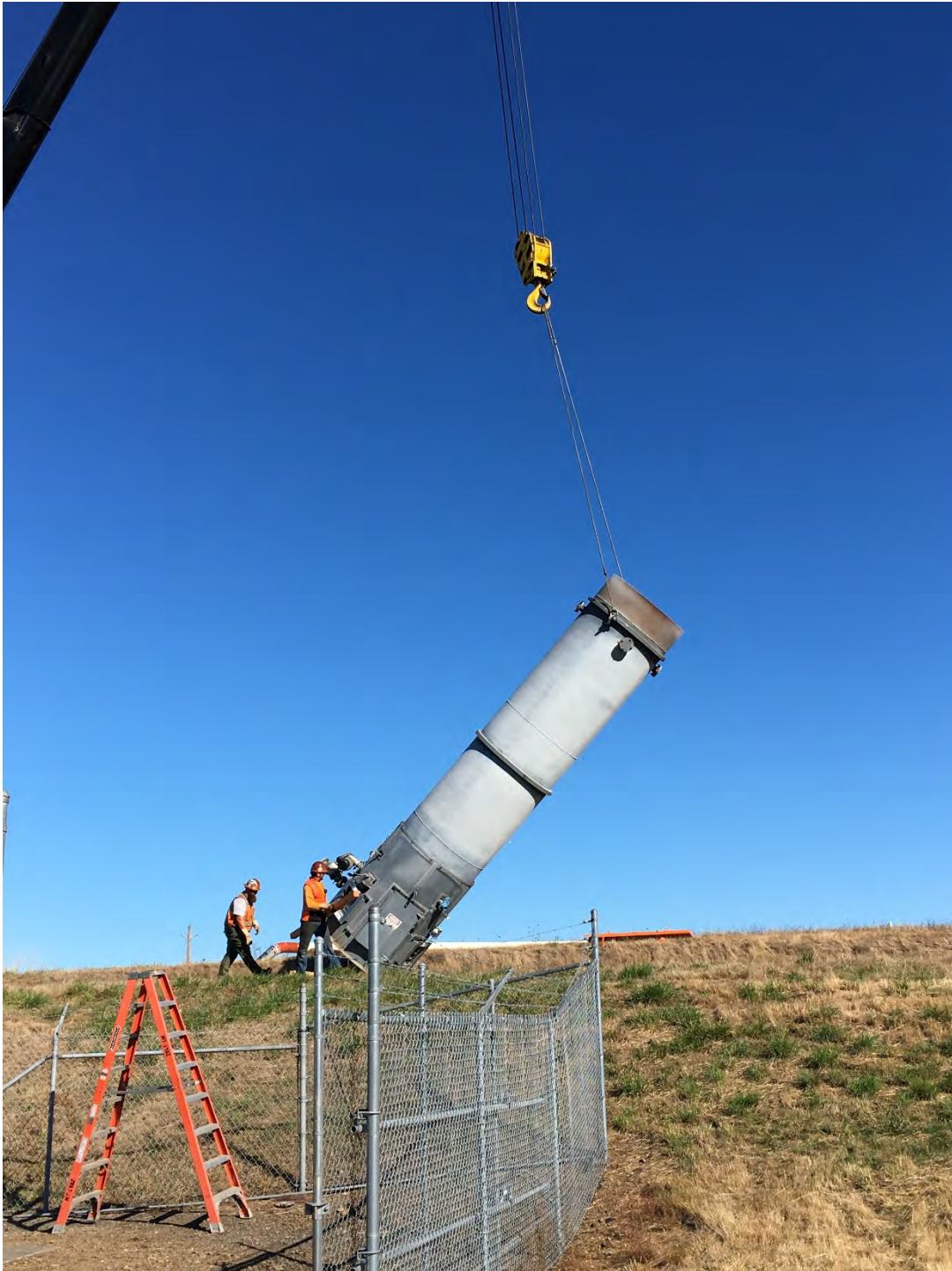
September 28, 2020 – setting flare down prior to placement on truck
