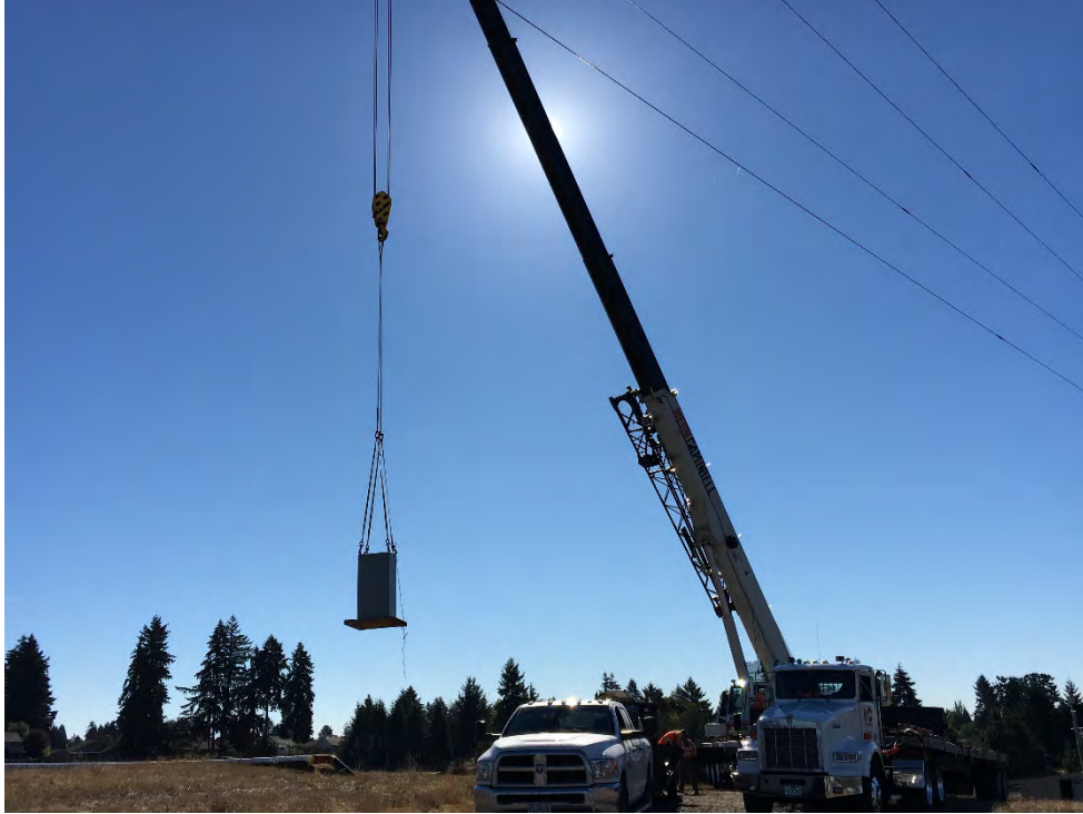
September 28, 2020 – Lift of control panel for placement inside flare compound
