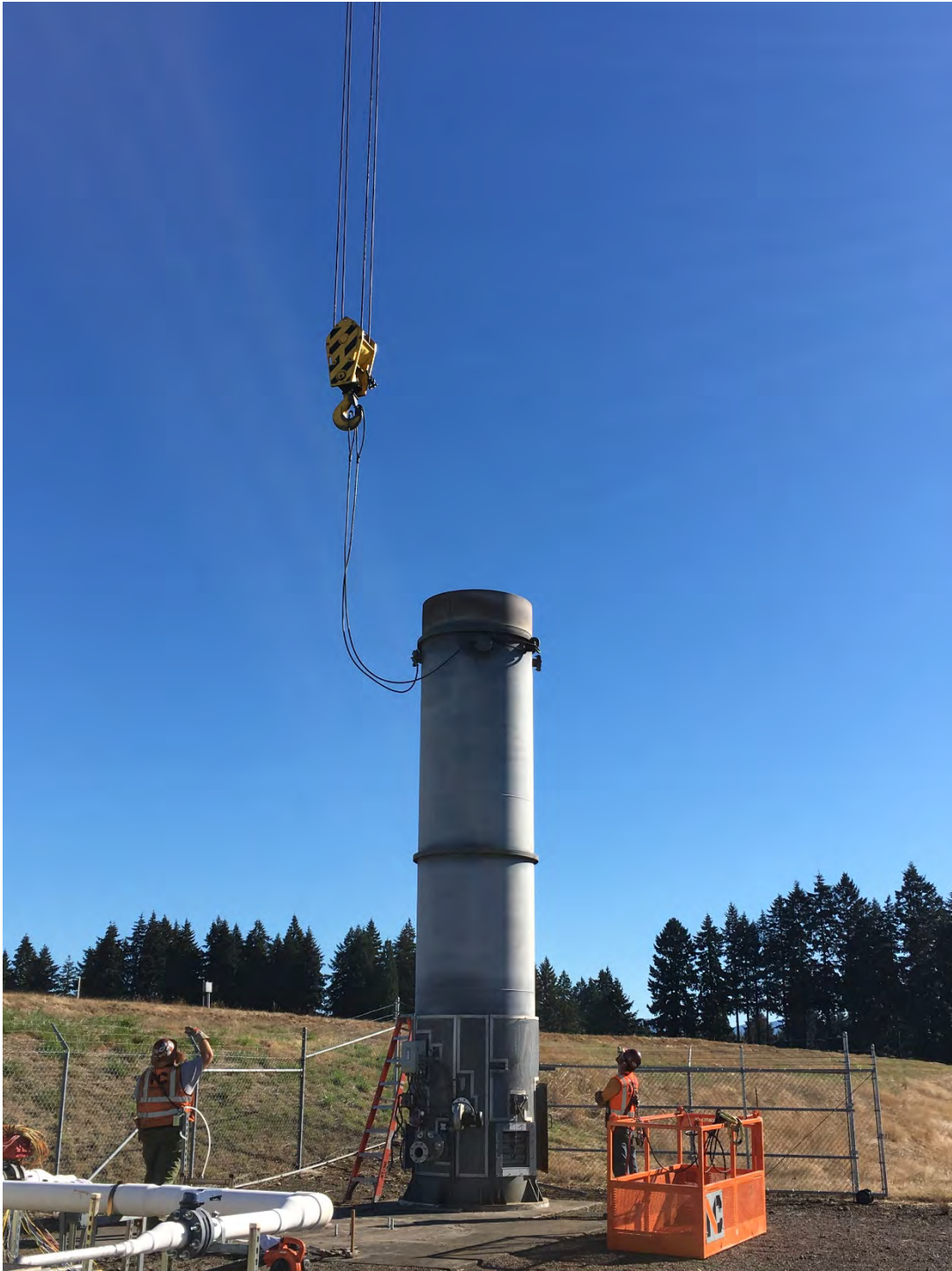
September 28, 2020 – Getting ready to remove old flare
