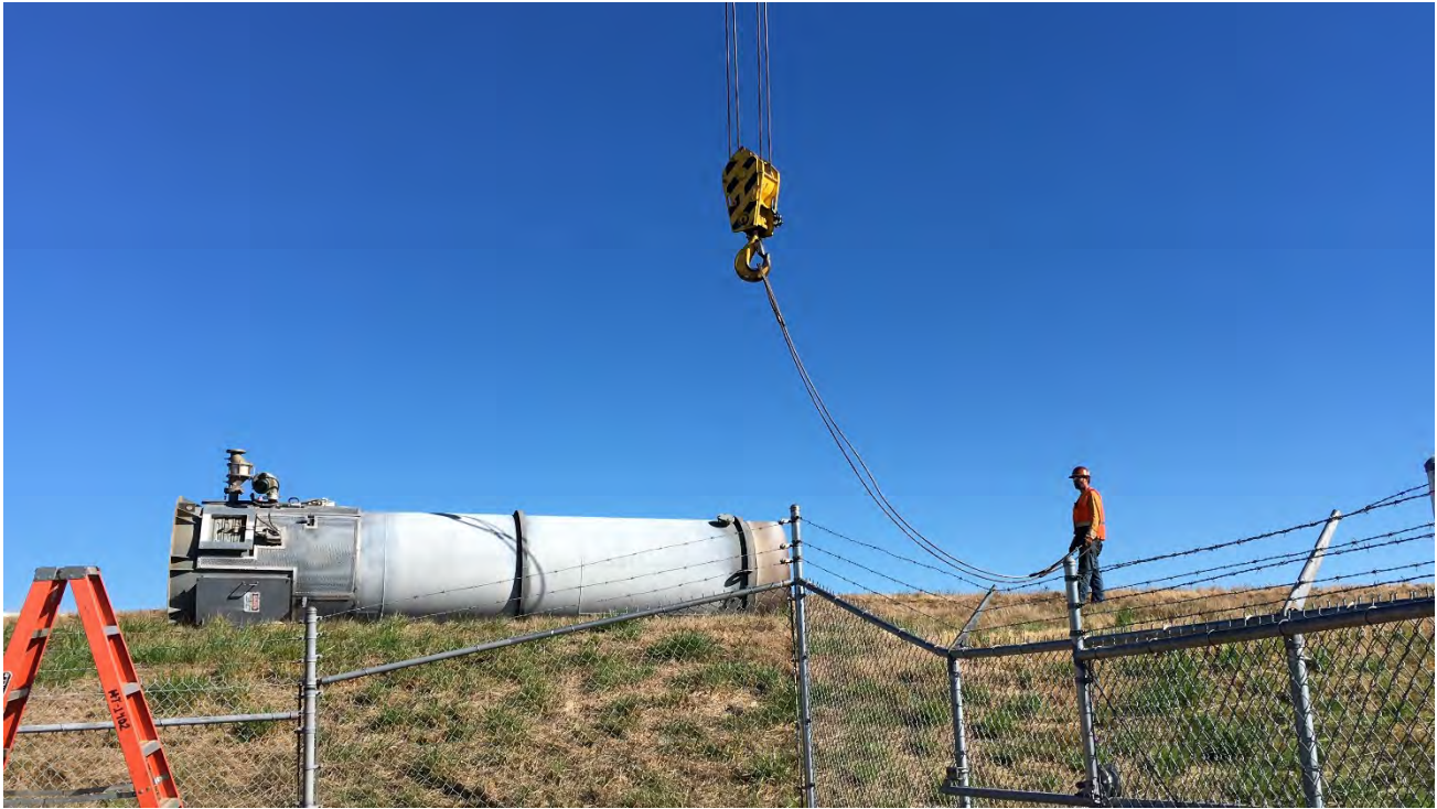
September 28, 2020 – setting flare on its side prior to placement on truck
