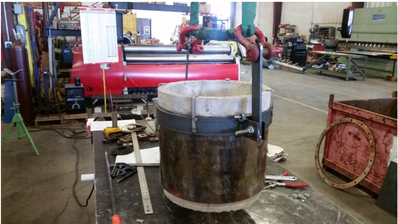
August 25, 2020 – Flare burner pot at Perennial manufacturing facility
