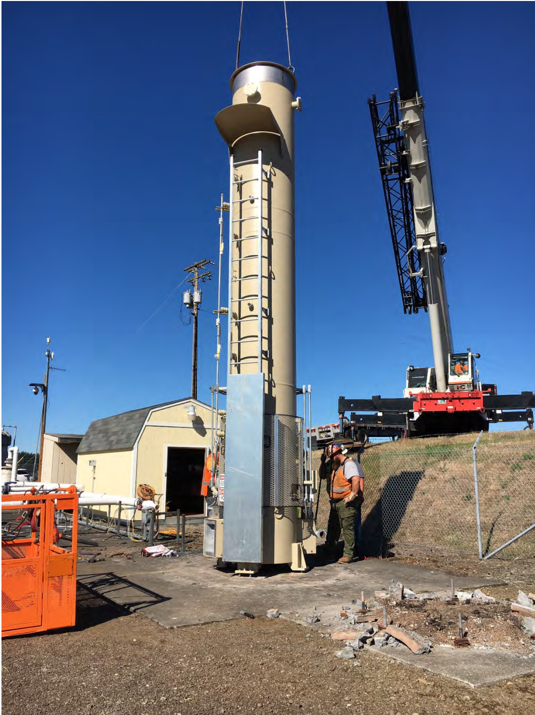
September 28, 2020 – flare alignment adjustments on flare pad
