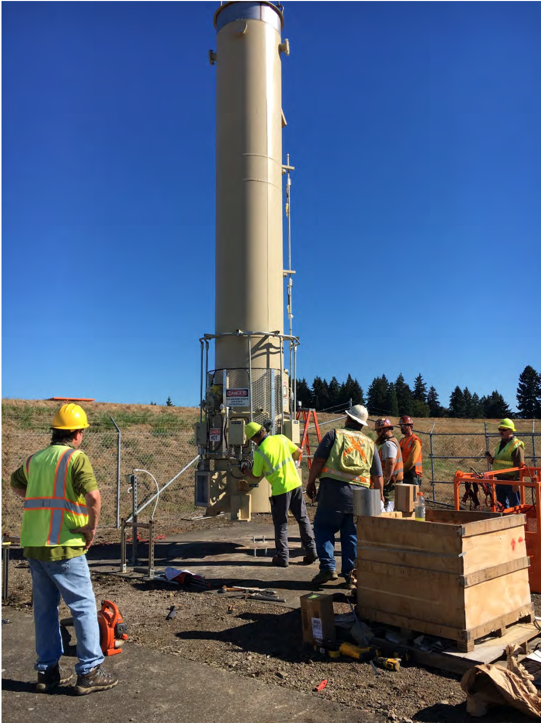
September 28, 2020 – aligning flare on flare pad
