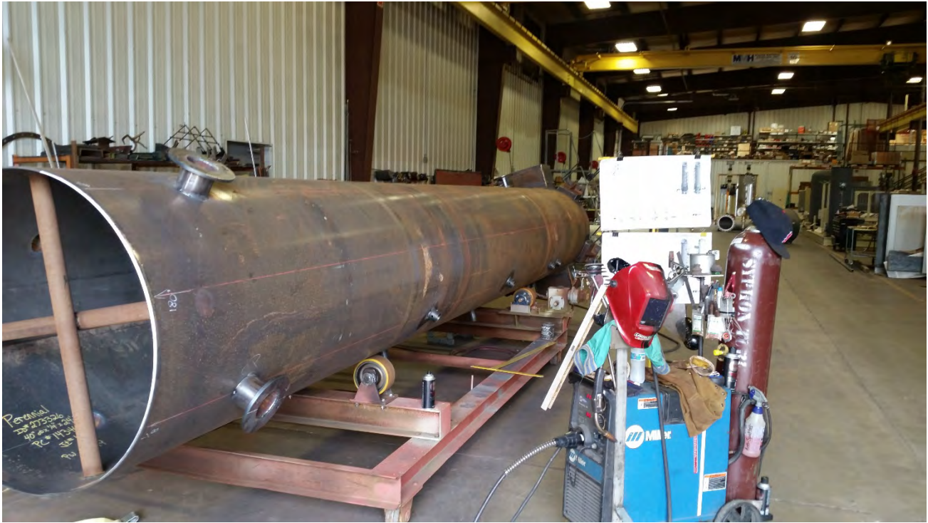
August 14, 2020 - Flare shell during construction at Perennial manufacturing facility
