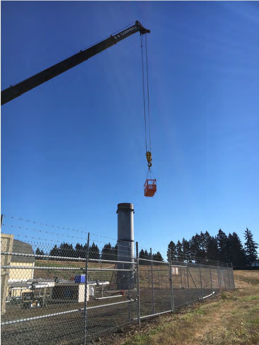
September 28, 2020 – Ness Campbell crane setup
