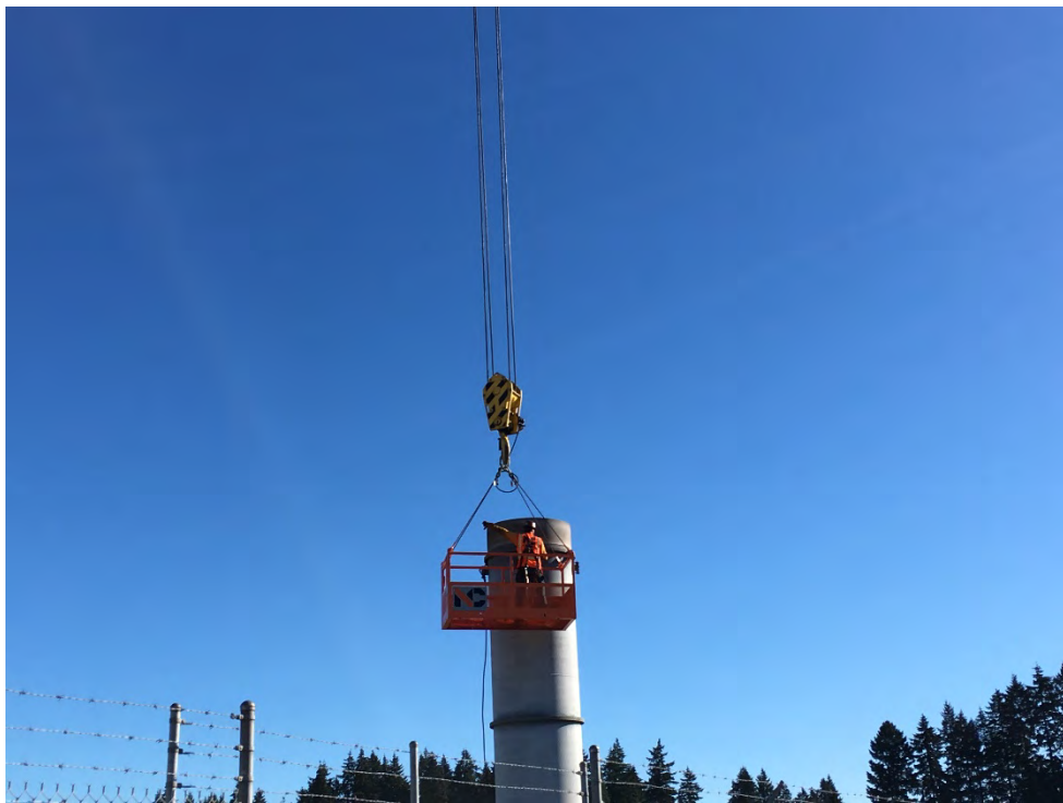
September 28, 2020 – Preparation of old flare for removal by attaching lift cords
