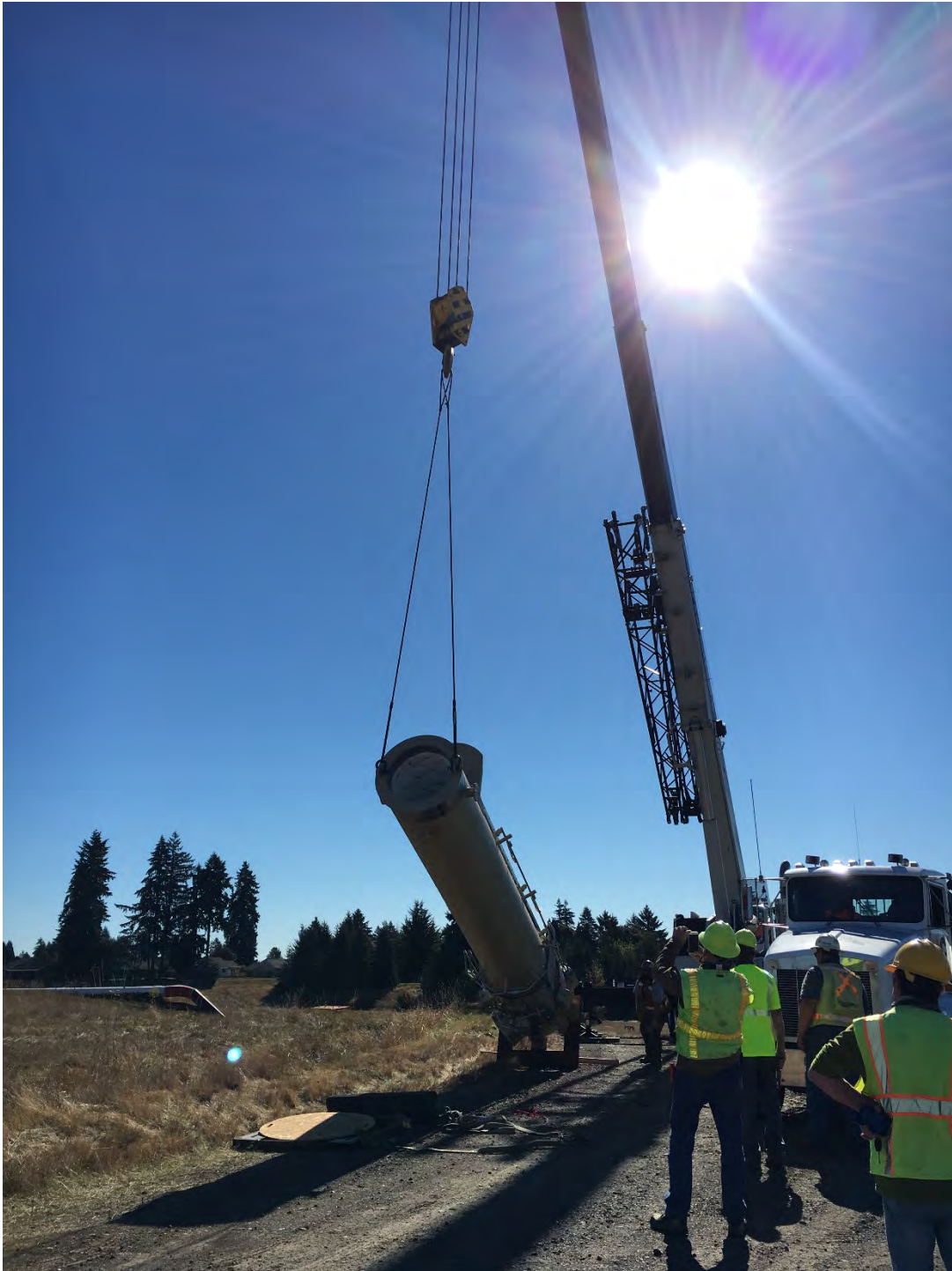
September 28, 2020 – lifting flare to flare pad
