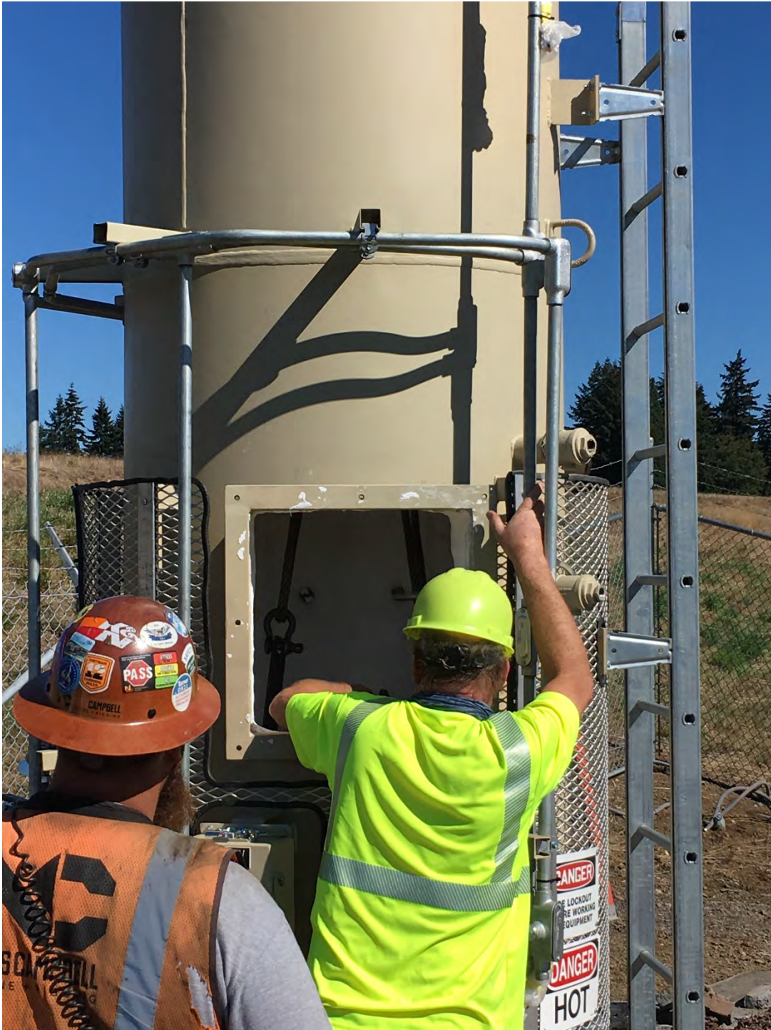
September 28, 2020 – alignment of burner pot inside flare
