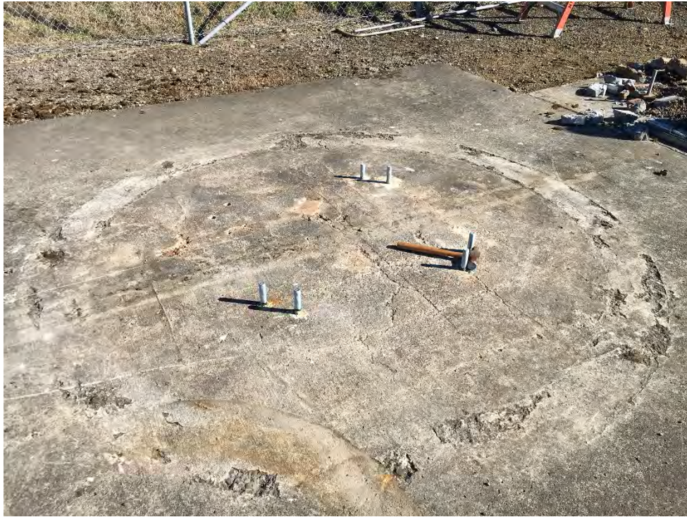
September 28, 2020 - New flare pad with 3 of 4 sets of pre-drilled bolt holes
