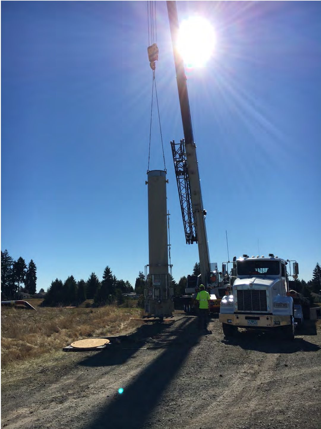
September 28, 2020 – lifting flare to flare pad
