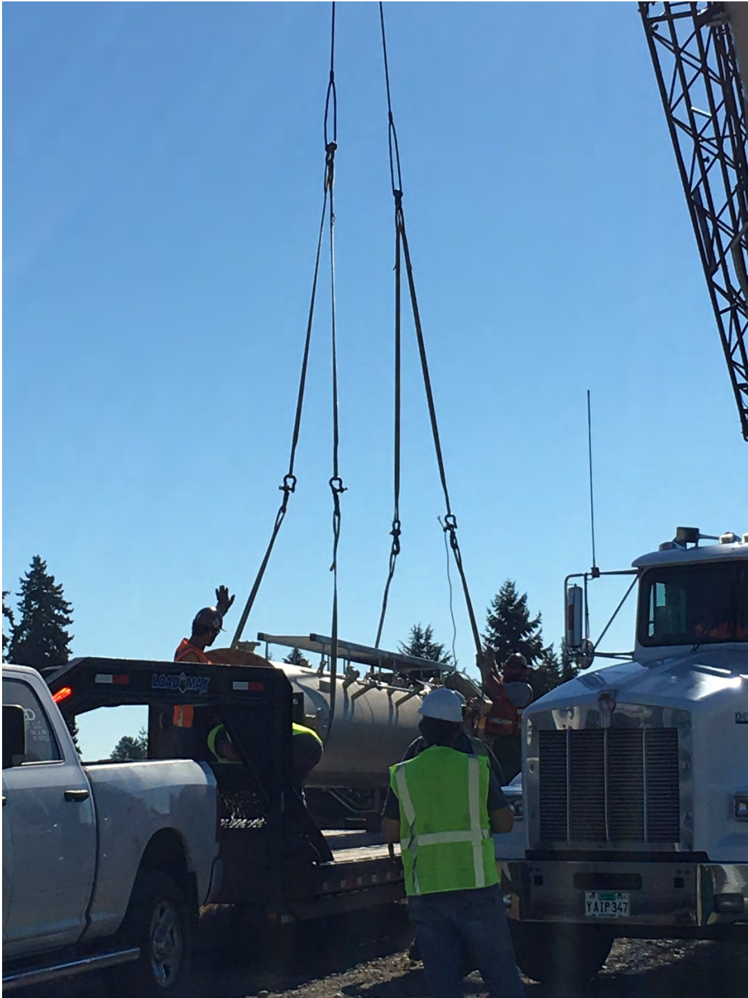
September 28, 2020 – Lifting new flare off of truck
