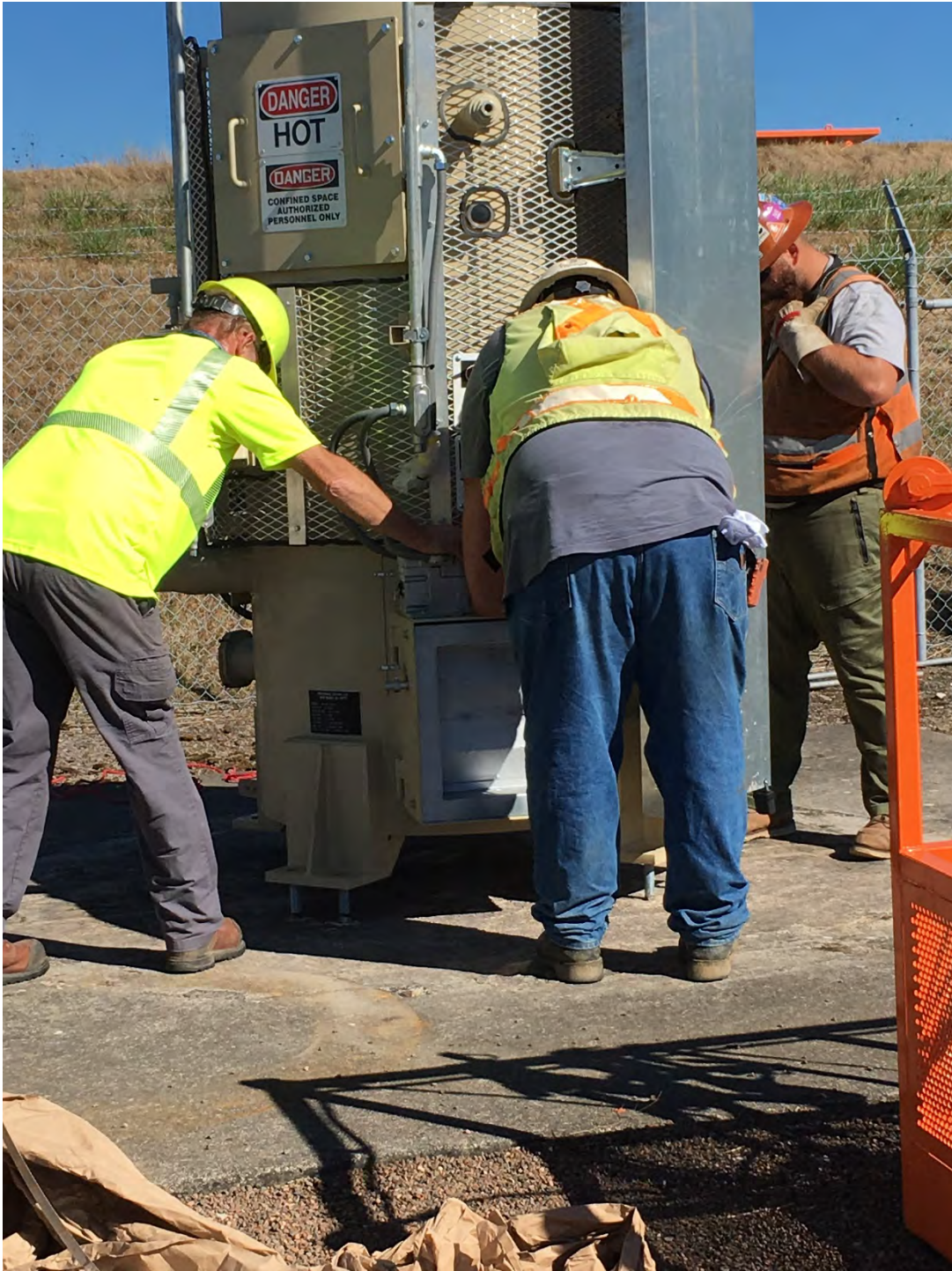
September 28, 2020 – aligning flare over bolts on flare pad
