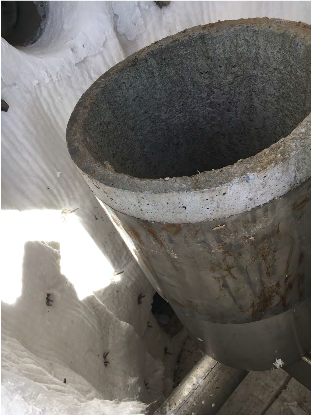
September 28, 2020 – flare burner pot alignment
