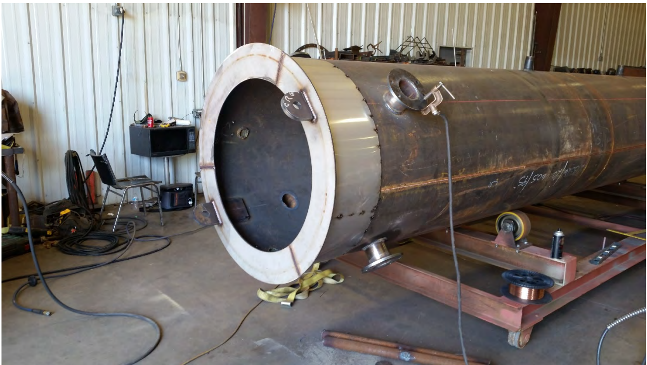
August 17, 2020 - Top of flare with lifting lugs and top ring in place at Perennial manufacturing facility
