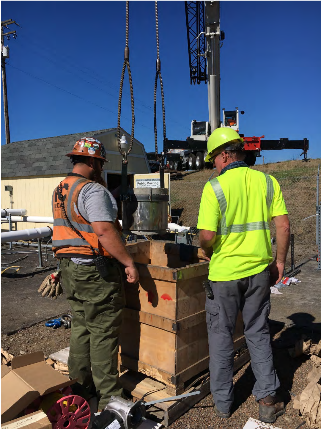
September 28, 2020 – preparing to place burner pot
