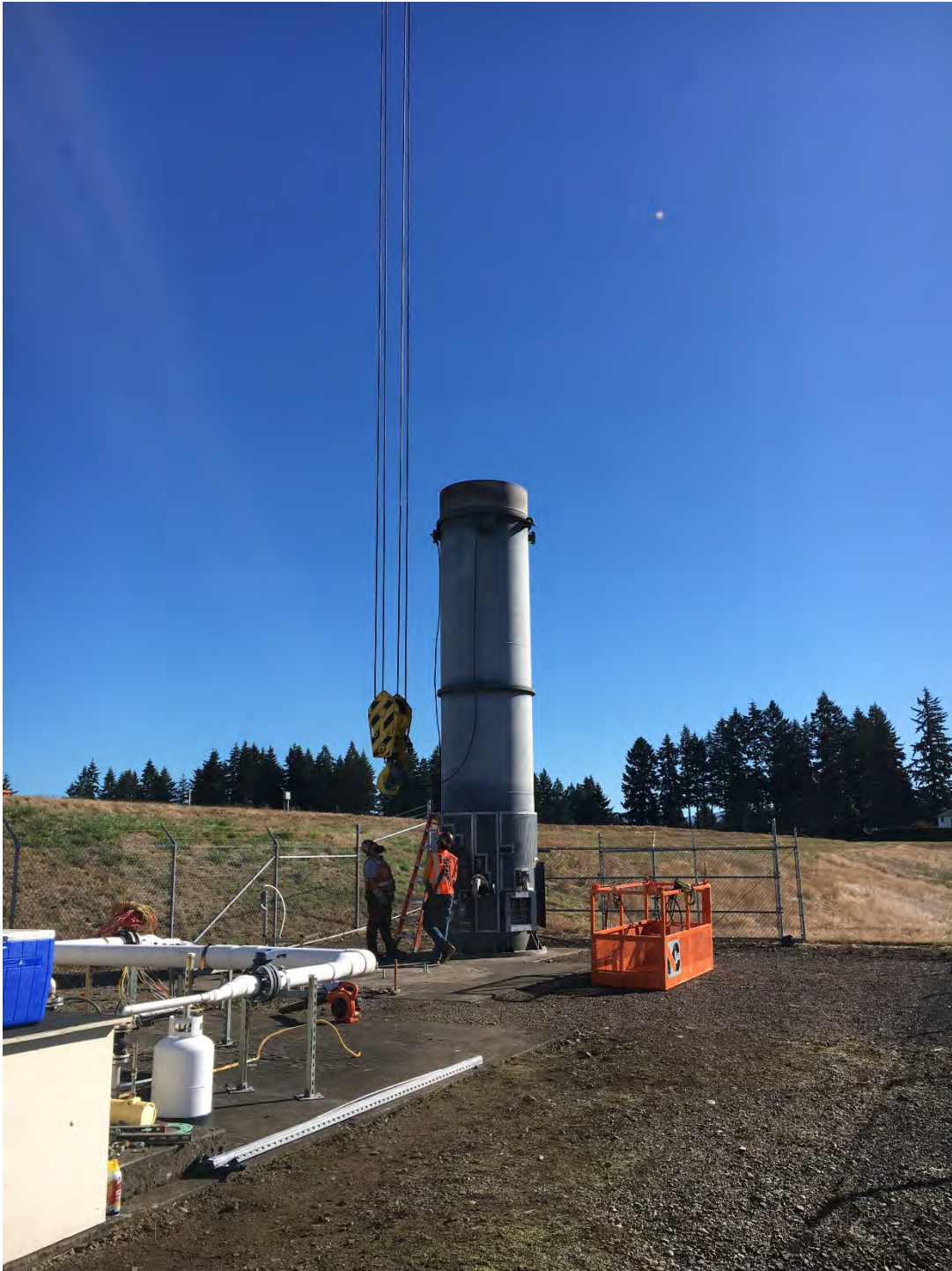
September 28, 2020 – Preparation of old flare for removal by attaching lift cords
