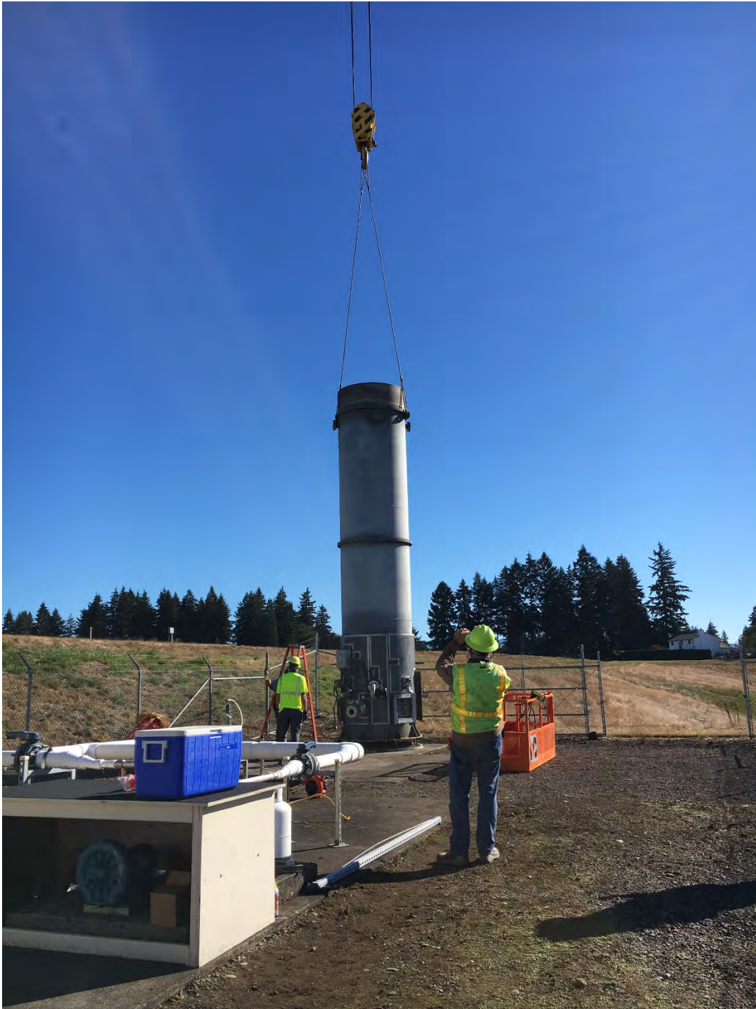
September 28, 2020 – Lifting old flare from existing flare pad
