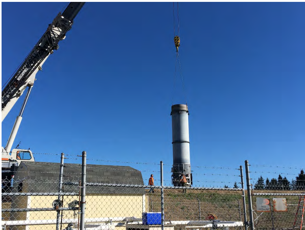
September 28, 2020 – lifting flare off of flare pad
