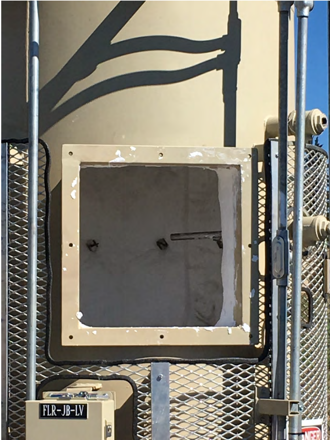
September 28, 2020 - inside side access hatch
