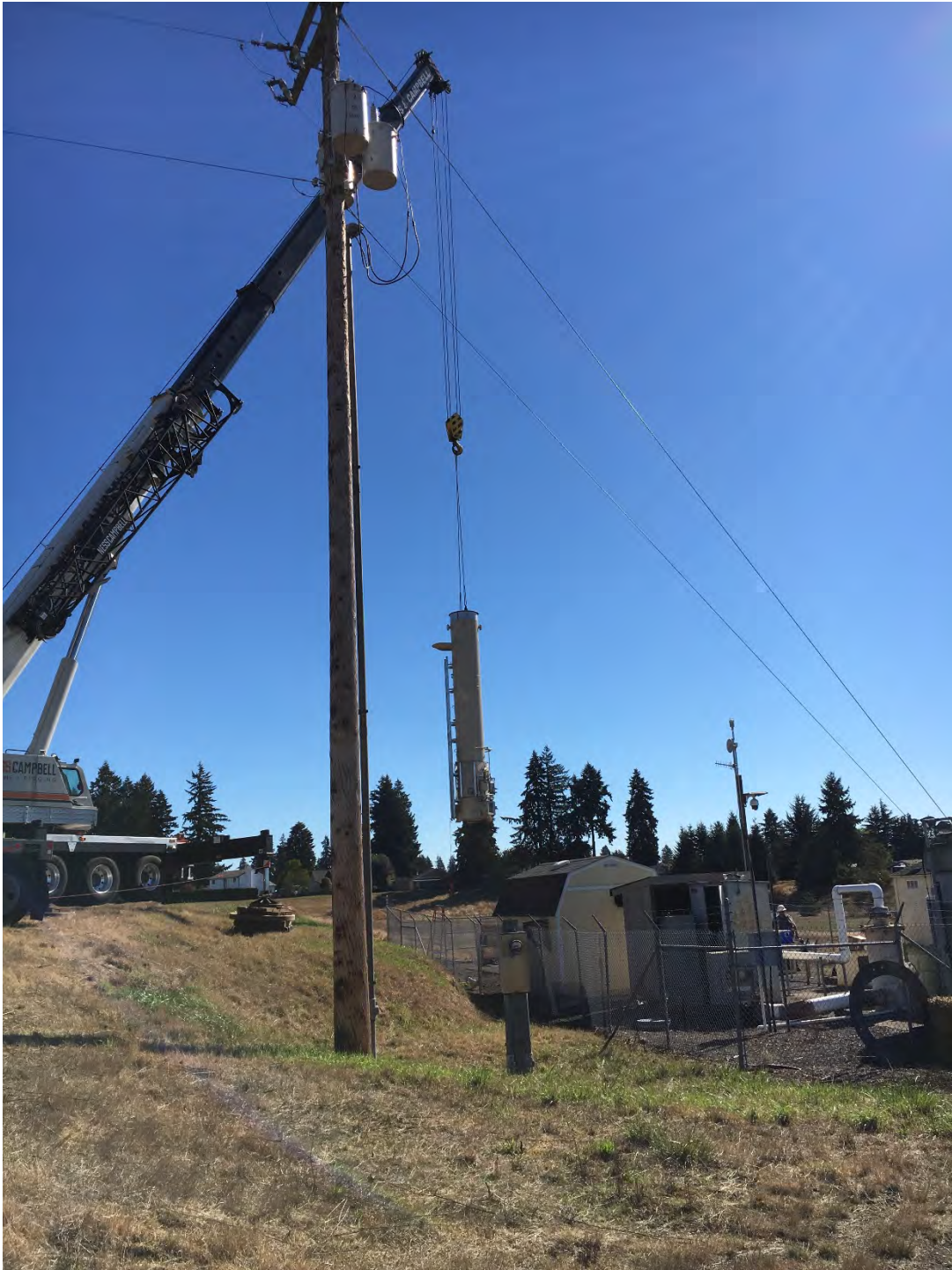
September 28, 2020 – lifting flare to flare pad
