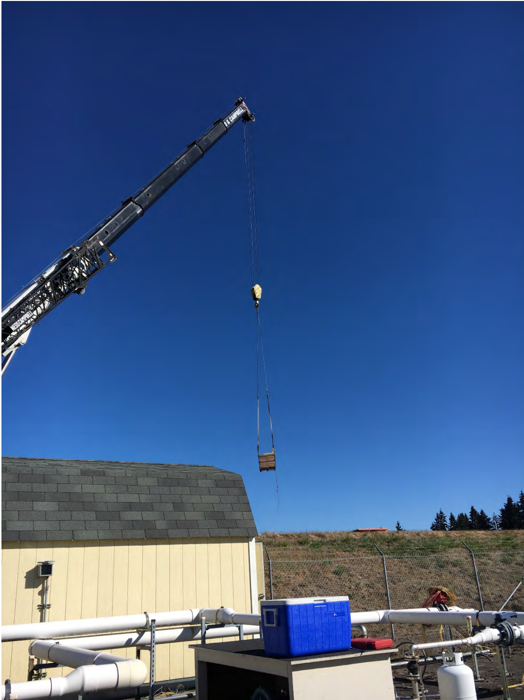
September 28, 2020 – lifting of parts and components to flare station compound
