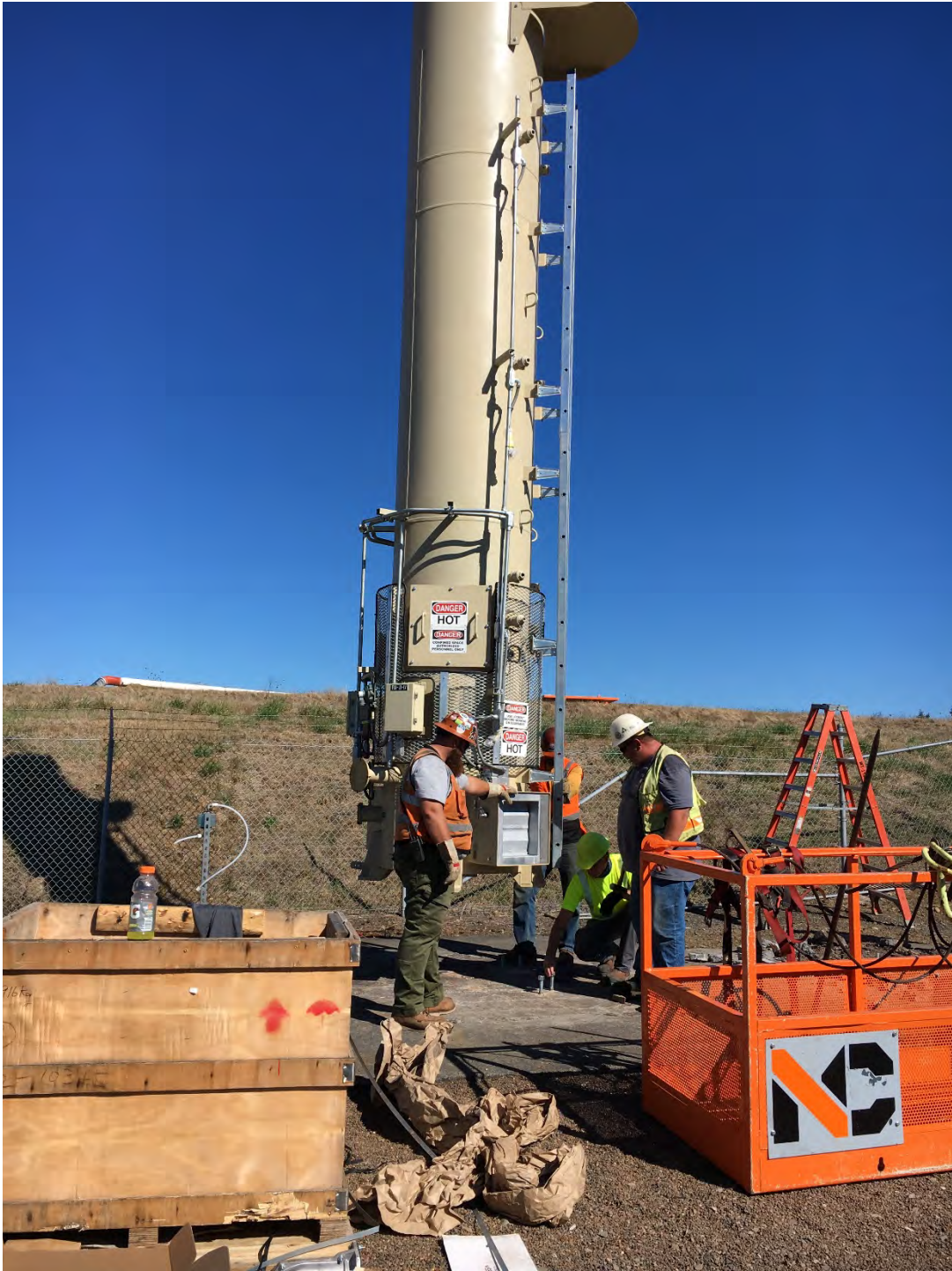
September 28, 2020 – repositioning bolts in flare pad
