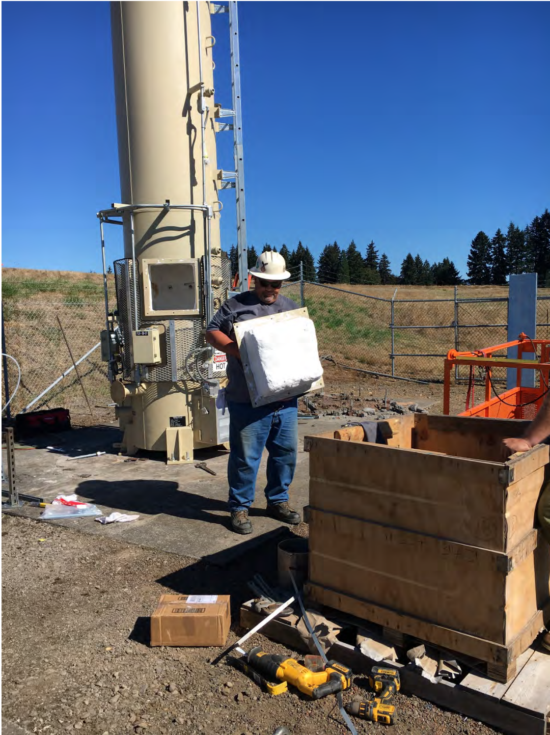
September 28, 2020 – side hatch door removal for burner pot placement
