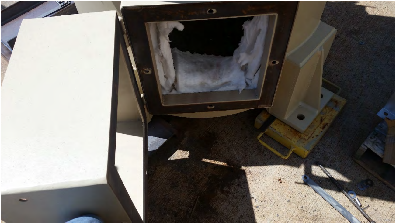
August 25, 2020 – Looking into flare louver boxes at Perennial manufacturing facility
