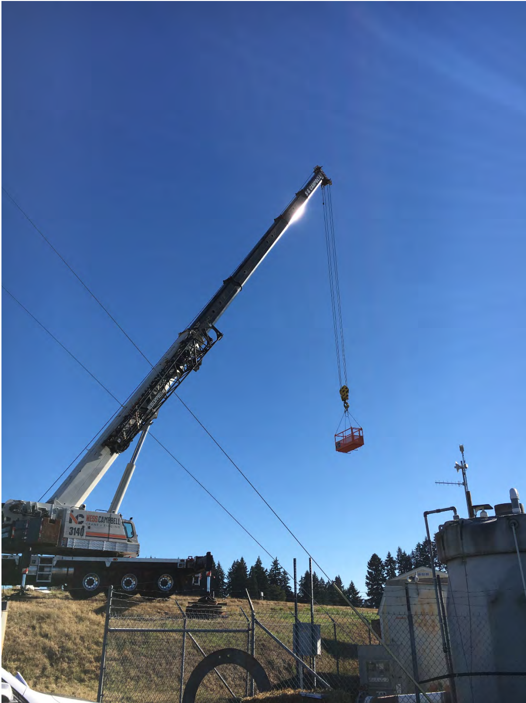
September 28, 2020 – Ness Campbell crane setup
