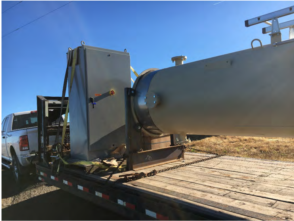
September 28, 2020 – Flare on delivery truck at Leichner Landfill, morning of installation
