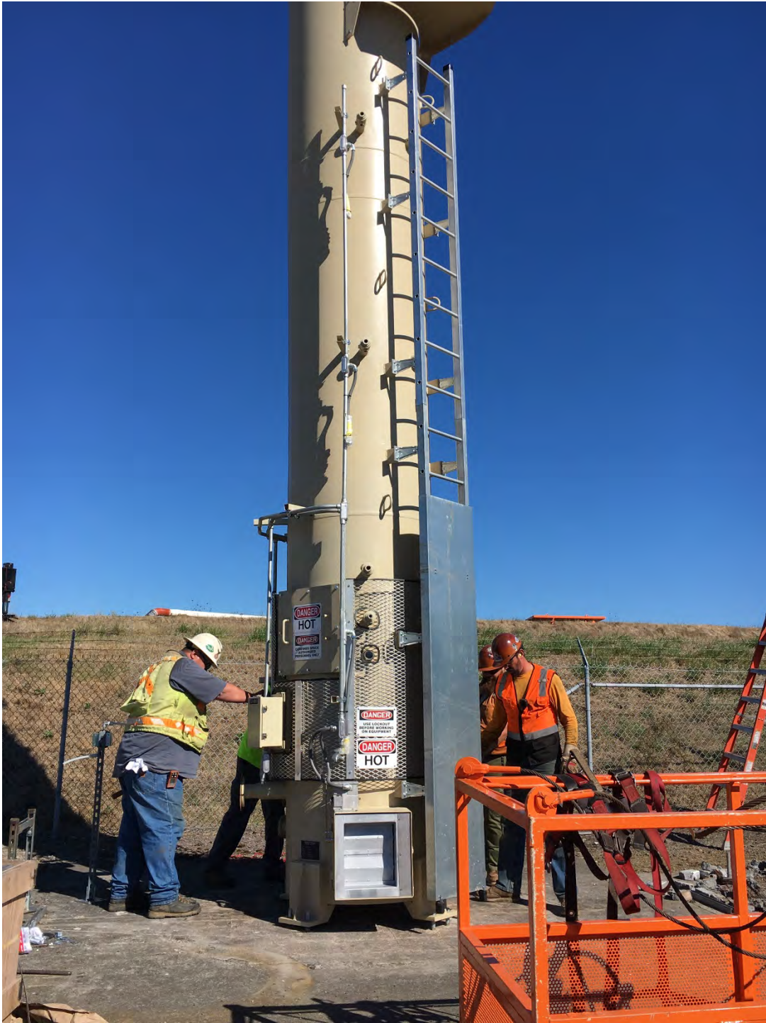
September 28, 2020 – aligning flare on bolts on flare pad
