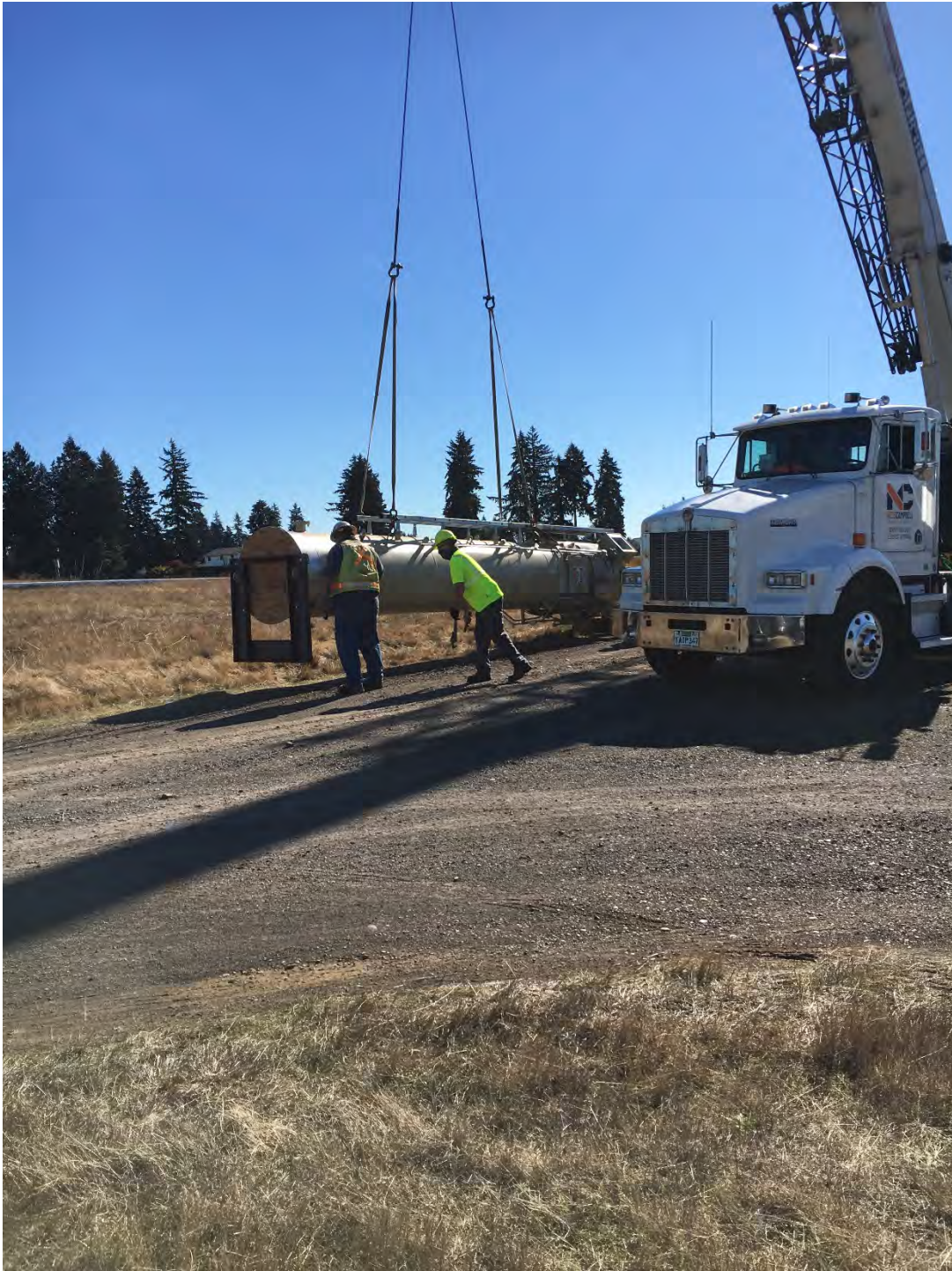
September 28, 2020 – setting new flare on ground to remove shipping stand
