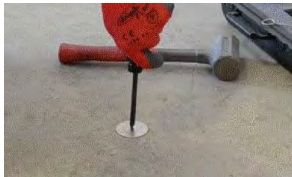
Figure 5. Tightening the Secured Cover.
