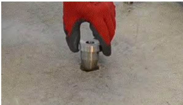
Figure 3. Installing the Drilling Guide.
