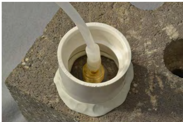
Figure 6. Water dam used for leak detection.
