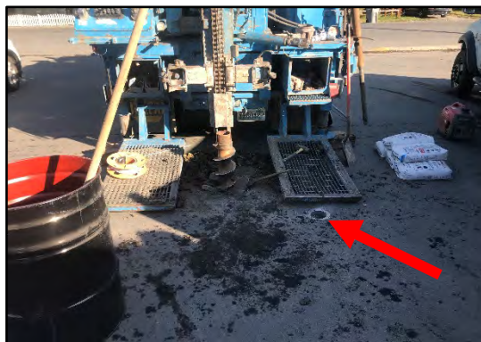
View of monitoring well MW-06 being installed north of the carwash. The historical MW-06 was decommissioned in place (see arrow).
