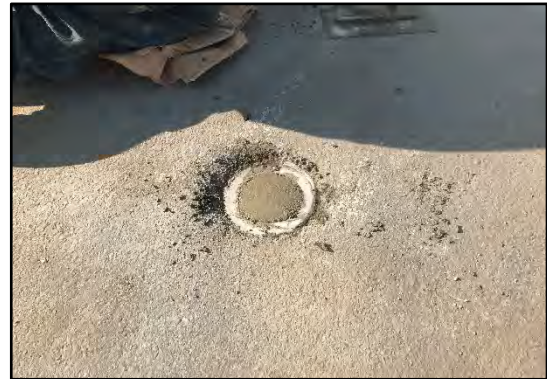
View of historical monitoring well MW-06 after decommissioning.
