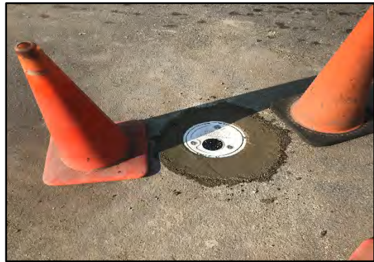
View of monitoring well MW-02 after completion of well installation.
