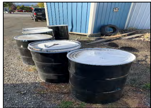
View of soil and waste water drums associated with September 29, 2020, well installation activities.
