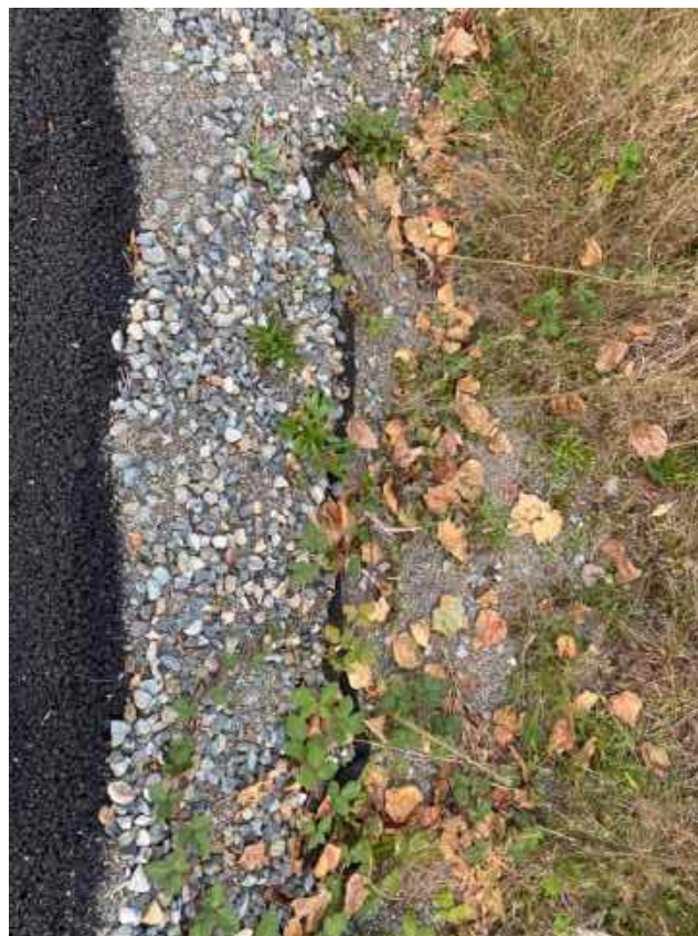
Photograph 4. This photograph shows the transition of the DMCA wildlife barrier to the surrounding ground surface near monitoring station DMCA 03.
