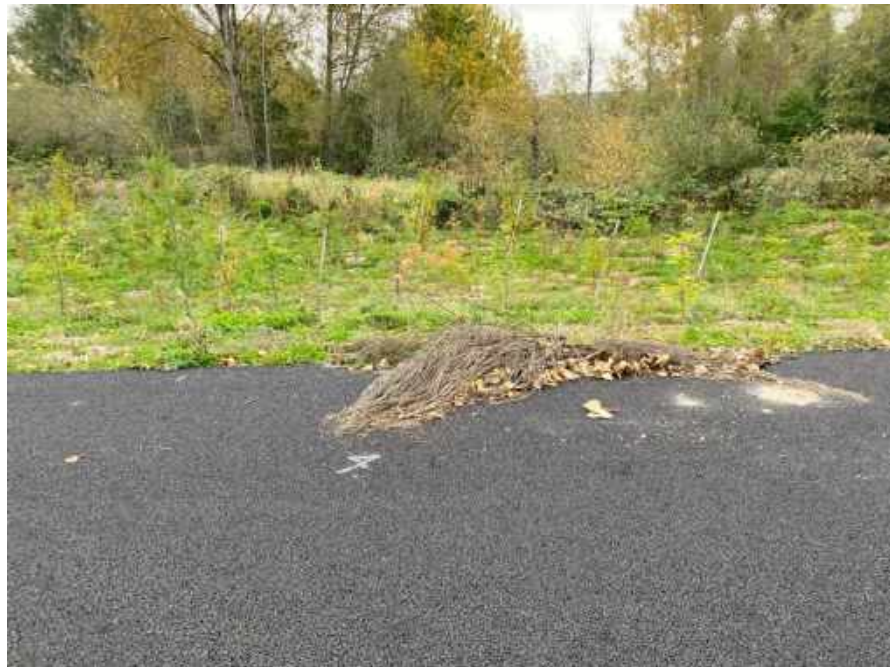
Photograph 8. This photograph was taken near monitoring station DMCA 07, facing southeast. Debris piled on pavement was observed at this location.
