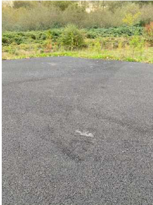
Photograph 7. This photograph was taken near monitoring station DMCA 06, facing southeast.
