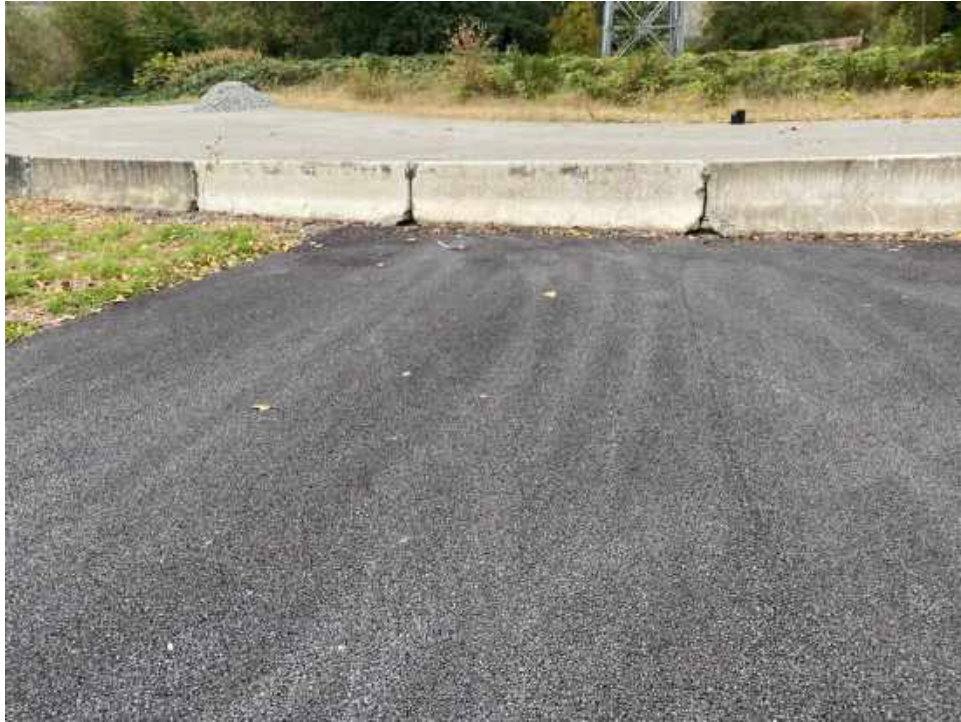
Photograph 9. This photograph was taken near monitoring station DMCA 08, facing south.
