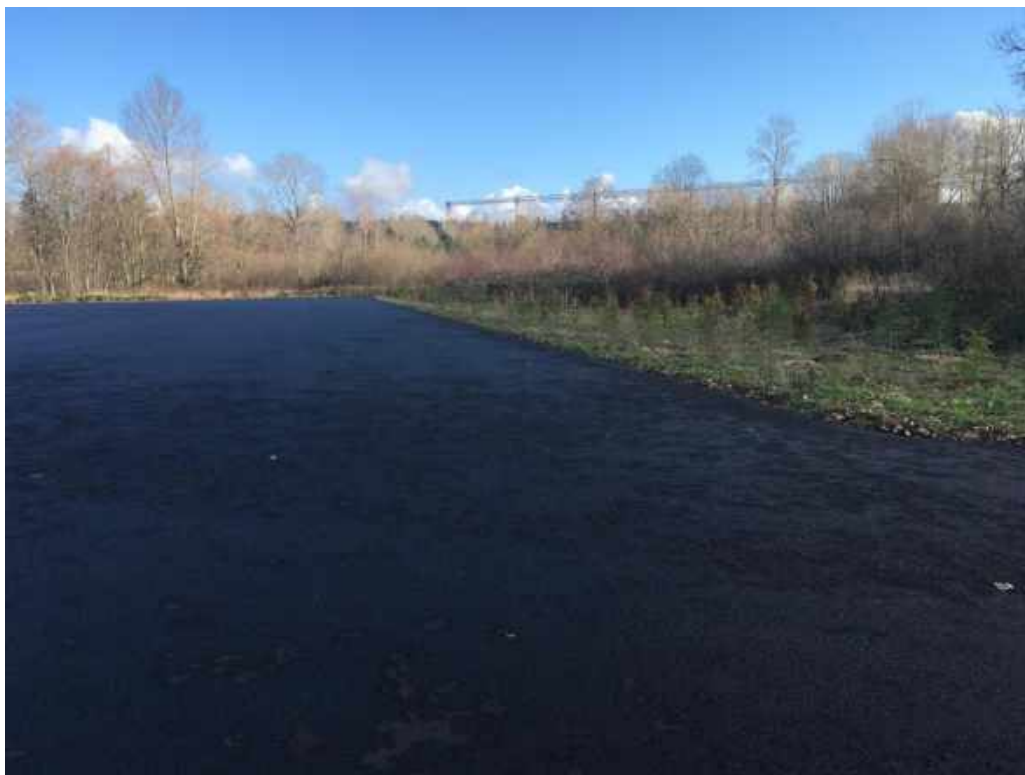
Photograph 4. Southern edge of the DMCA after removal of excess debris.
