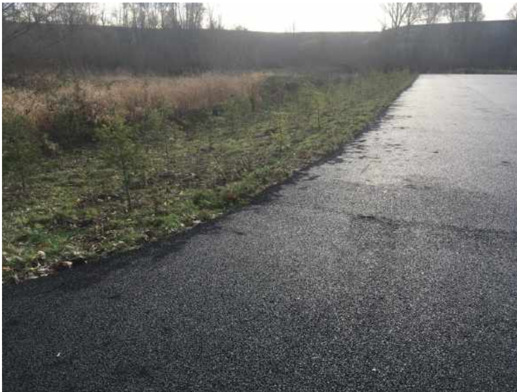
Photograph 2. Area near station DMCA 05 after removal of excess debris.
