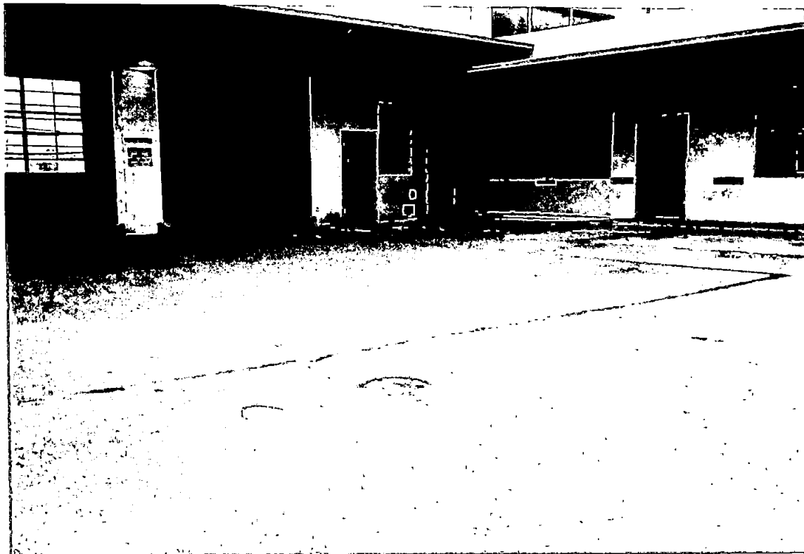
Photograph 8: View to the northeast towards inside of the "L" of the VMF building. The two underground hydraulic lift pit were located in the two bays seen in the left side of the photograph, and AOC #2 is seen in the foreground, where the edge of the new asphalt is the approximate edge of the excavation.
