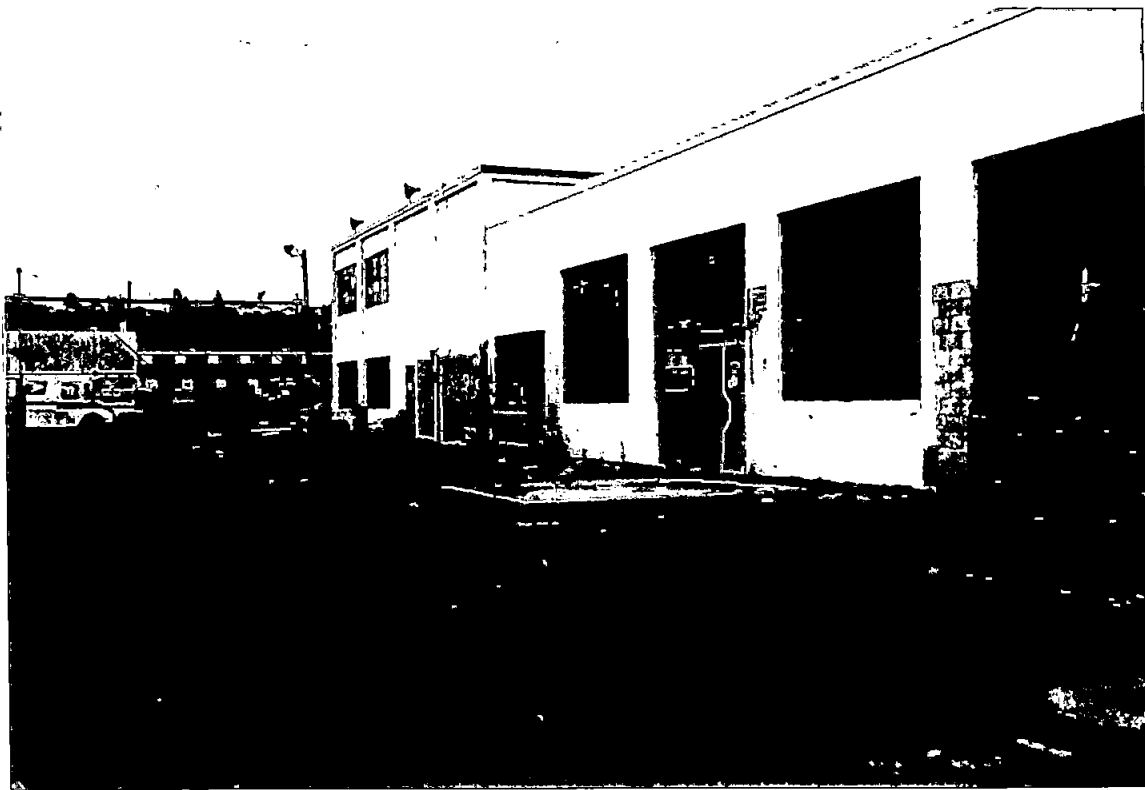
Photograph 5: View to the east along the north side of the VMF building.
