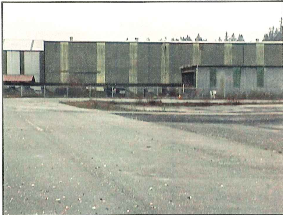
View of southern-central portion of site facing south.
