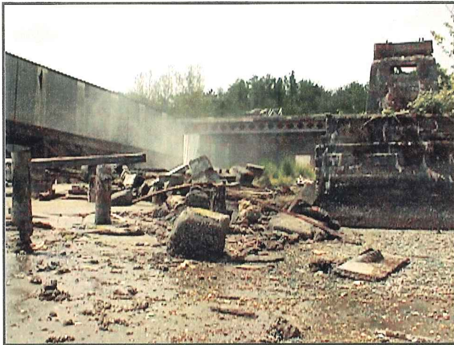
View of Reliable Steel Fabricators, Inc., facility from intertidal zone.
