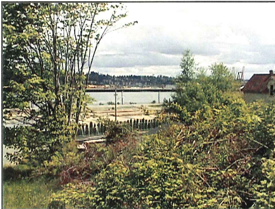
Overview of Hardel Plywood Facility facing southeast.
