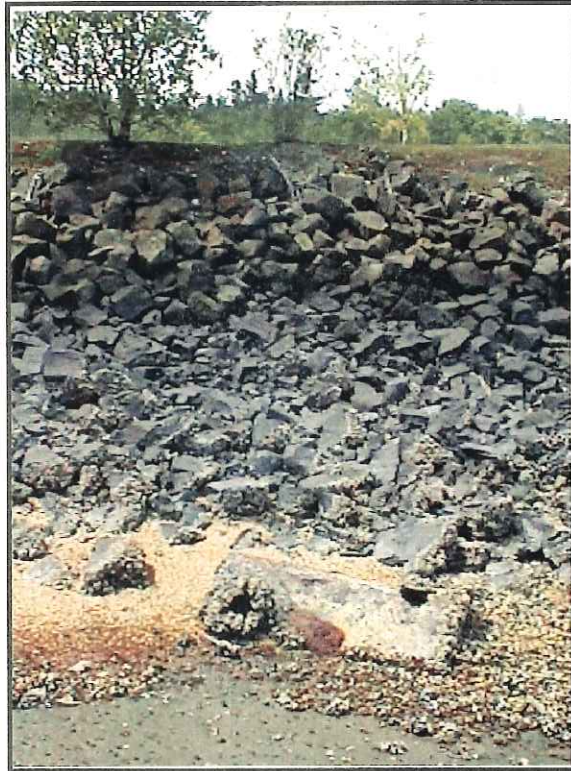
View of empty storage tank and iron stained sediments in intertidal zone.
