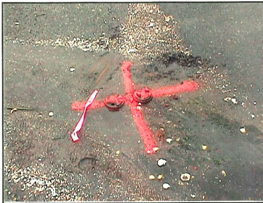
Close-up of two capped pipes (pt 114), probable part of stormwater drainage system.
