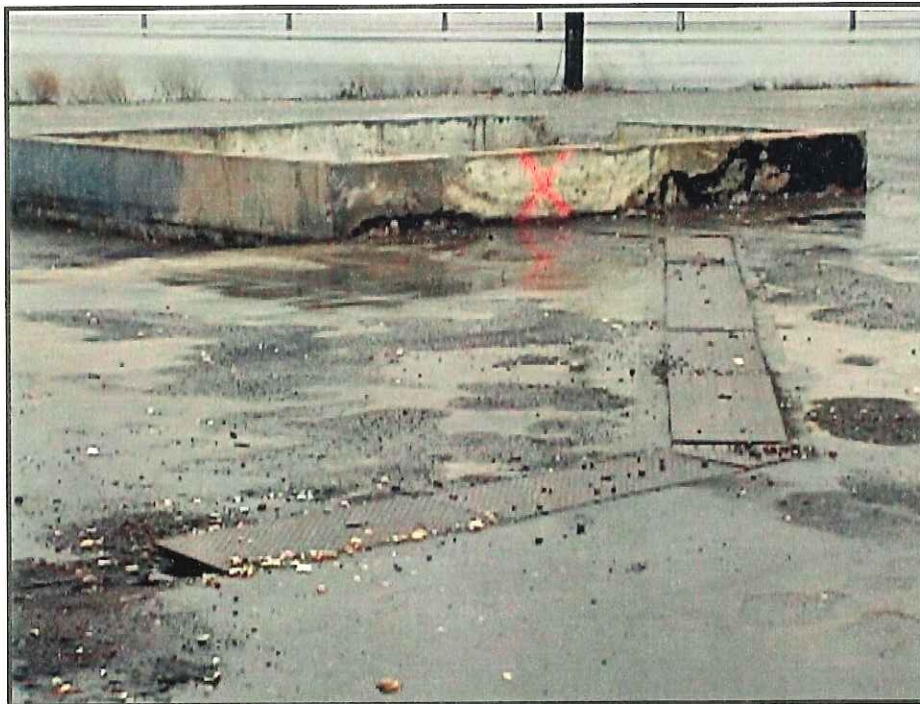
Glue spreader wastewater tank foundation (point 103).
