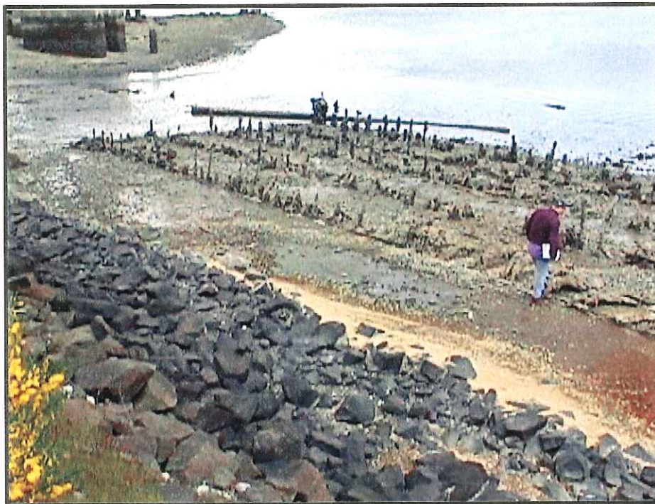
View of old pilings in southeast portion of property and iron stained sediments..
