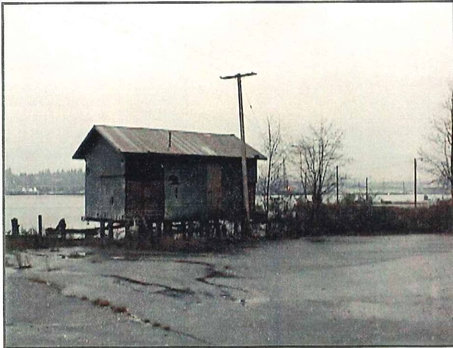
View of storage shed straddling northwestern property boundary, facing southeast.
