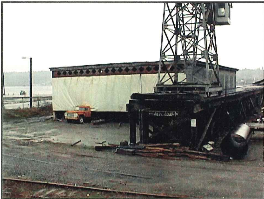
View of crane at Reliable Steel Fabricators, Inc.
