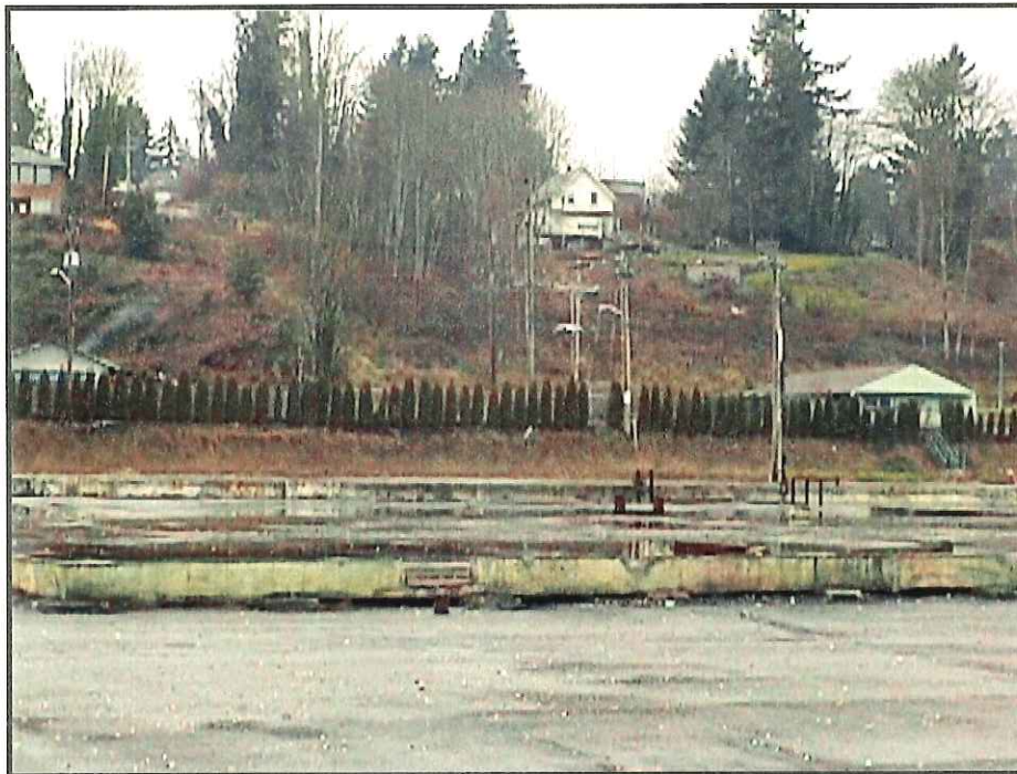
Overview of north-central portion of site facing west.
