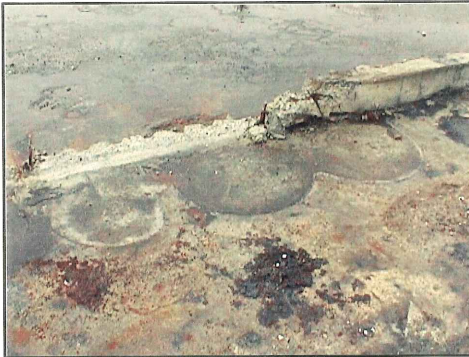
Close-up view of bermed area near resin and caustic storage area.
