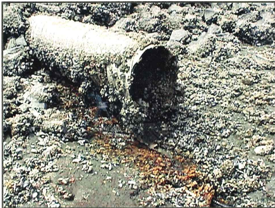
Close-up of southernmost storm sewer outfall.
