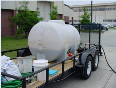
Figure 1: Bacteria food awaits injection into the Boeing Auburn site.
