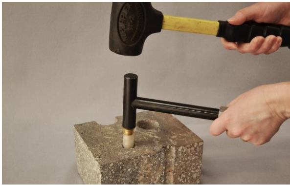
Figure 2. Installing the VAPOR PIN®
