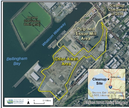
Aerial view of Georgia-Pacific West site
