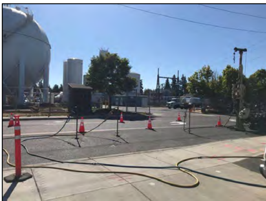
Photo 5: DPT injection wells on Row 11.
