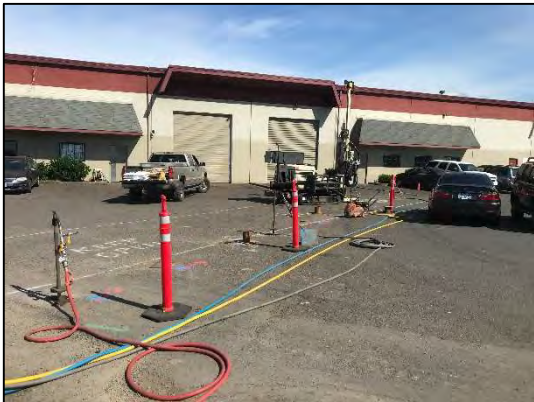
Photo 3: DPT injection wells on Row 9.
