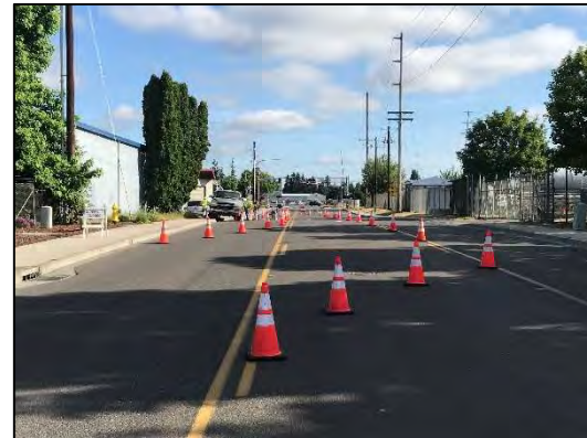
Photo 4: Roadway traffic control.
