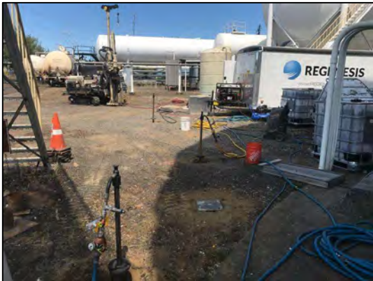
Photo 9: DPT injection wells on Row 13.
