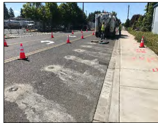
Photo 6: Row 11 air-knife clearing.
