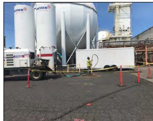
Photo 12: Row 14 air-knife clearing and traffic control for Messer plant trucks.
