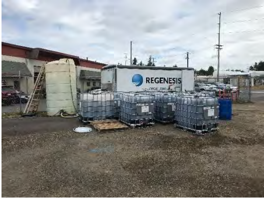
Photo 1: Product storage on-site and RRS Trailer.
