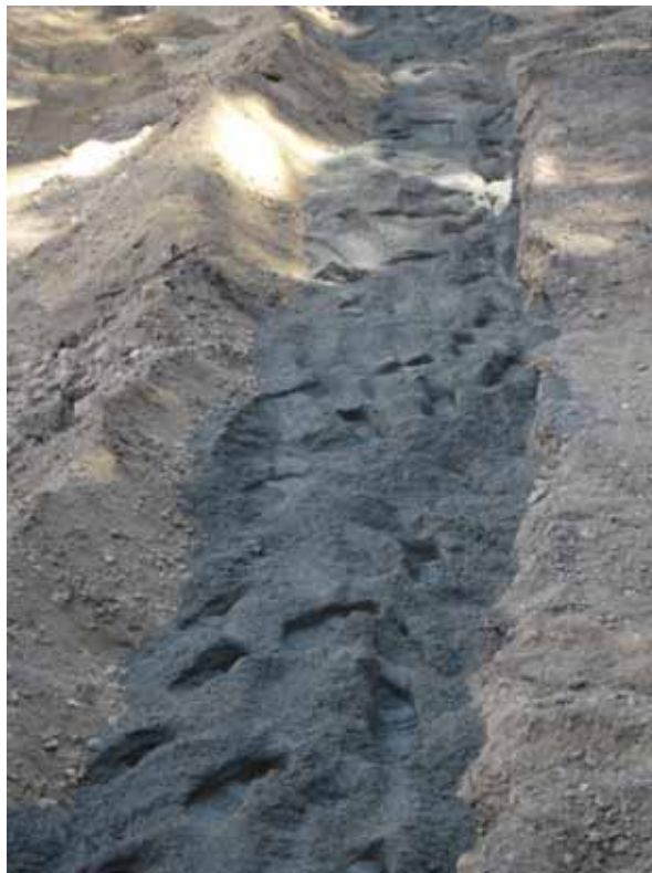
20. Morgan utility trench bedded in sand.
