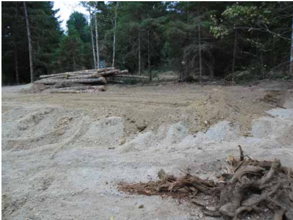
40. Hytec Spears south central trench mostly backfilled.
