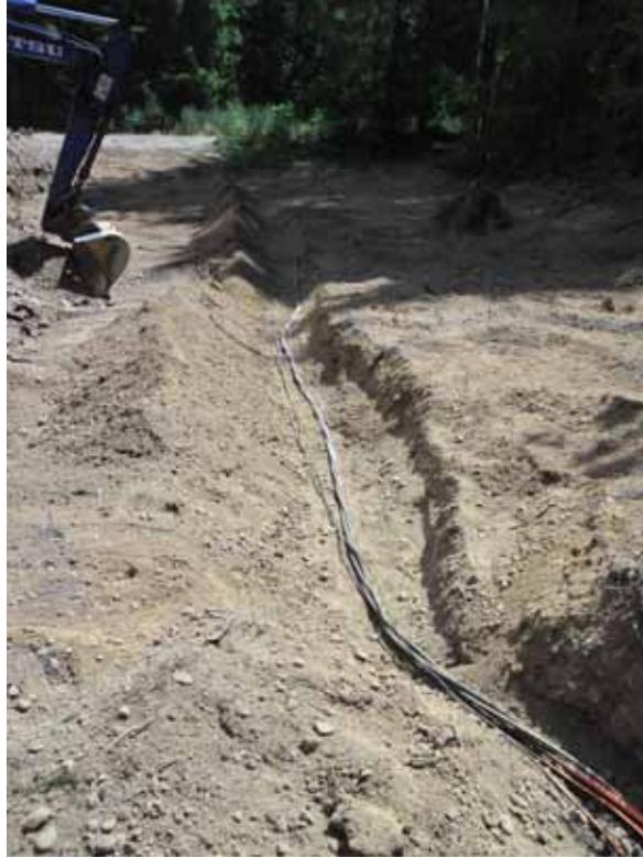
19. Morgan utility trench excavated (in HM sub unit)
