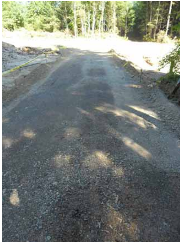
26. Temporary driveway restoration complete.
