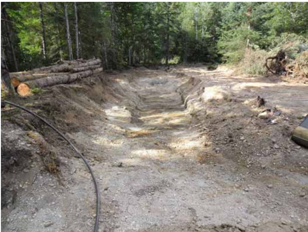
32. Hytec Spears (HS) sub unit south central trench.
