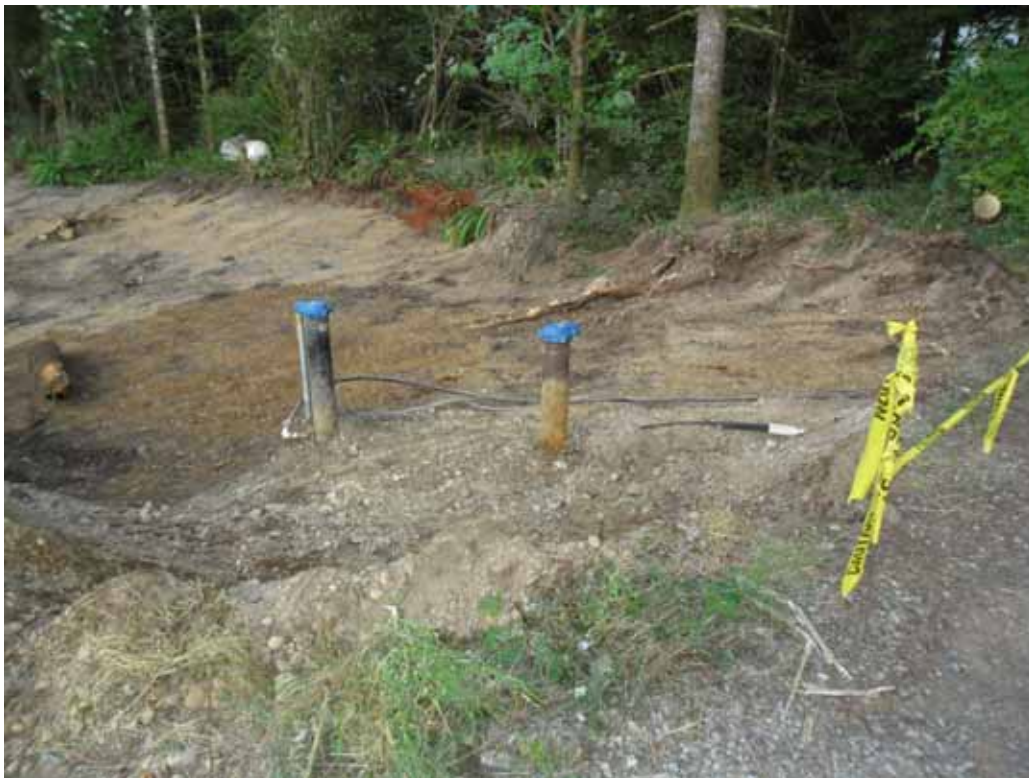
22. Debris cleaned from around Morgan and Spears wells.
