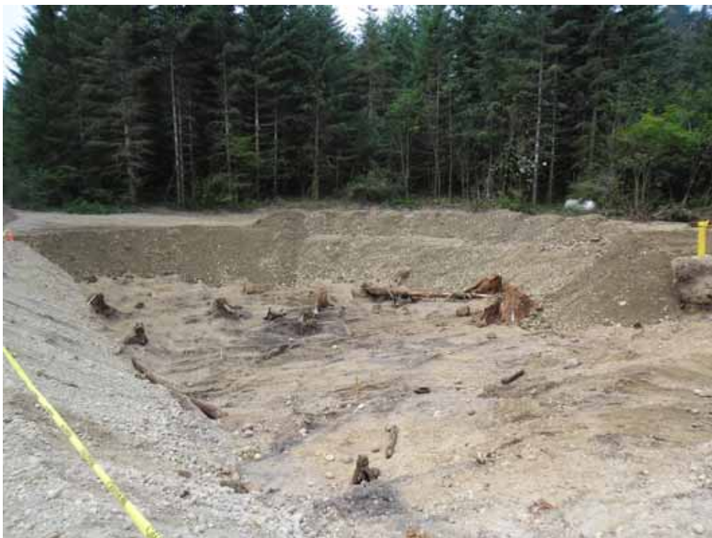
29. Backfilling Hytec Morgan (HM) sub unit
