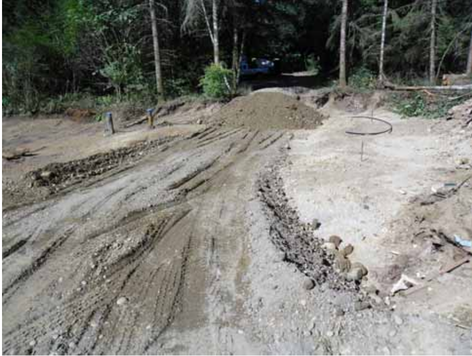
25. Debris removed from under Morgan driveway with driveway partially restored.
