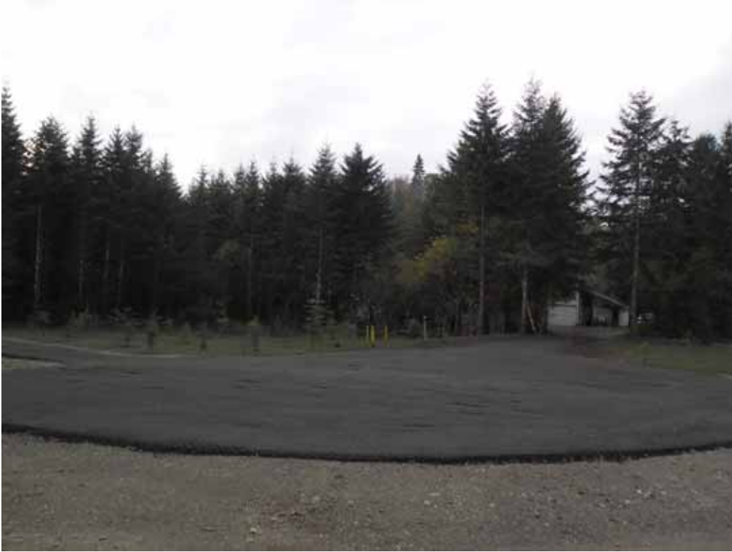
51. Road, cul-de-sac and driveway fully restored.
