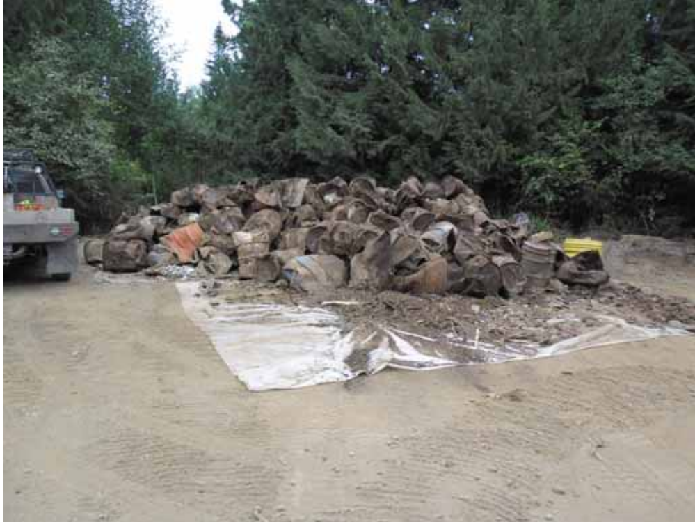
41. Crushed drum stockpile (as excavated)
