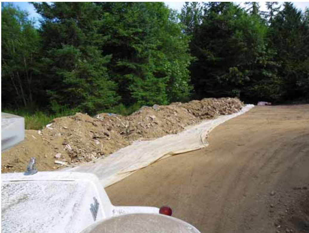
1. Debris stockpile from Hytec East (HE) sub unit.
