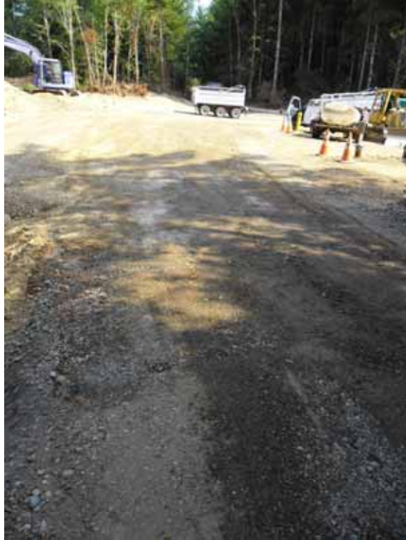
37. Morgan driveway restored.
