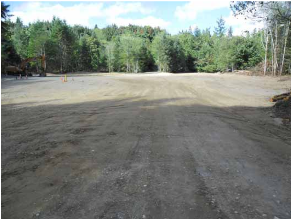
46. Overview of backfilled Fiberglass Debris Landfill site.
