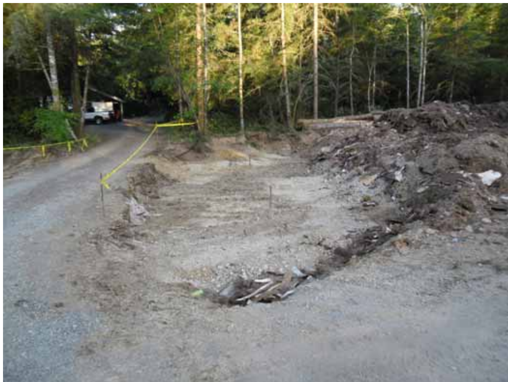
24. Debris removal on Hytec Spears (HS ) sub unit started.
