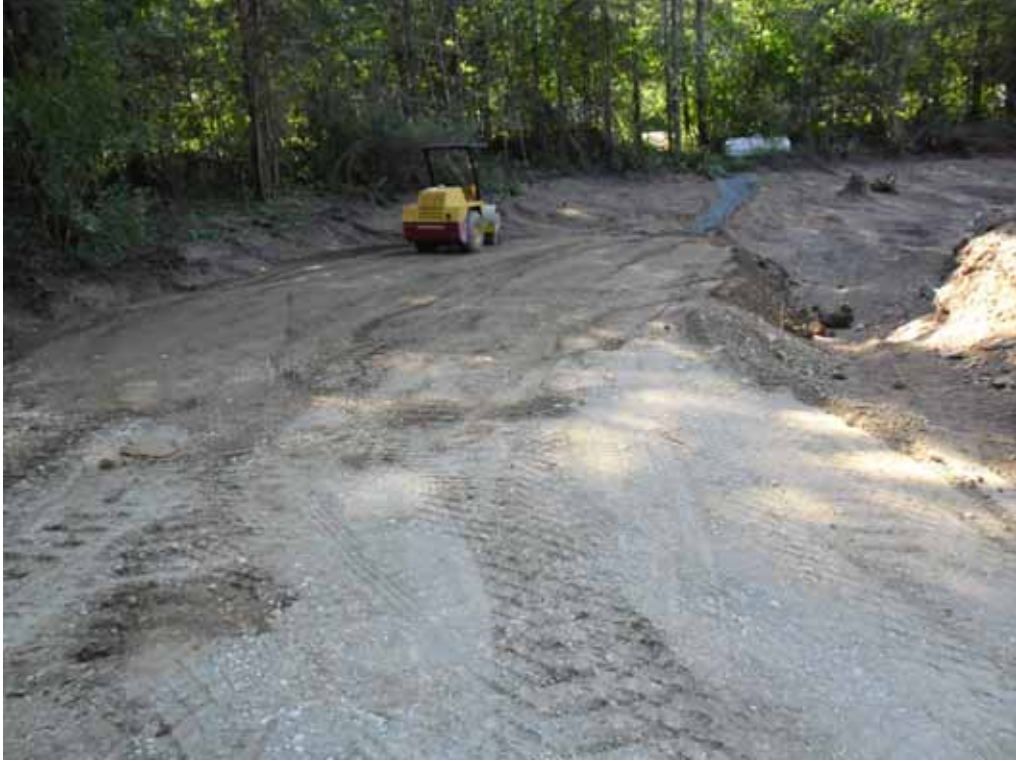
27. Backfill on Hytec Morgan (HM) sub unit.
