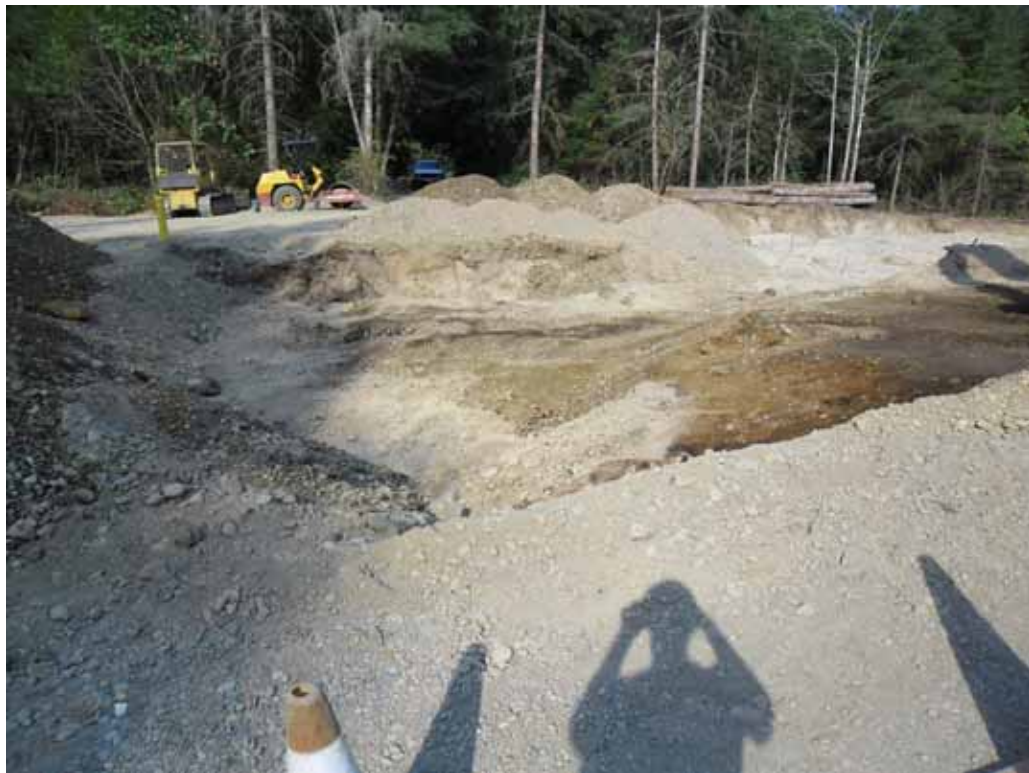
36. Last of Morgan driveway and cul-de-sac excavation.
