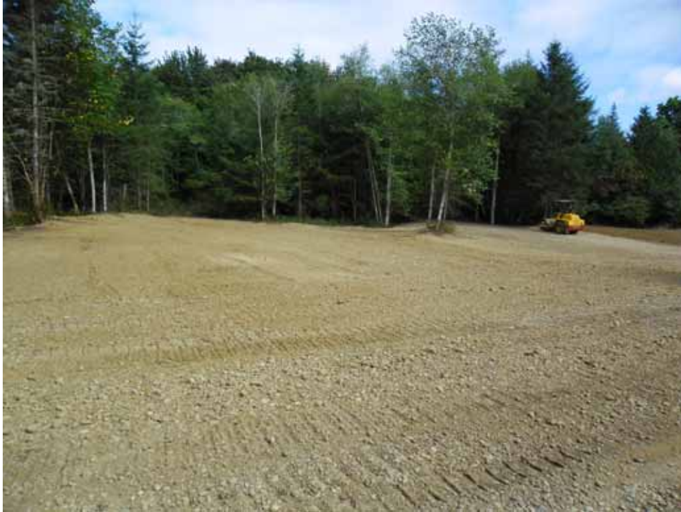
43. Hytec Spears backfilled.
