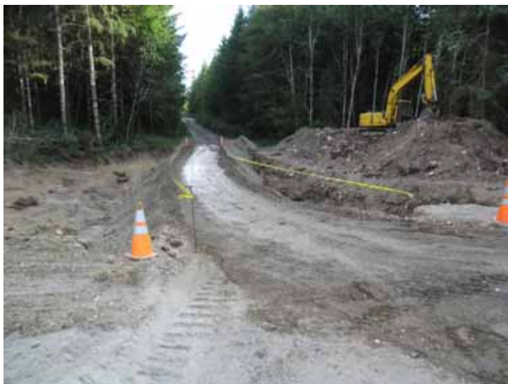
12. Temporary road watered and rolled.
