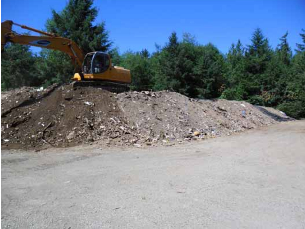
31. Hytec debris stockpile.
