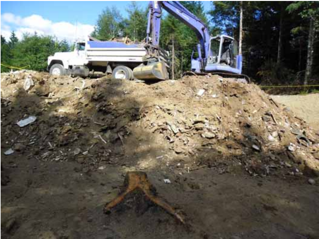
28. Loading out road spoils debris.
