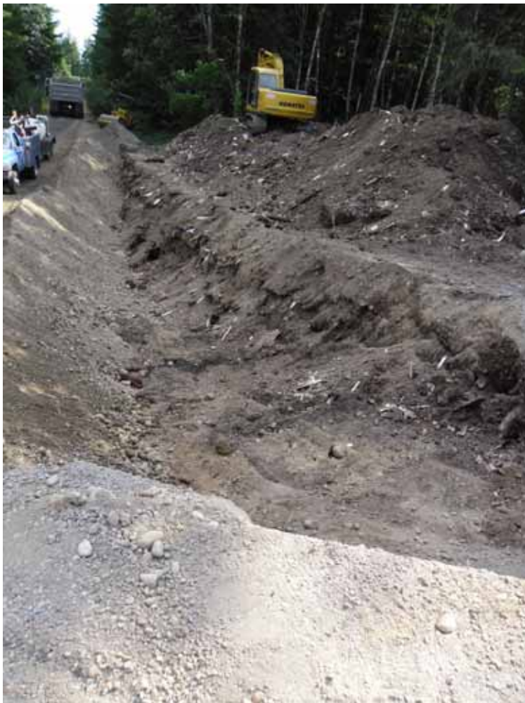
10. Debris under road excavated.
