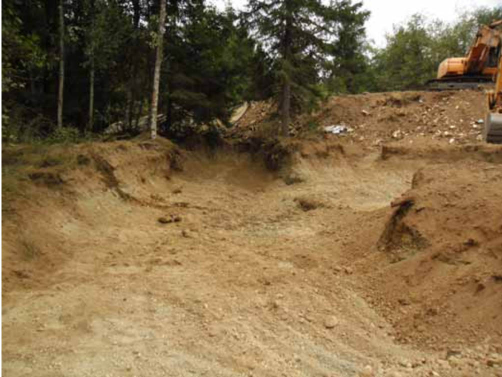
39. East end of drum trench excavated.
