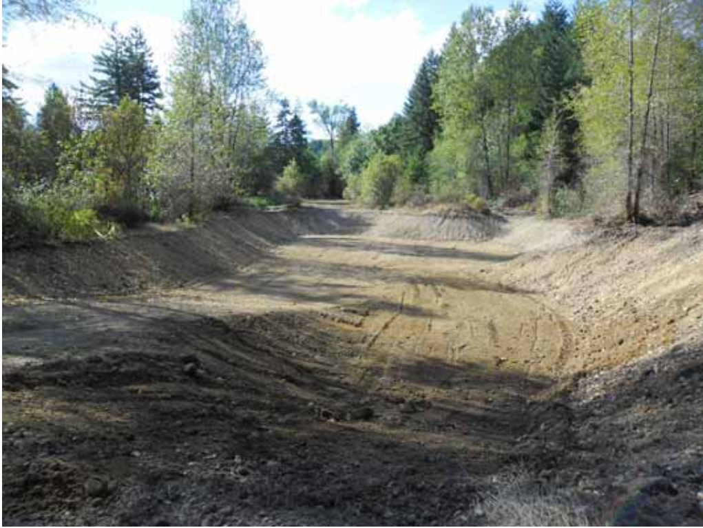
47. Borrow pit final grading.
