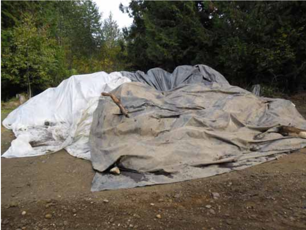
53. Final waste pile covered and awaiting trucks.
