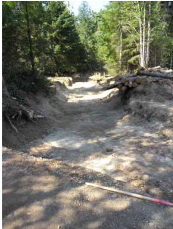
38. Hytec Spears west trench excavated.
