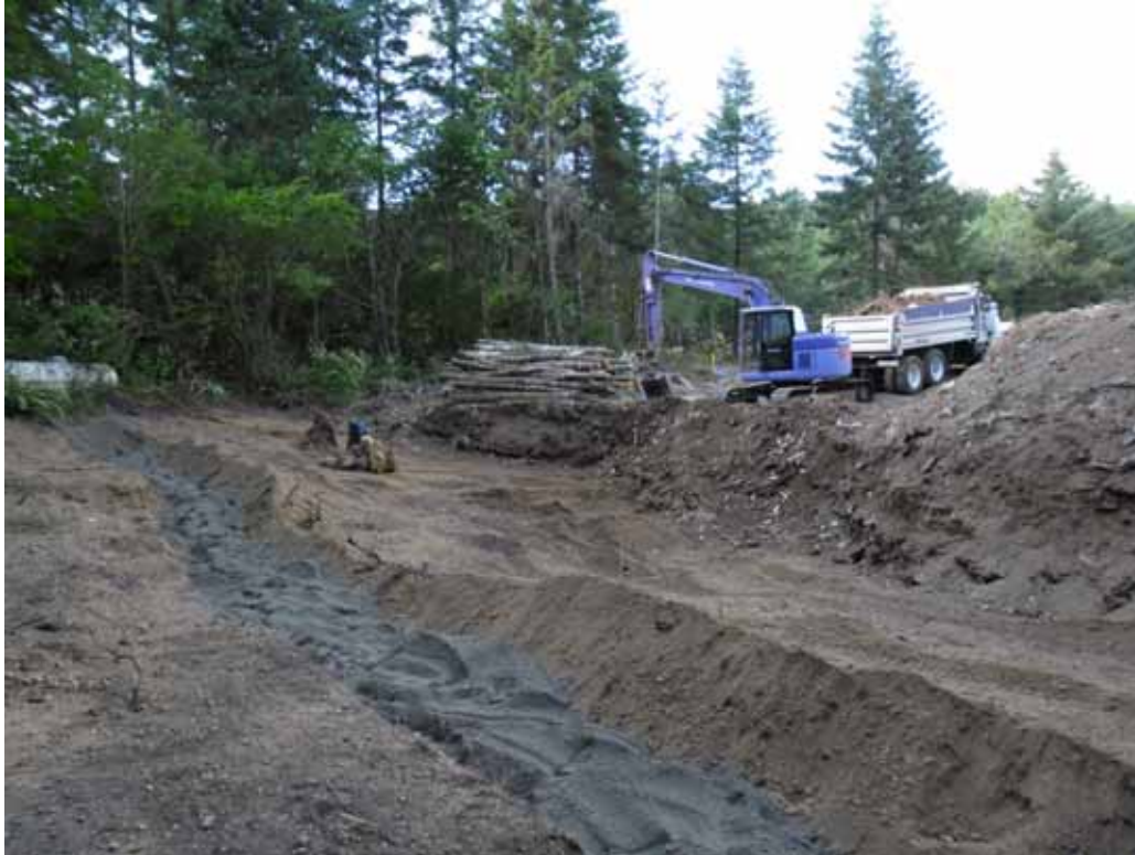
21. Hytec Morgan (HM sub unit) debris being excavated.
