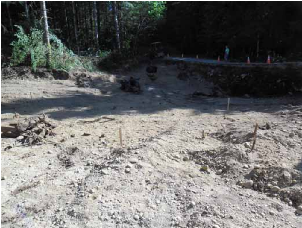
8. Hytec east subunit with excavation and sampling completed.
