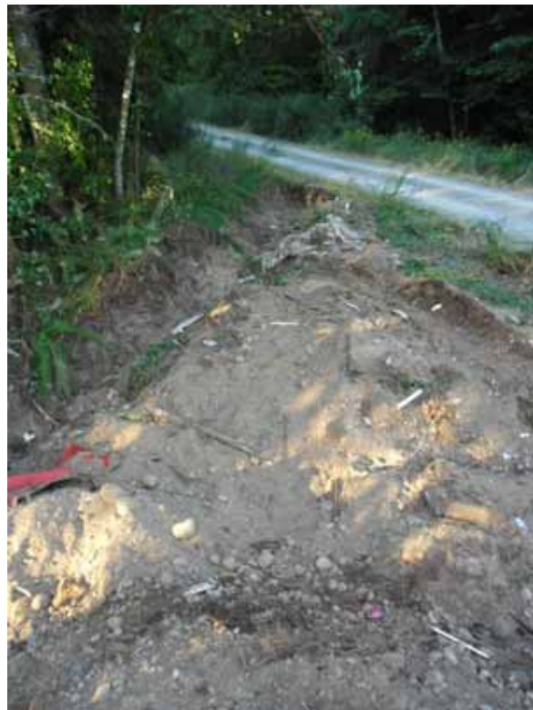
4. South end of Hytec East (HE) sub unit
