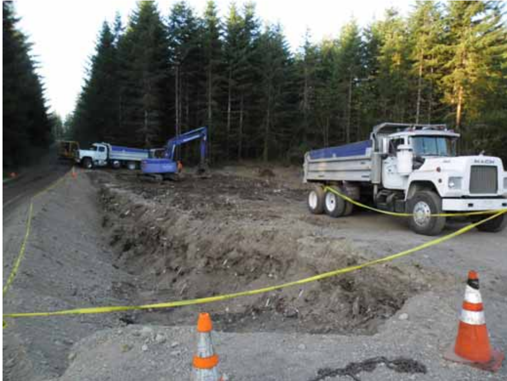
23. Debris from under road removed.
