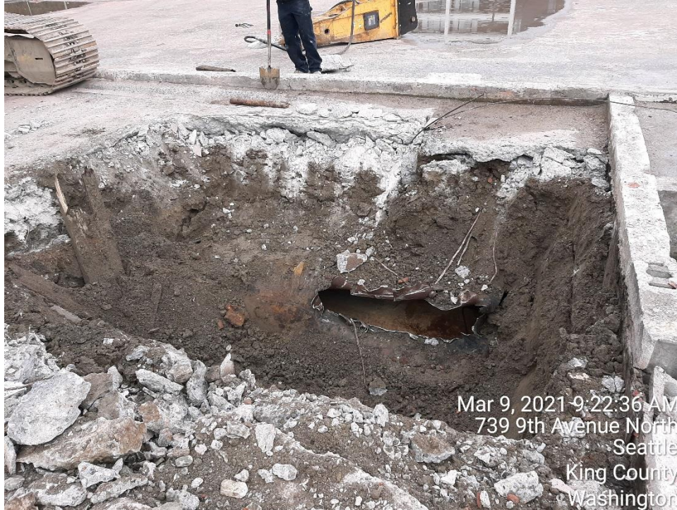
Photograph 1: UST-L excavation showing UST-L tank opened to inspect fill material.
