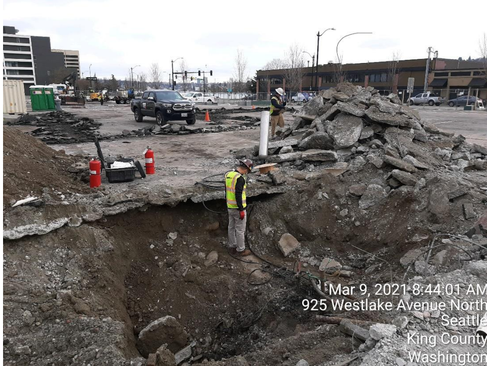
Photograph 5: Marine Chemist inerting UST-A.
