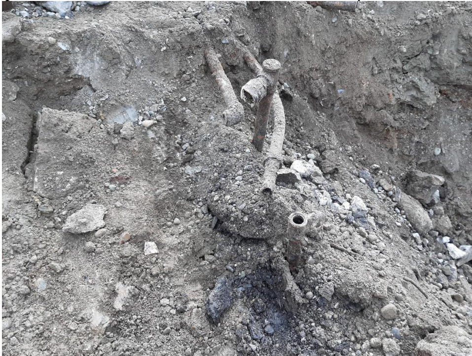
Photograph 4: Uncovering the top of UST-A and associated piping. Note, oil-soaked soil around lines at top of tank.
