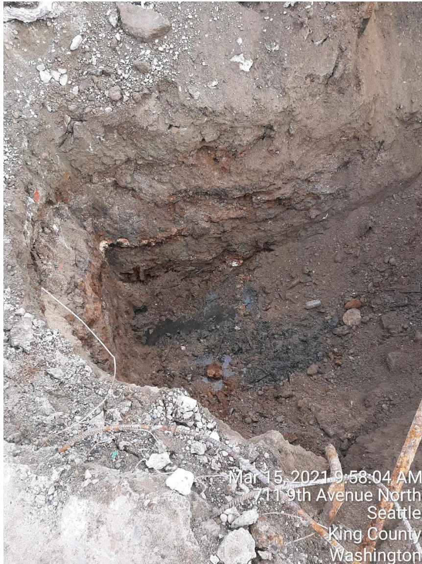
Photograph 10: Above right. Groundwater with sheen entering southwestern corner of UST-A excavation at a depth of 15 feet bgs.
