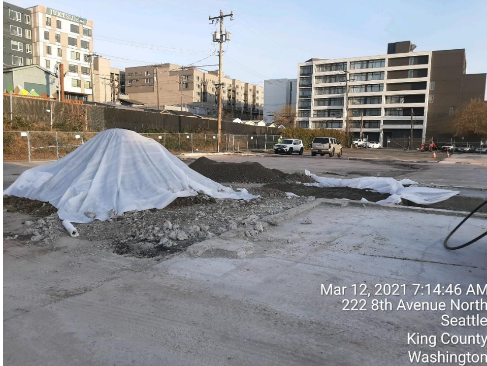
Photograph 3: UST-L lined and backfilled excavation and stockpile, viewed from the south.
