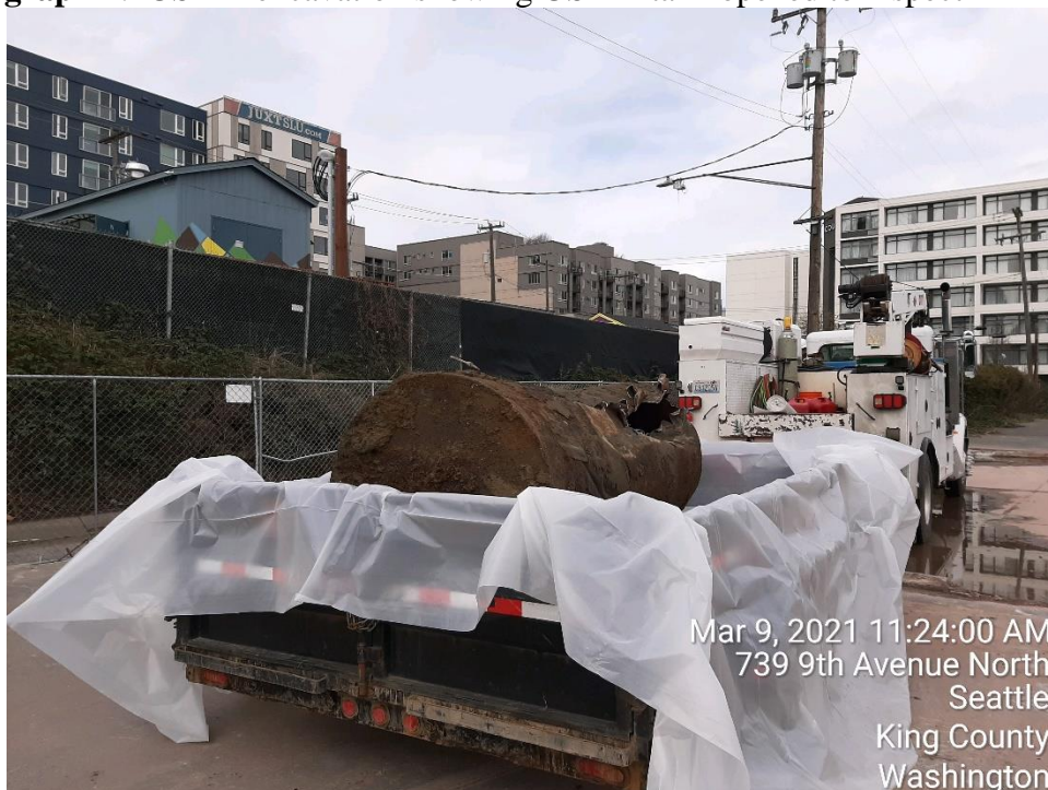
Photograph 2: UST-L removed from the excavation.
