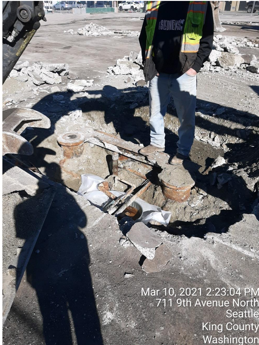
Photograph 17: Below left. ECI cutting lines at Hoist-5 and draining remaining oil.
