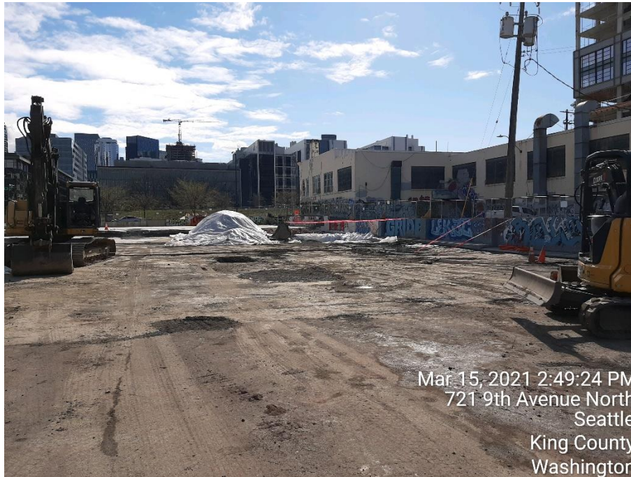
Photograph 24: Western hoists lined, backfilled, and compacted.
