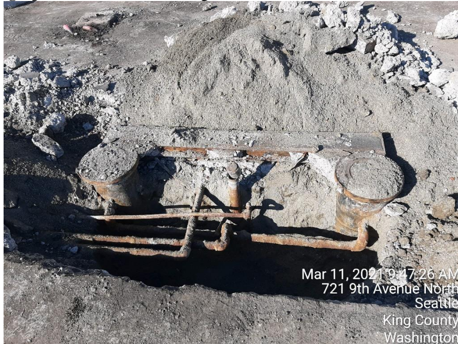
Photograph 15: Mar-Vac removing oil from accessible hoist reservoir fill lines.
