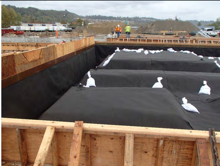
Photograph 19 Top layer of geofabric
