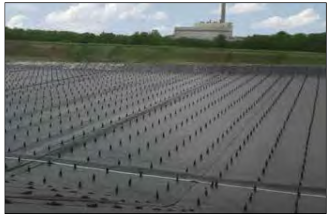
Landfill Rainshed Cover
