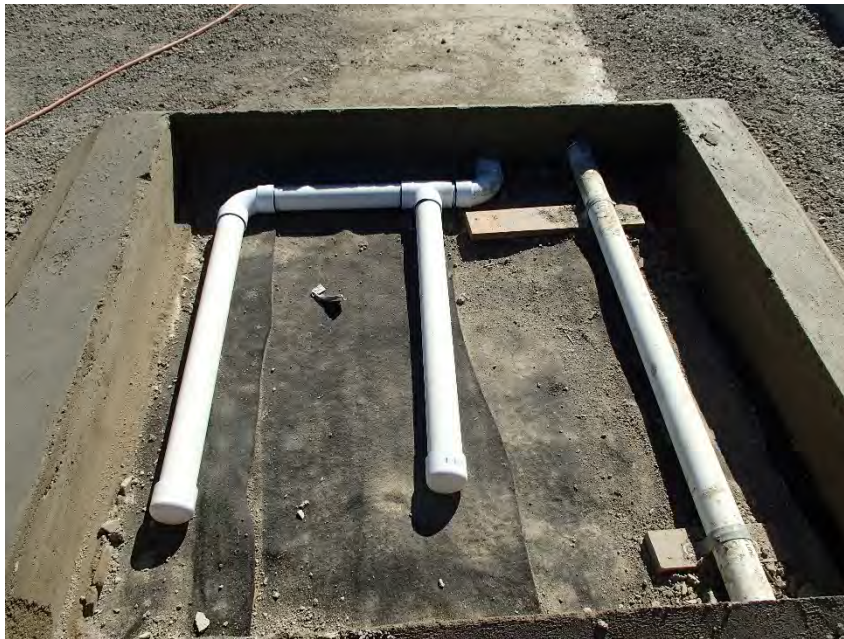
Photograph 9 Final pipe layout in Cell 5-A
