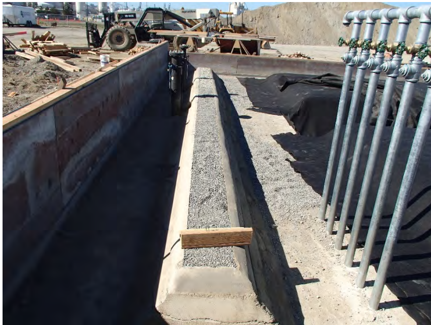
Photograph 12 Gravel backfill and bottom layer of geofabric
