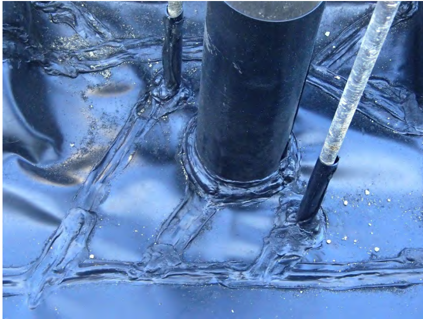
Photograph 15 Liner boot welds
