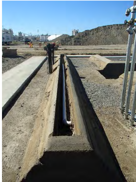
Photograph 8 Final pipe layout in Cell 3-E
