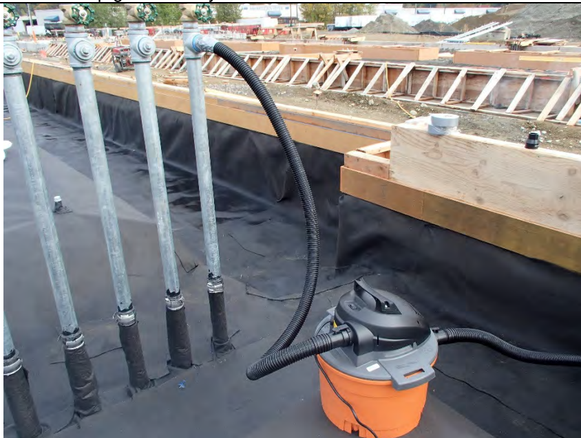
Photograph 22 Smoke testing liner
