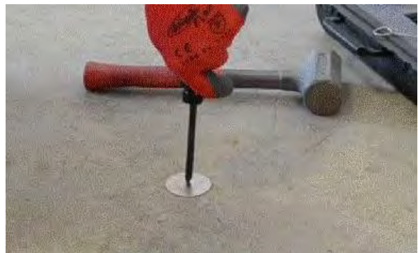
Figure 5. Tightening the Secured Cover.
