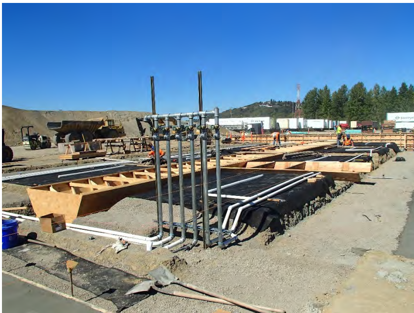
Photograph 2 Overview of project site and manifold
