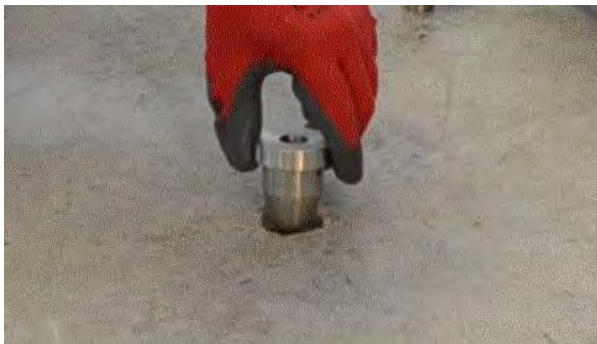
Figure 3. Installing the Drilling Guide.
