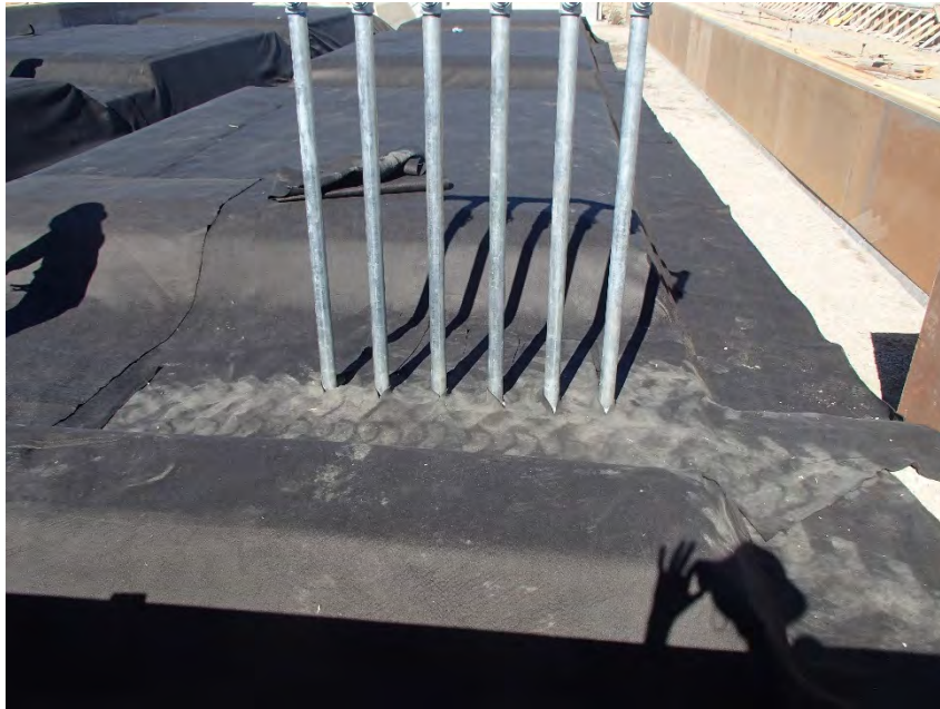
Photograph 13 Bottom layer of geofabric
