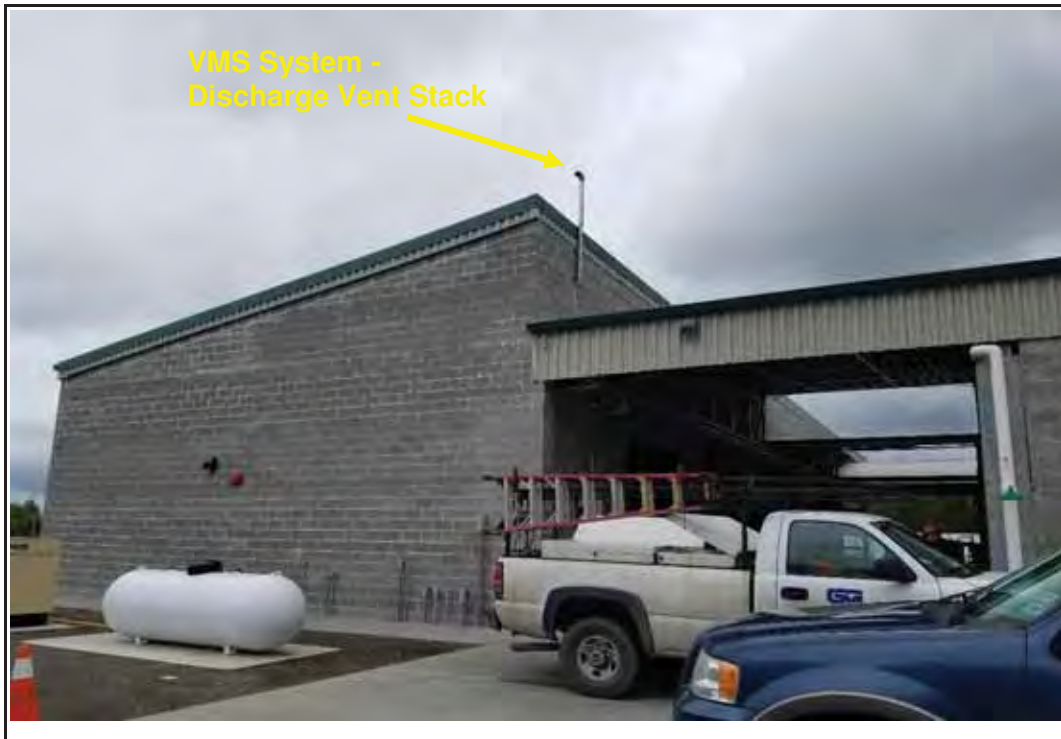
Photo 3: View of the south side of the receiving building showing the vent stack in the center of the picture at the roof line. Mechanical room is on south side of building.
