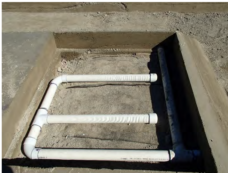
Photograph 10 Final pipe layout in Cell 4-AA
