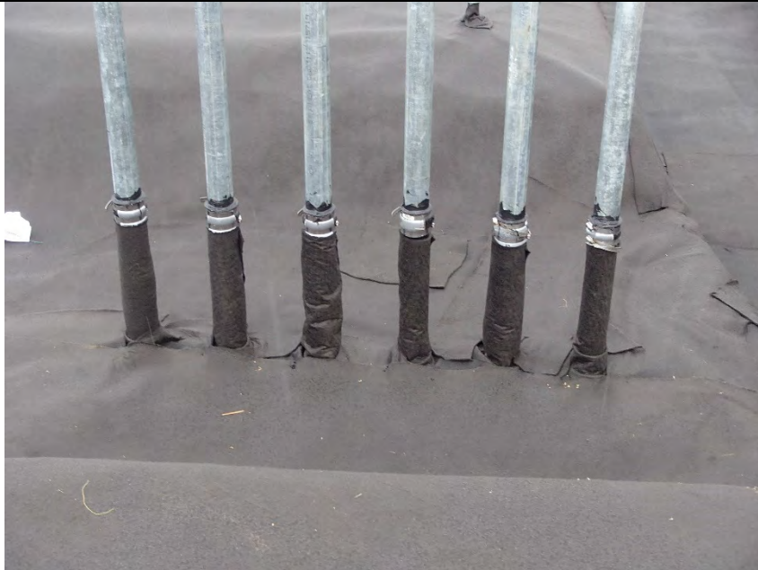
Photograph 21 Manifold top geofabric layer
