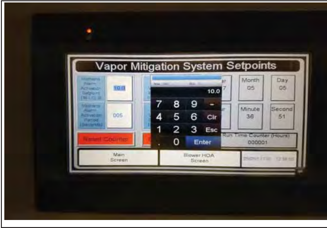
Photo 19: View of the VMS Control Panel - System Setpoints screen with the numeric touchpad active to help program in set point values or date/time values.
