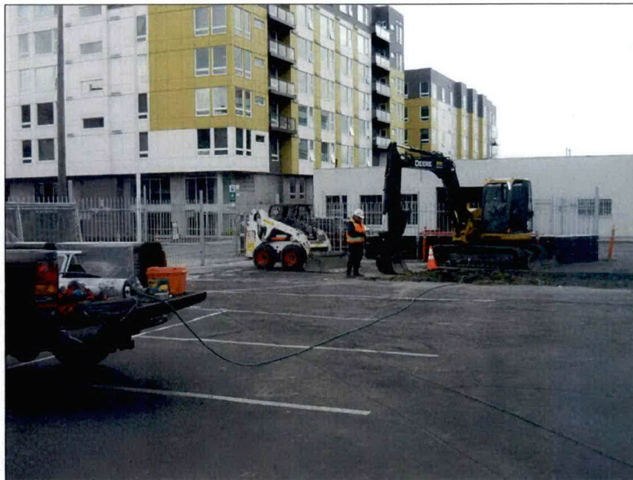
Photograph 2: Marine chemist inserting the USTs.
