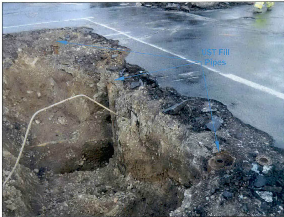
Photograph 1: The three uncovered UST fill pipes.
