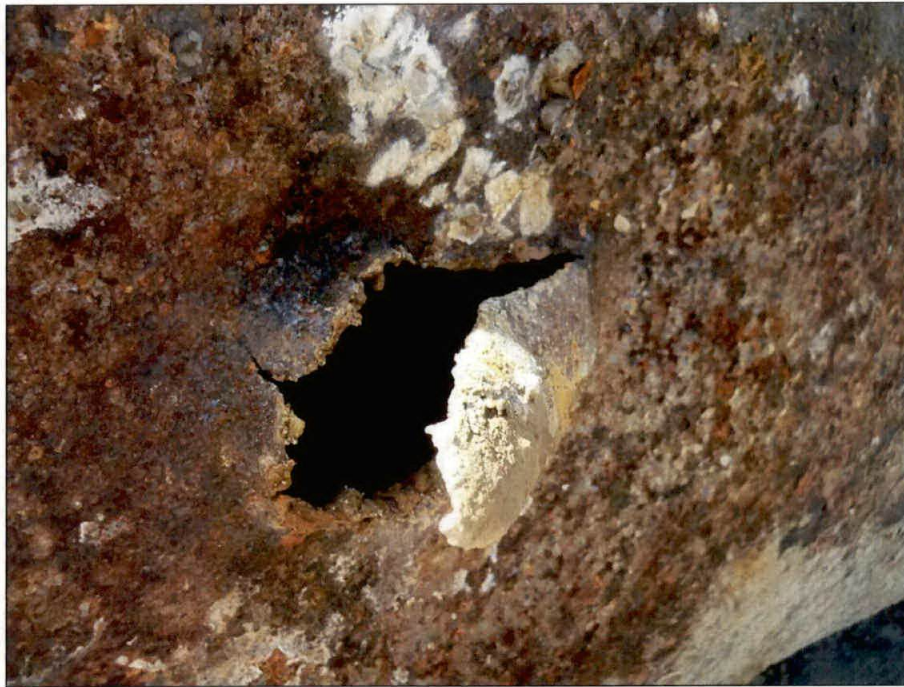
Photograph 9: Borehole in UST1.
