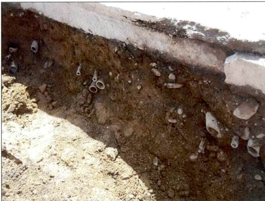
Photograph 12: Piping in the southwestern corner of the UST excavation.
