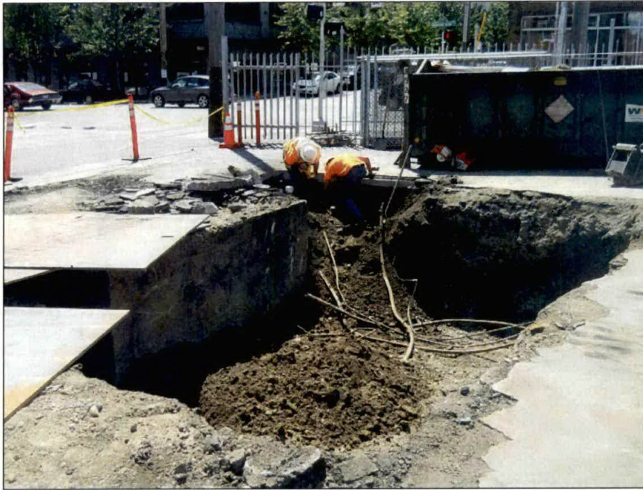
Photograph 11: Excavation in the southwestern corner where product piping was located.
