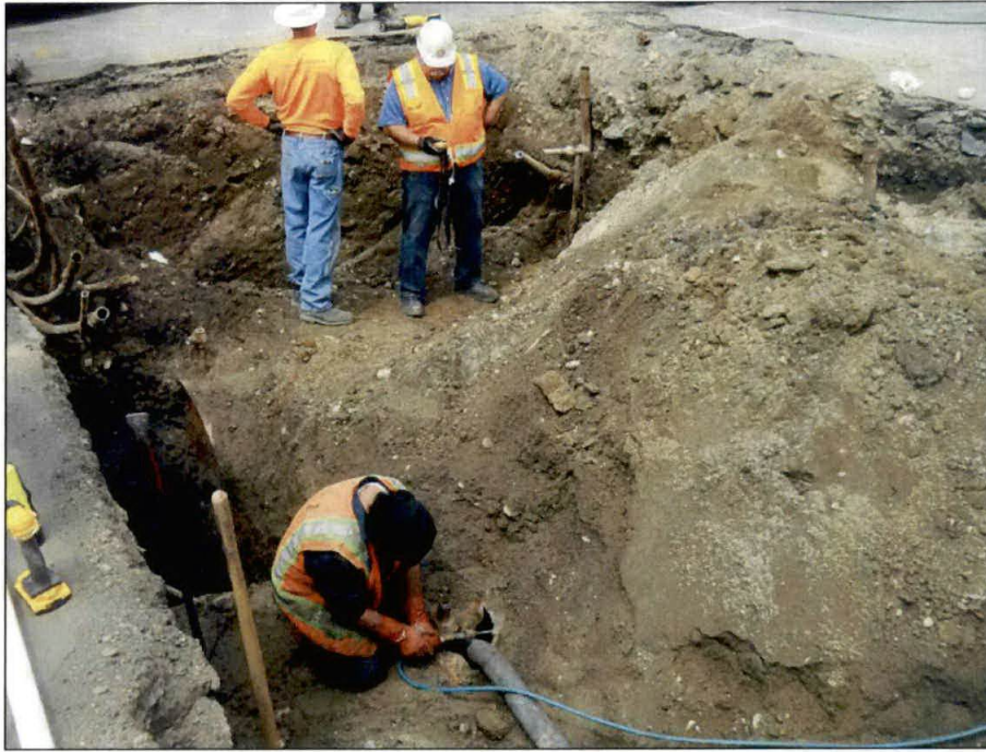
Photograph 3: Mar-Vac pumping and rinsing the USTs.
