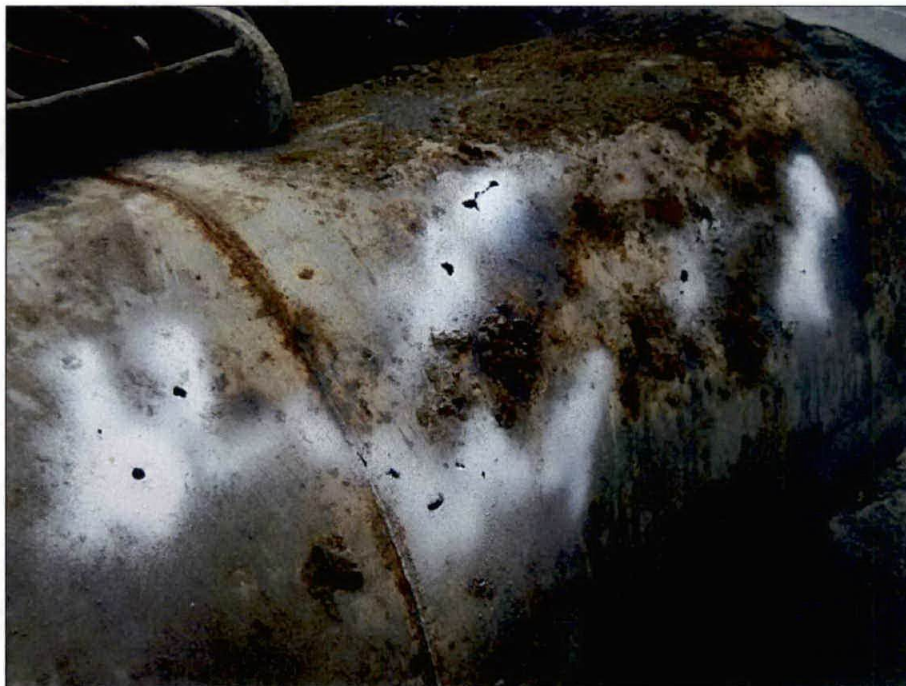
Photograph 8: UST3 with numerous small holes marked in white paint.
