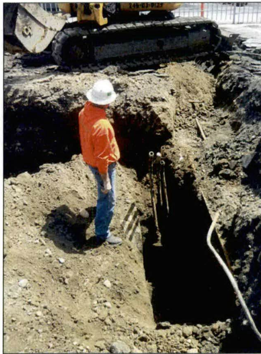
Photograph 5: One of the uncovered pressure vessels.
