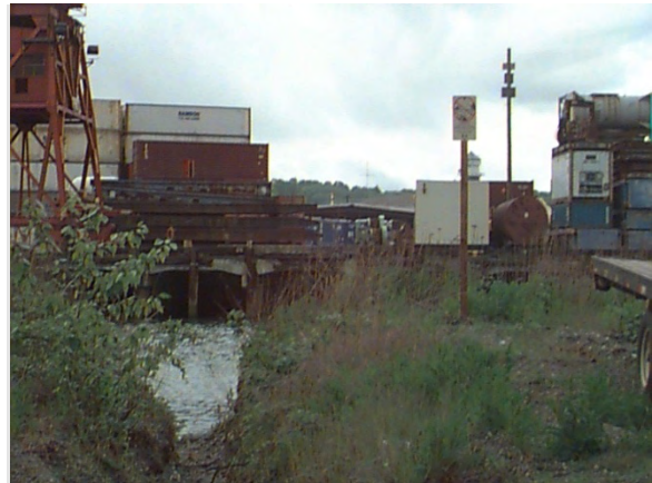
Vicinity of East Marginal Way Pump Station CSO; Looking North Across Slip 4
