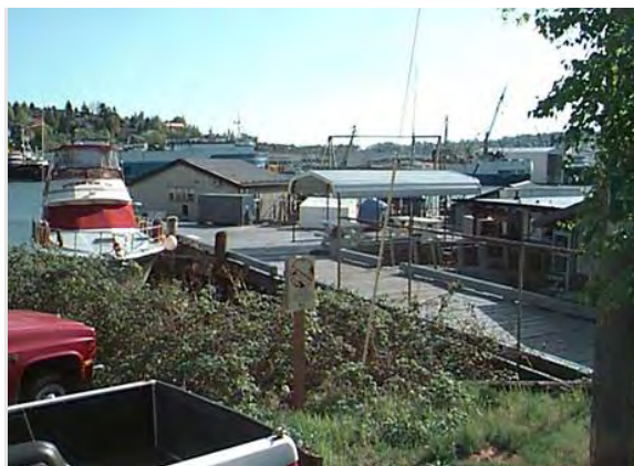
11th Avenue NW CSO Vicinity; Looking South Across Ship Canal
