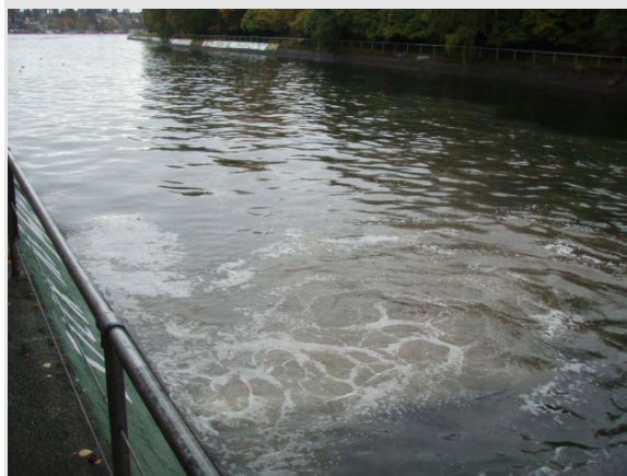
Montlake CSO Overflowing 10/26/09
