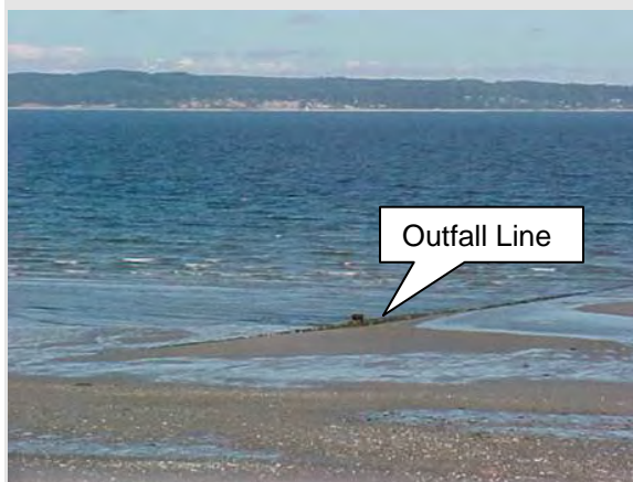
North Beach CSO Wetwell Overflow Outfall; Looking West Across Puget Sound
