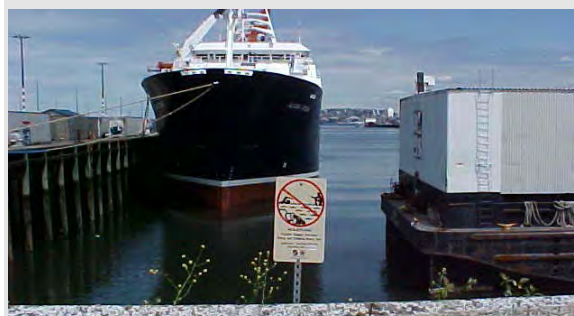
Vicinity of Harbor Avenue Regulator CSO; Looking Northeast Across West Waterway
