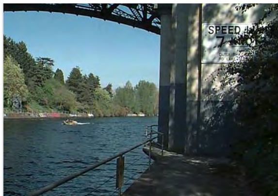
Montlake CSO Vicinity Looking East
