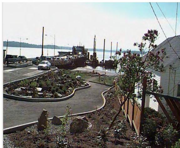
Barton Street Pump Station CSO Vicinity; Looking West Across Puget Sound.
