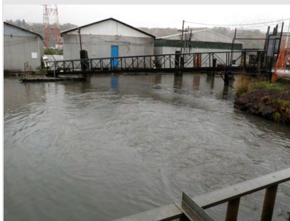
Michigan Regulator CSO Overflowing 10/26/09
