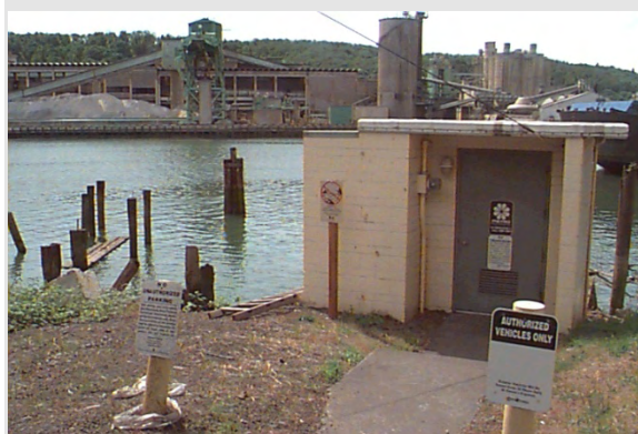
Brandon Regulator CSO Vicinity; Looking West Across Duwamish River
