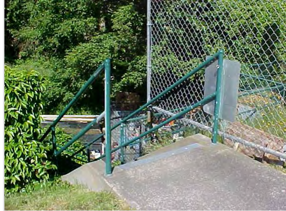
30th Avenue NE and Belvoir Place Pump Stations CSO Vicinity; Looking Southwest, No Warning Signage Because No Public Access
