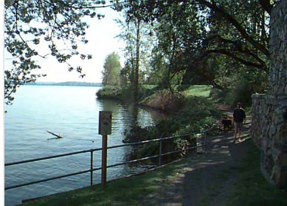
East Pine Street Pump Station Vicinity; Looking Southeast Over Lake Washington
