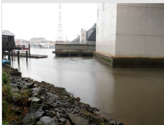
West Michigan Regulator CSO Overflowing 10/17/2009
