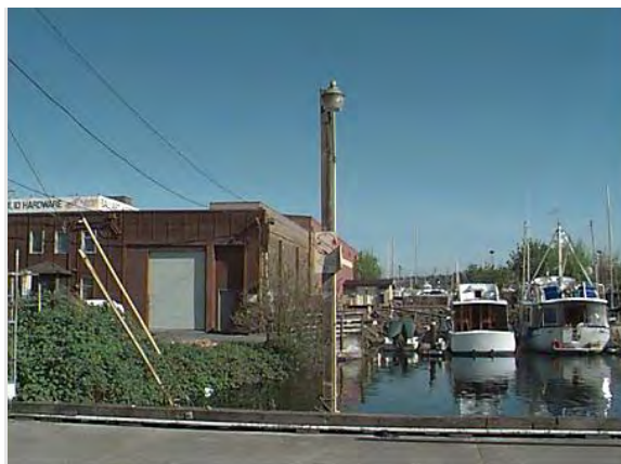
Ballard Siphon Regulator CSO Vicinity; Looking South Across Ship Canal
