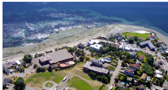
Alki CSO Treatment Plant Vicinity; Aerial, Looking West into Puget Sound
