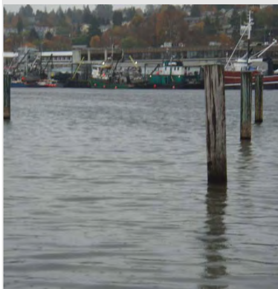
11th Avenue NW CSO Overflowing 10/26/09
