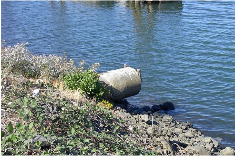
Photo 100-0842 – Looking NE at outfall T115_01.
