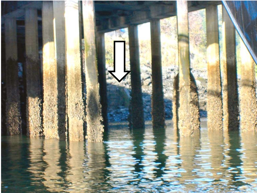
Photo 100-0932 – Looking west at outfall T115_07, a 36" concrete pipe.
