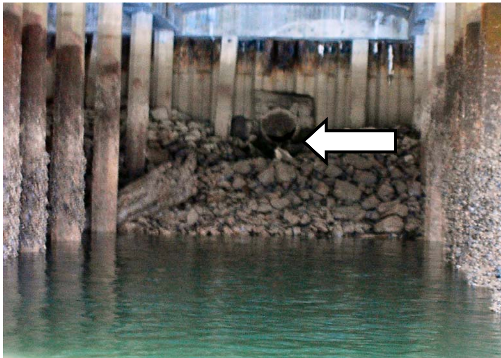
Photo 100-0935 – Looking west at outfall T115_06, a 24" concrete pipe.
