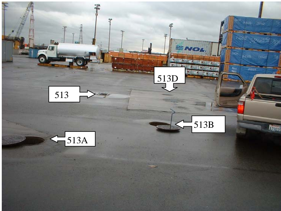
Photo 100-0030 – Looking S at MH 513, MH 513B, CB 513 and Oil Water Separator 513D. .
