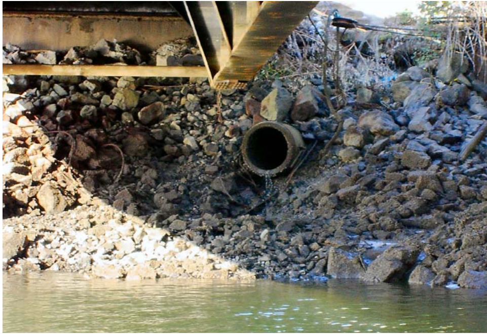
Photo 100-0936 – Looking west at outfall T115_05. This outfall is a 30” concrete pipe.
