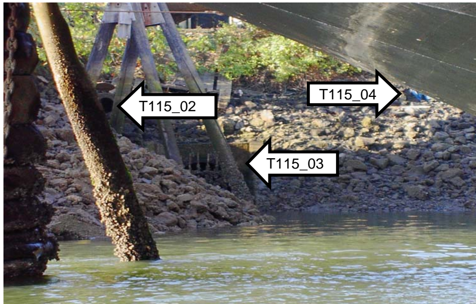
Photo 100-0938 – Looking west at outfall T115_03, a 32" concrete outfall. Outfall T115_02 an 18" concrete pipe, shown on the left side of the photo. Outfall T115_04, a 12" composite pipe, is just out of view on the right side of photo. The edge of the ship on the right side of photo is also in photo100-0937.
