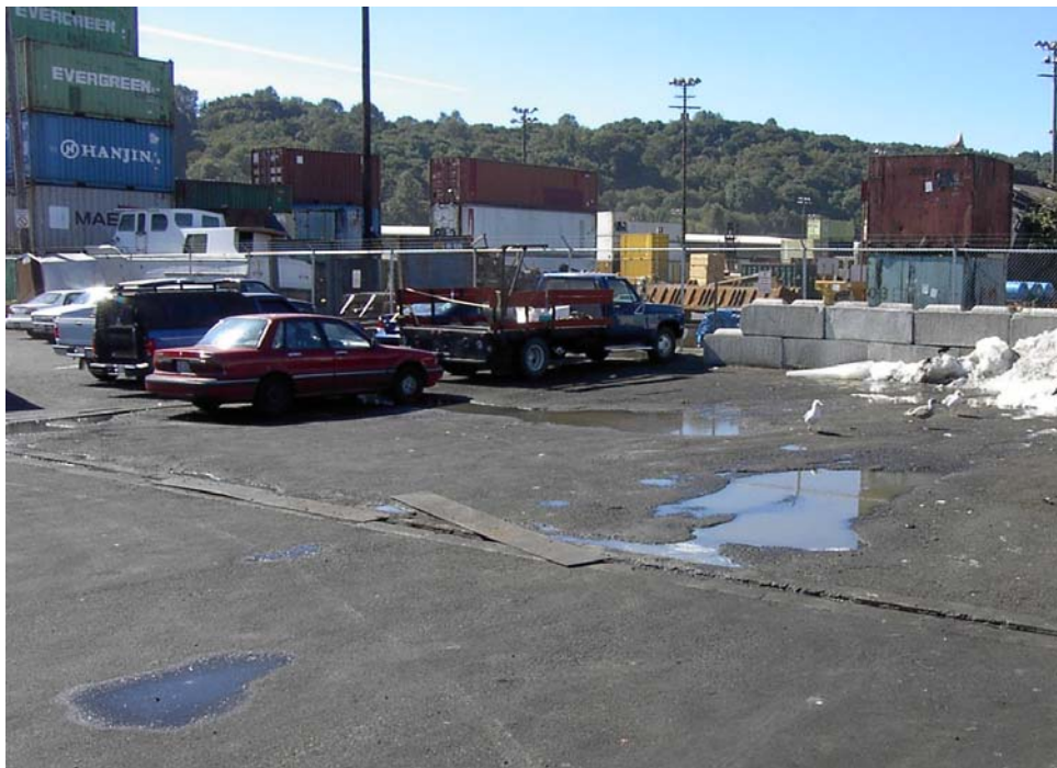
Photo 100-0842 – Looking NW at trench drain 637A.
