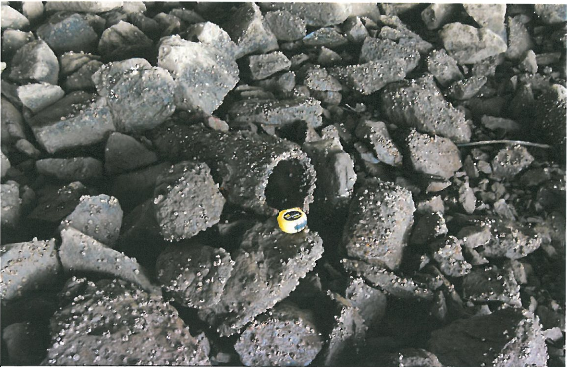
June 14, 2007 - Photo DSC-0101 Looking west at outfall # T18_Outfall_20.
