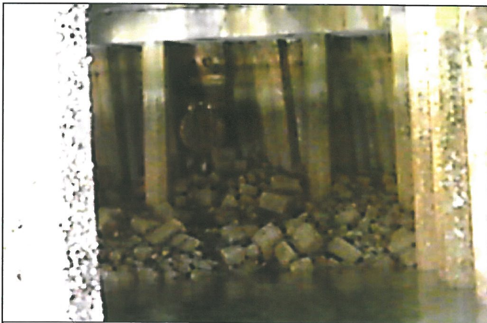
October 4, 2006 – Photo 100-0044 Looking west at outfall # T5_Outfall_13.
