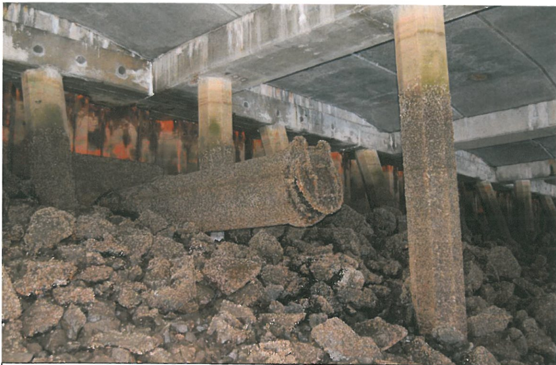
June 13, 2007 - Photo DSC-0021 Looking southeast at outfall # T25_Outfall_01.
