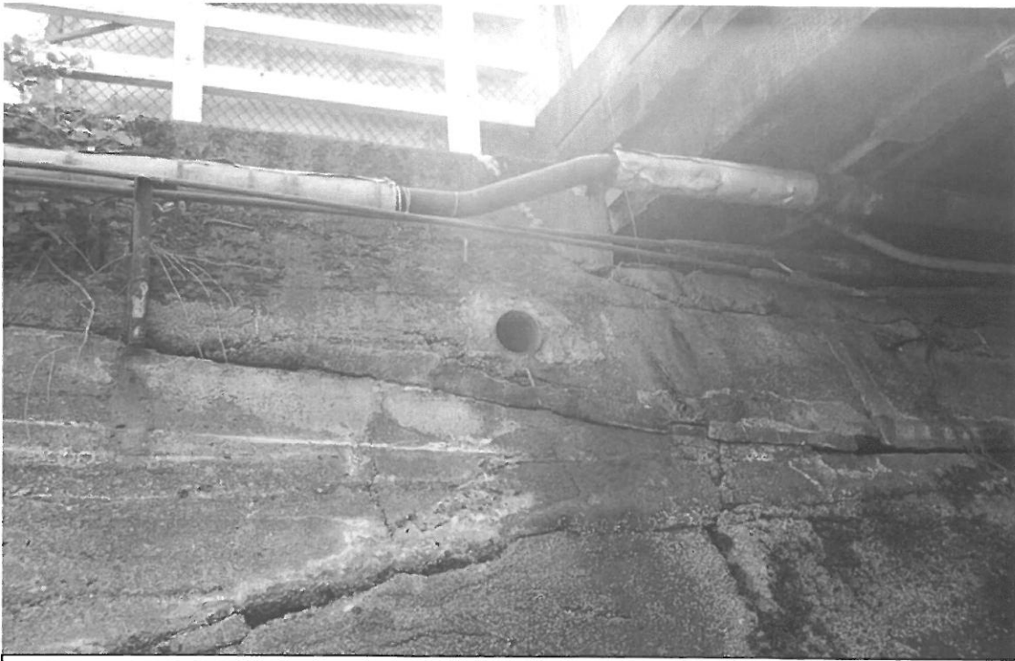
June 13, 2007 - Photo DSC-0061 Looking east at outfall # P48_Outfall_02.
