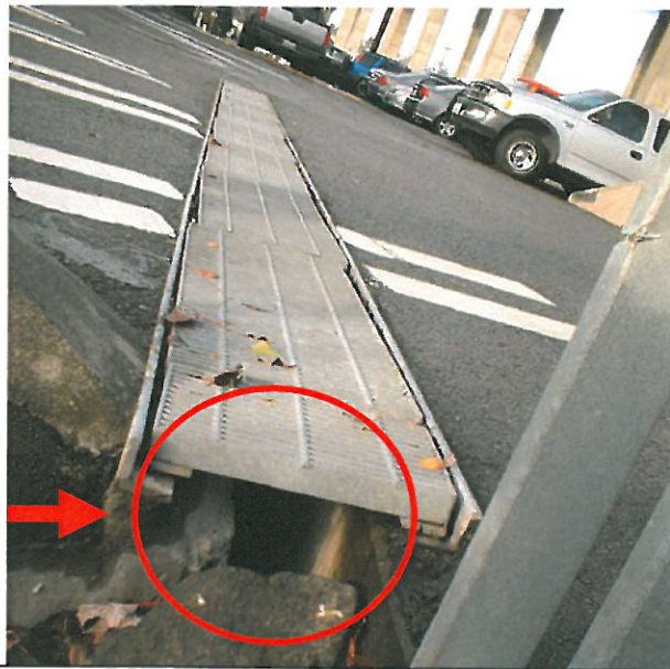
November 10, 2006 - Photo 100-0002 Looking west at trench drain and outfall # T102_Outfall_01.
