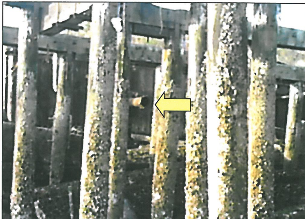
October 4, 2006 – Photo 100-0023 Looking south at outfall # T5_Outfall_02.
