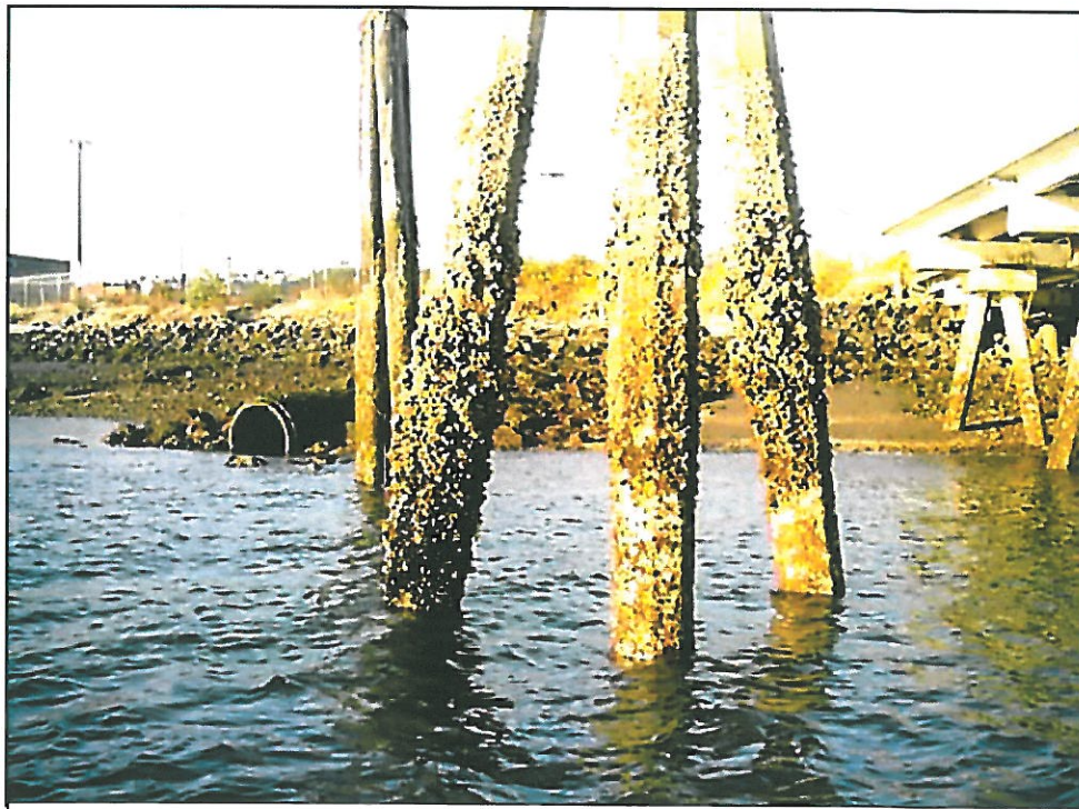
October 4, 2006 – Photo 100-0029 Looking west at outfall # T5_Outfall_06.
