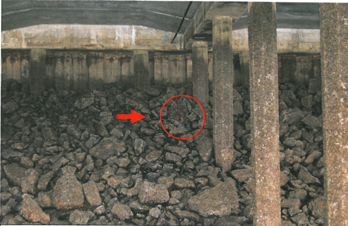
June 14, 2007 - Photo DSC-0020 Looking west at outfall # T18_Outfall_13.
