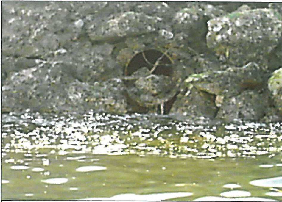
October 4, 2006 – Photo 100-0020 Looking south at outfall # T5_Outfall_03.
