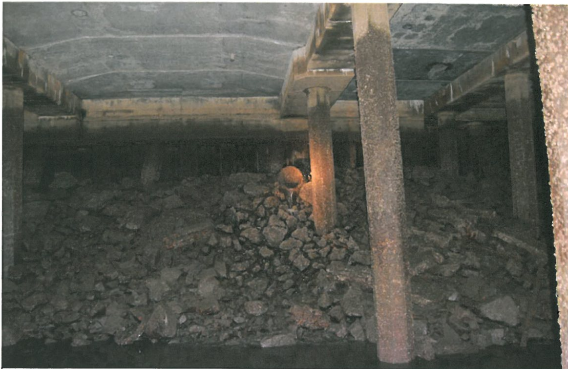
June 14, 2007 - Photo DSC-0010 Looking west at outfall # T18_Outfall_16.
