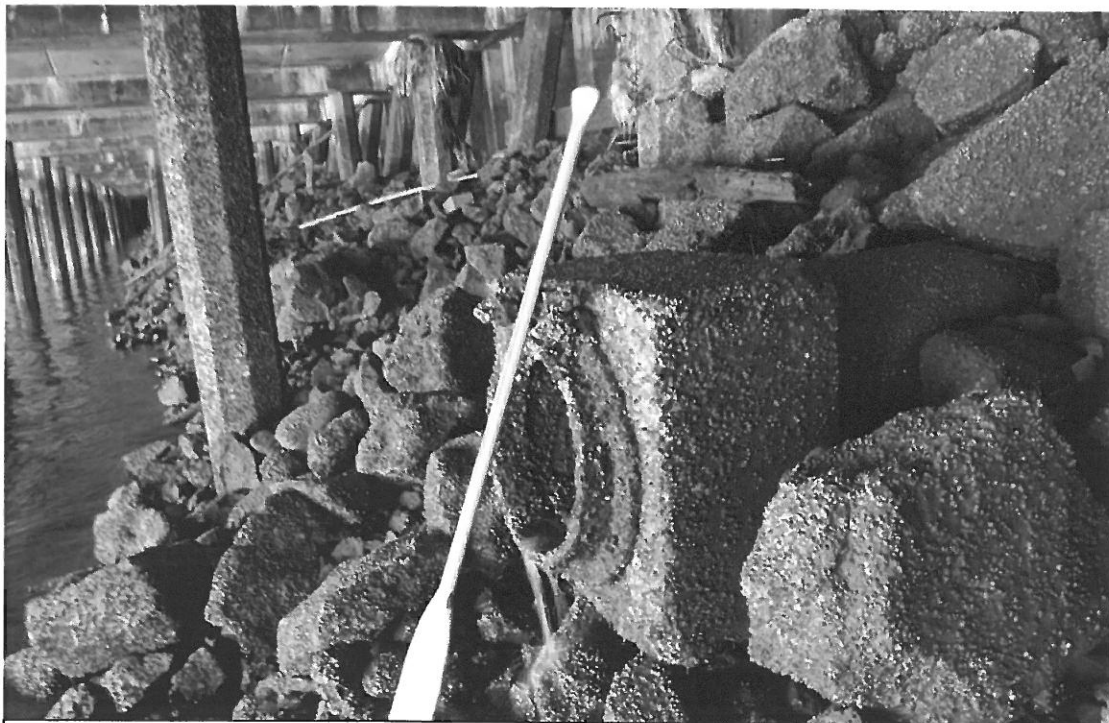
June 13, 2007 - Photo DSC-0087 Looking southwest at outfall # T18_Outfall_10.
