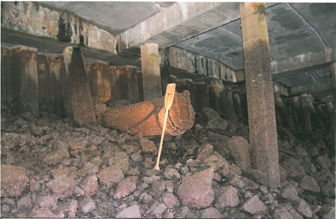
June 13, 2007 - Photo DSC-0017 Looking southeast at outfall # T25_Outfall_03.
