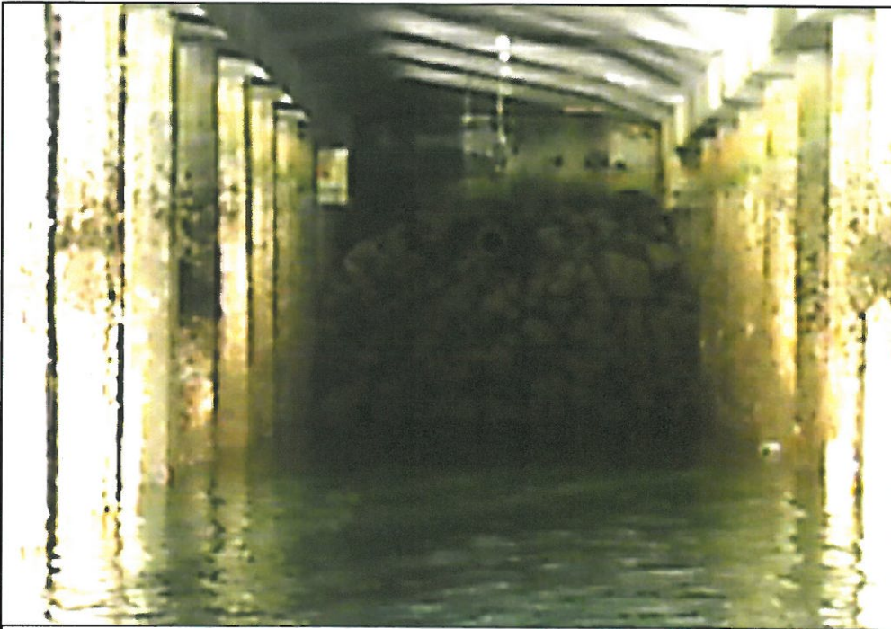
October 4, 2006 – Photo 100-0032 Looking west at outfall # T5_Outfall_07.
