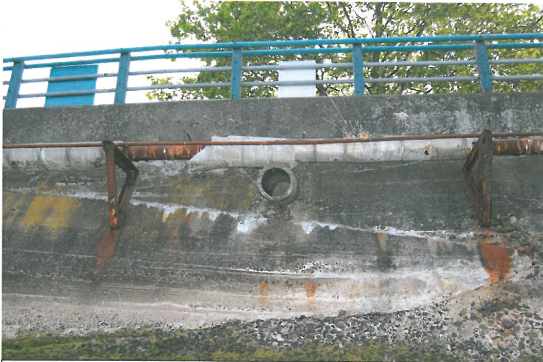
June 13, 2007 - Photo DSC-0065 Looking east at outfall # Alaska Square Park_Outfall_01.
