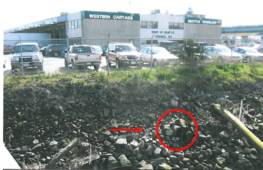
April 3, 2007 - Photo 100-0292 Looking east at outfall # T104_Outfall_01.
