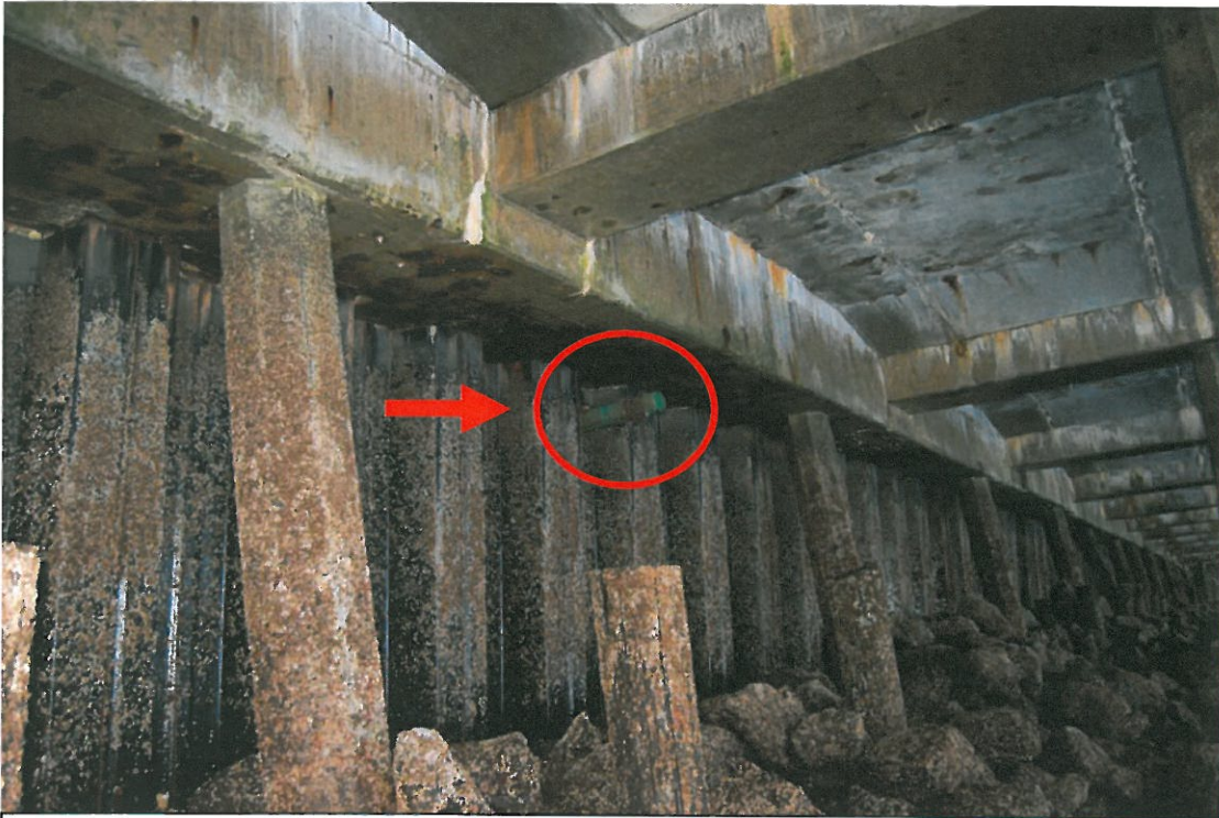
June 13, 2007 - Photo DSC-0054 Looking southeast at outfall # T46_Outfall_04.
