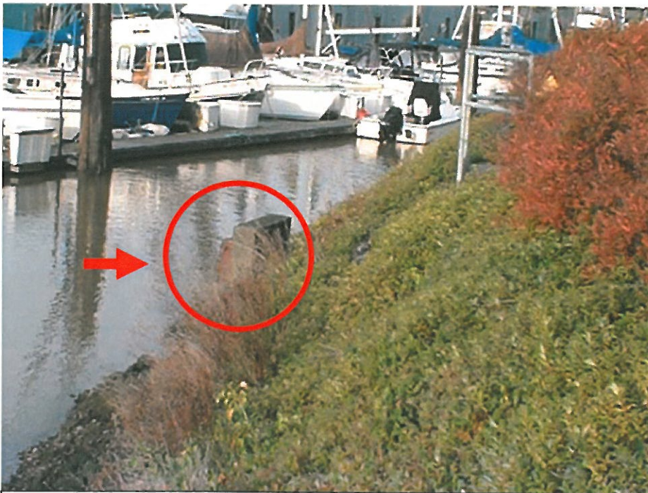
November 10, 2006 - Photo 100-0005 Looking west at outfall # T102_Outfall_04.
