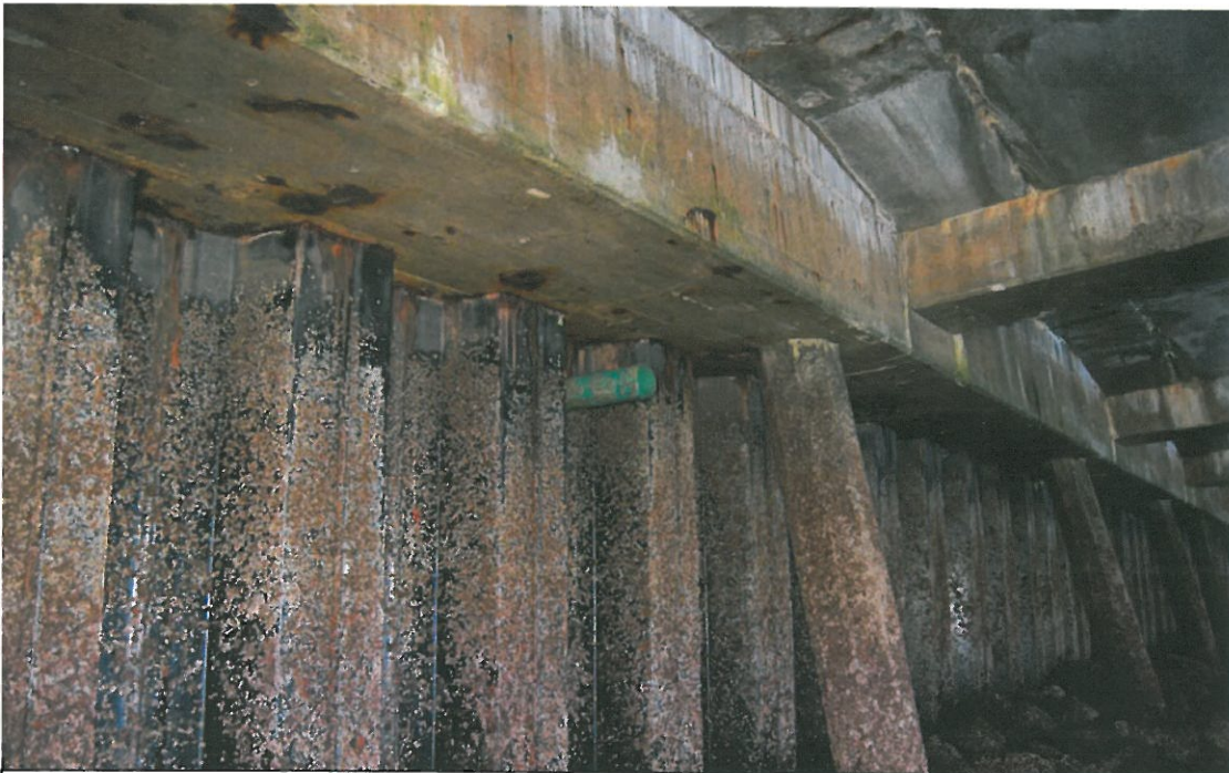
June 13, 2007 - Photo DSC-0052 Looking southeast at outfall # T46_Outfall_03.
