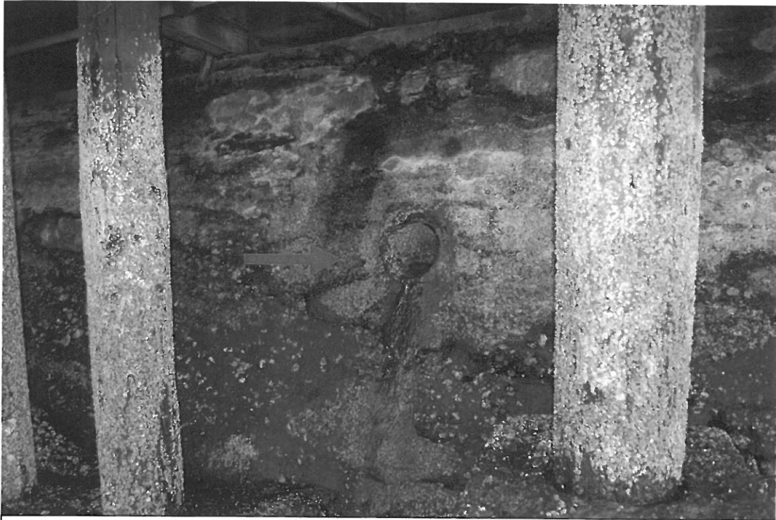
June 13, 2007 - Photo DSC-0055 Looking east at outfall # P48_Outfall_04.
