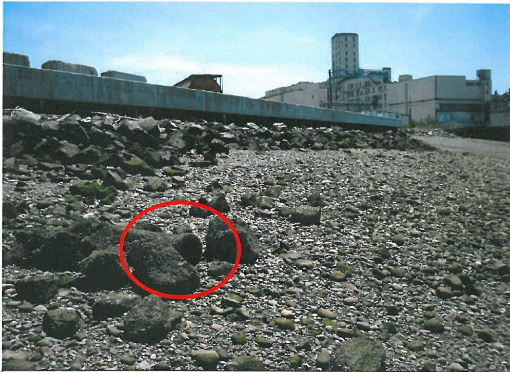
June 14, 2007 – Photo DCS –0038 Looking south at outfall # T10_Outfall_01.
