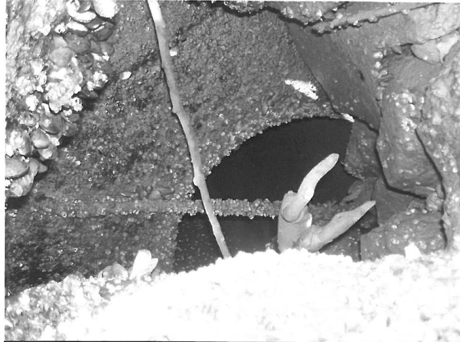
June 20, 2007 - Photo DSCF-0653 Looking east at outfall # T106_Outfall_01.
