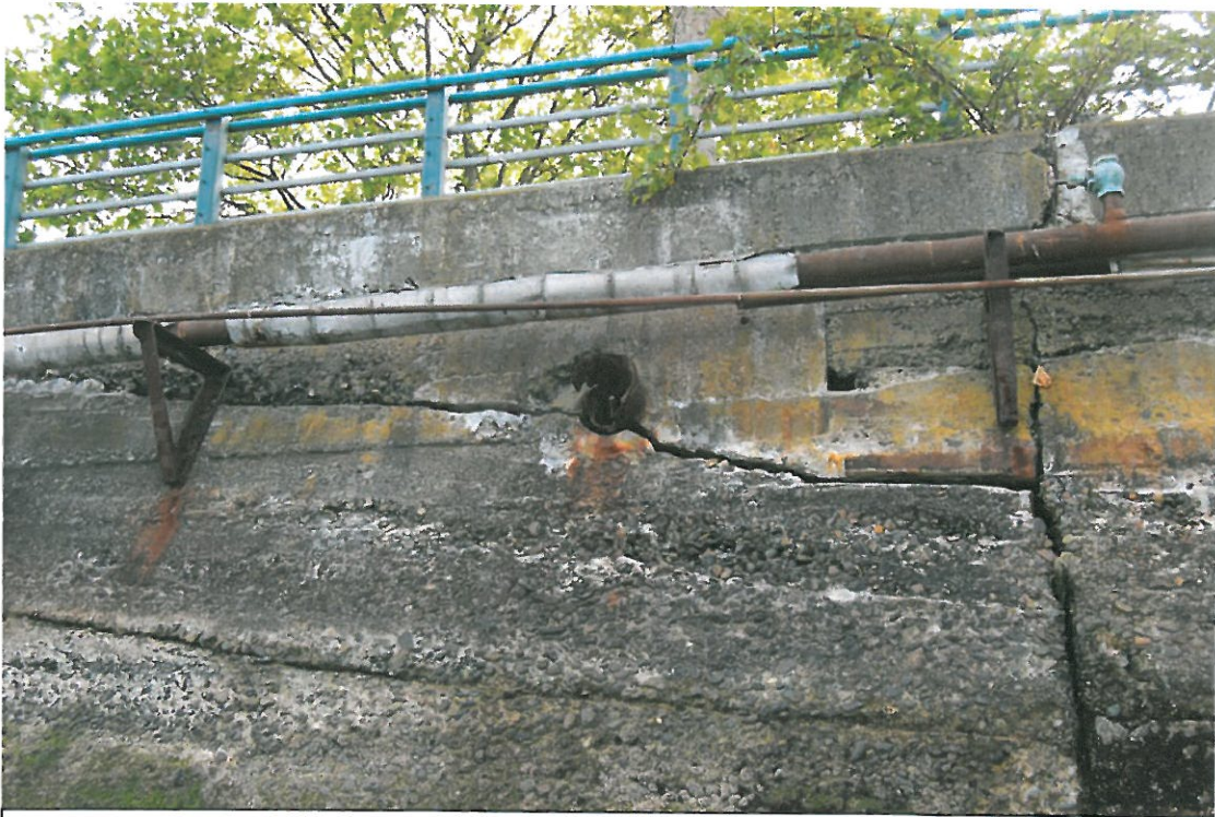
June 13, 2007 - Photo DSC-0064 Looking east at outfall # Alaska Square Park_Outfall_02.
