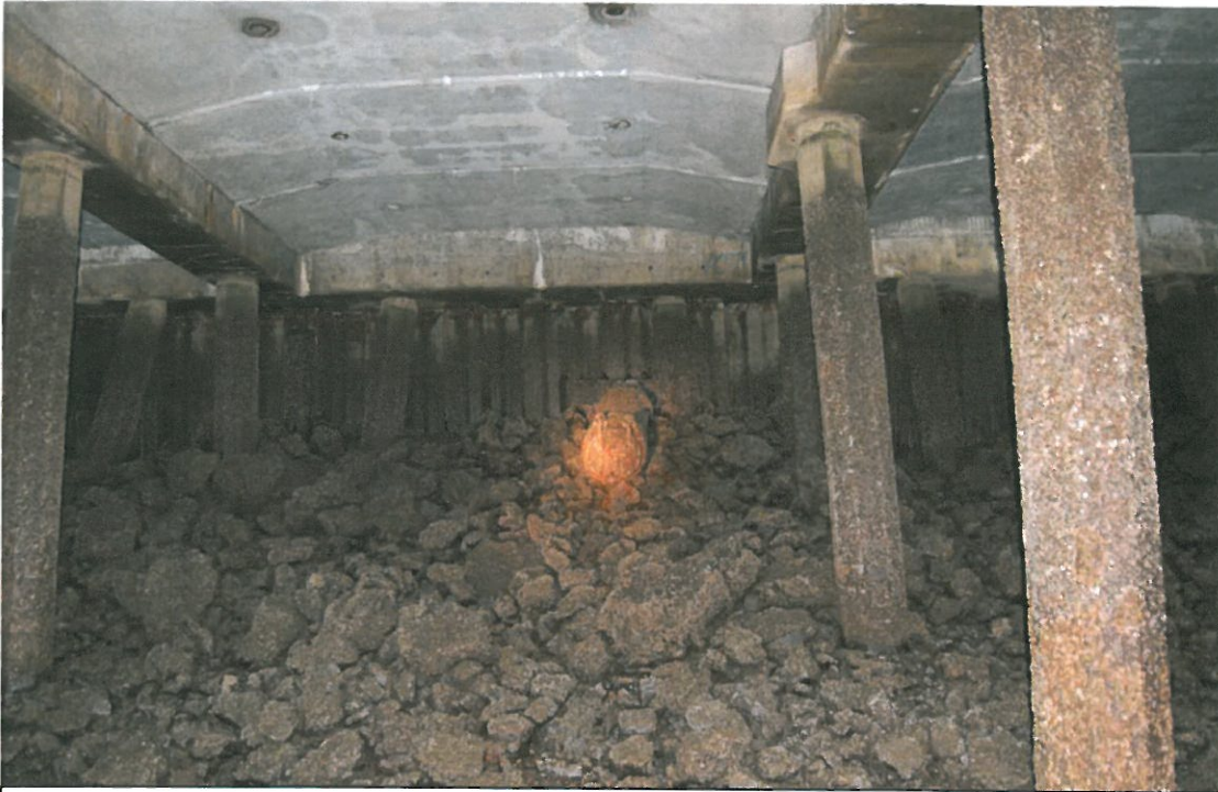
June 14, 2007 - Photo DSC-0012 Looking west at outfall # T18_Outfall_15.
