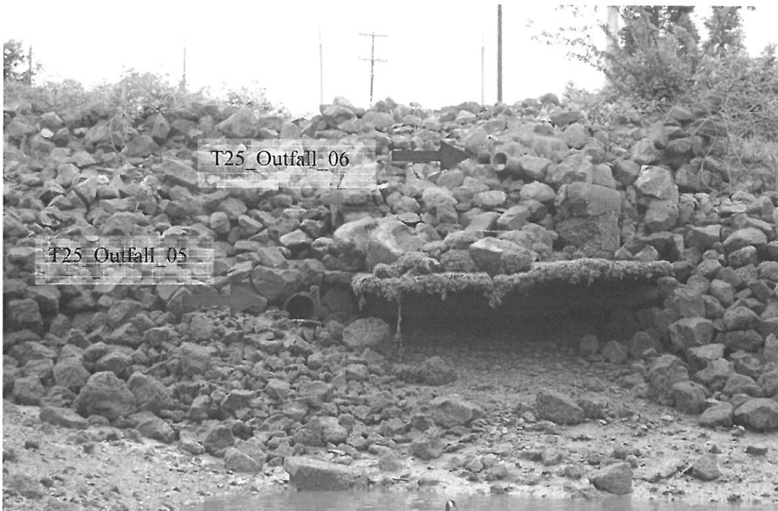
June 13, 2007 - Photo DSC-0013 Looking east at outfalls # T25_Outfall_05 and T25_Outfall_06.
