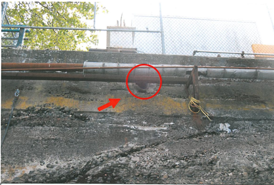
June 13, 2007 - Photo DSC-0063 Looking east at outfall # P48_Outfall_01.
