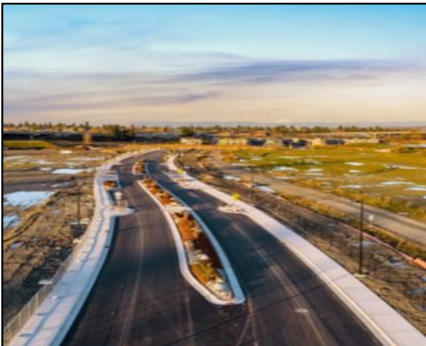
North view in the Everett Tire Fire Site
