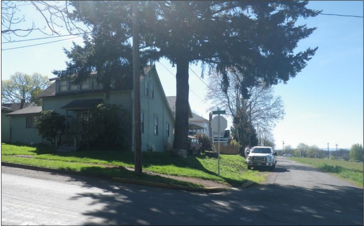
Figure 4. Overview of project area facing south, from the intersection of Railroad Avenue and Ash Street.
