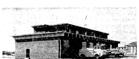
Fire and crash station went into service last month.
