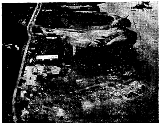
The same area early in construction period
