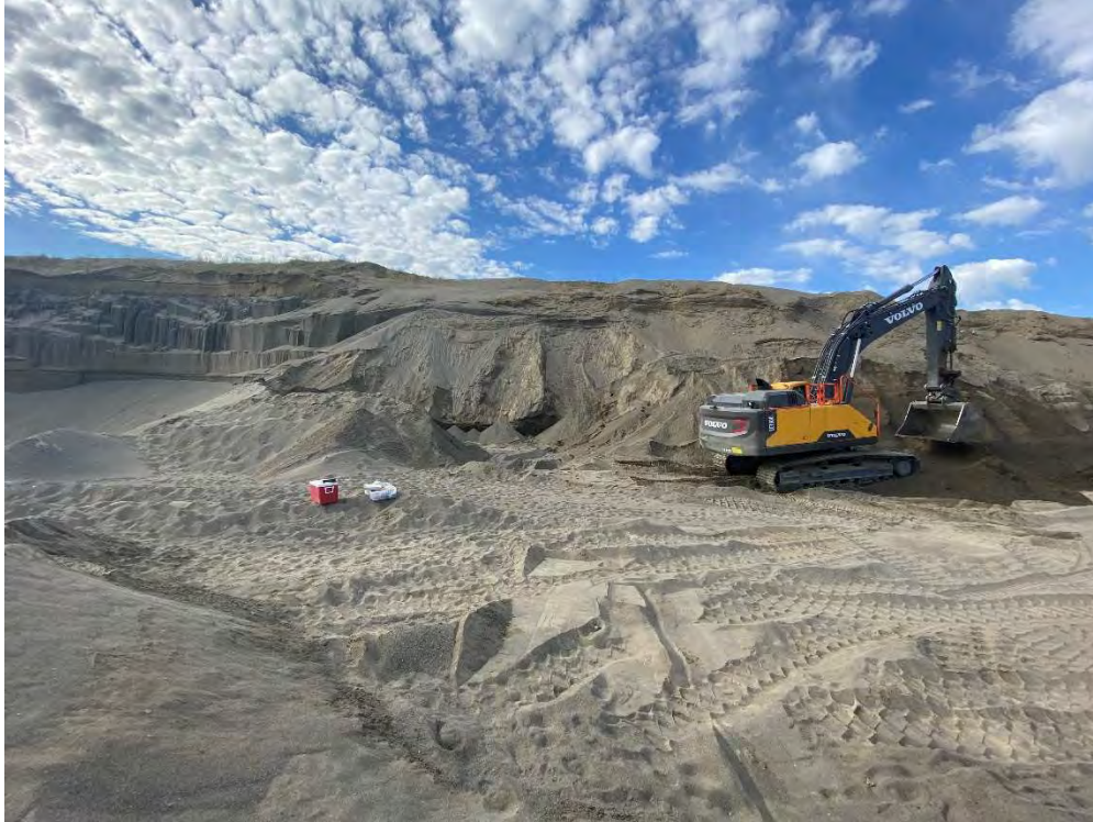
Photo shows contaminated soil being removed. Photo was taken looking in a southerly direction.
