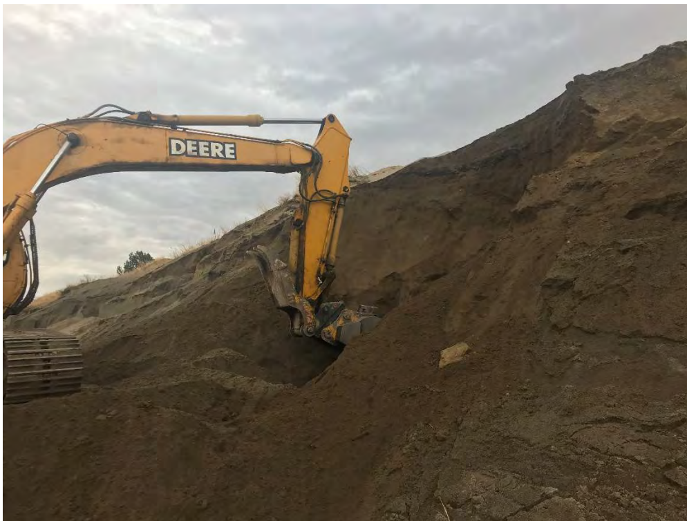
Photo shows test pit being dug into the slope to the south of where contamination was discovered. Photo was taken looking in a southeasterly direction.
