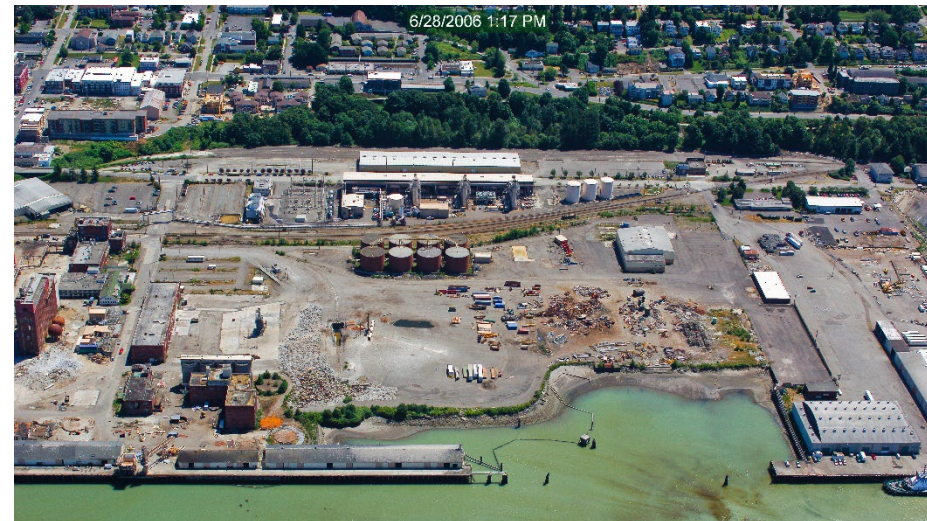
GP West Site, Chlor-Alkali Area facing southeast, June 2006.
