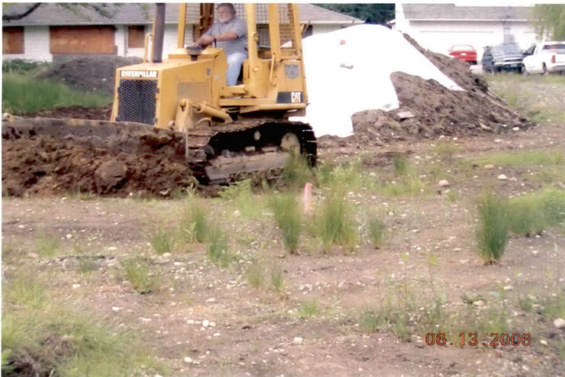
Photo 8 Excavating Soil South of House, View North 6/13/2006
