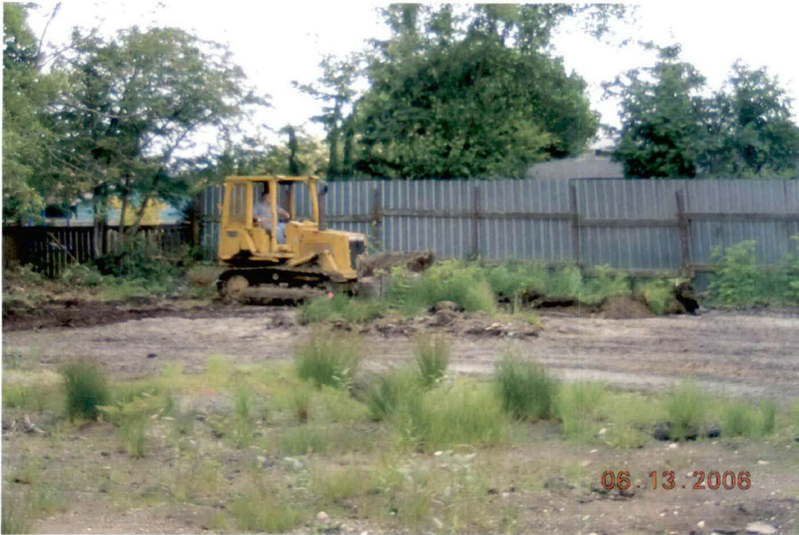
Photo 7 Excavating Soil Along South Fence, View South 6/13/2006
