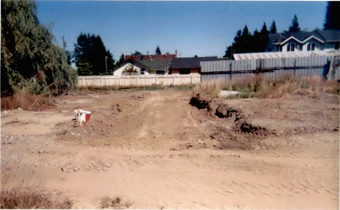
Photo 13 View East, Northern Excavation from near House 7/26/2006
