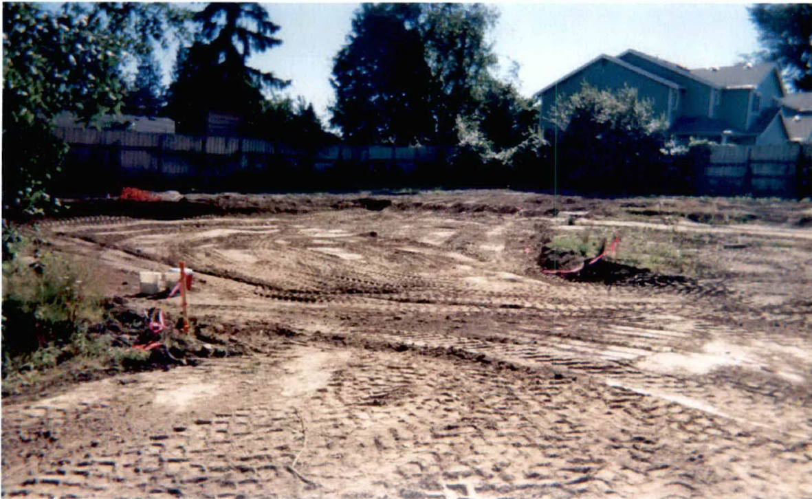
Photo 16 View SW, Southern Excavation from East Fence 7/26/2006
