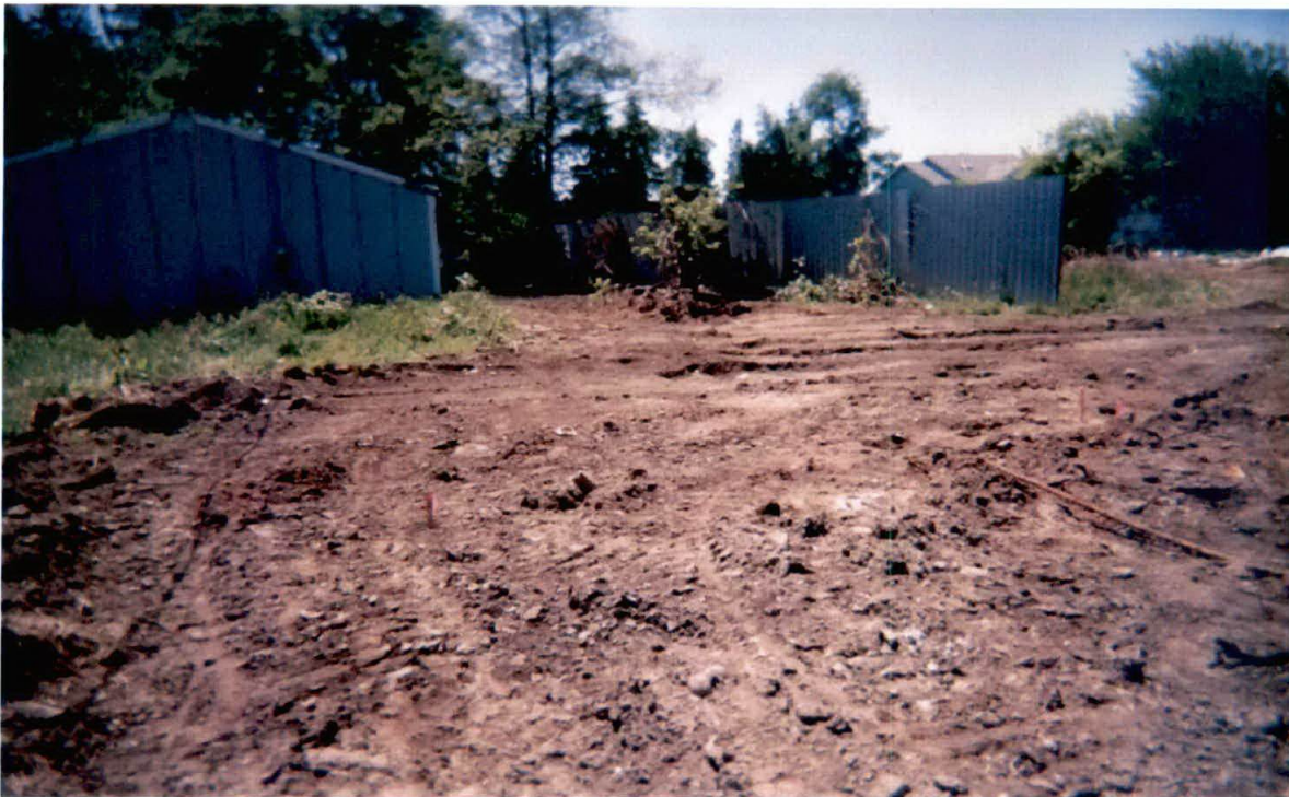
Photo 10 View South at Garage/Shop, Soil Piles Removed 6/24/2006
