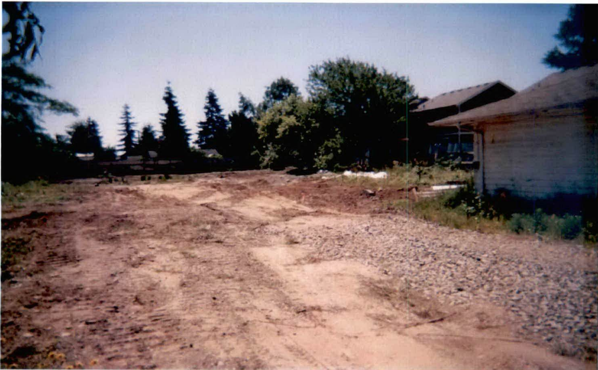
Photo 9 View South from House, All Soil Piles Removed 6/24/2006
