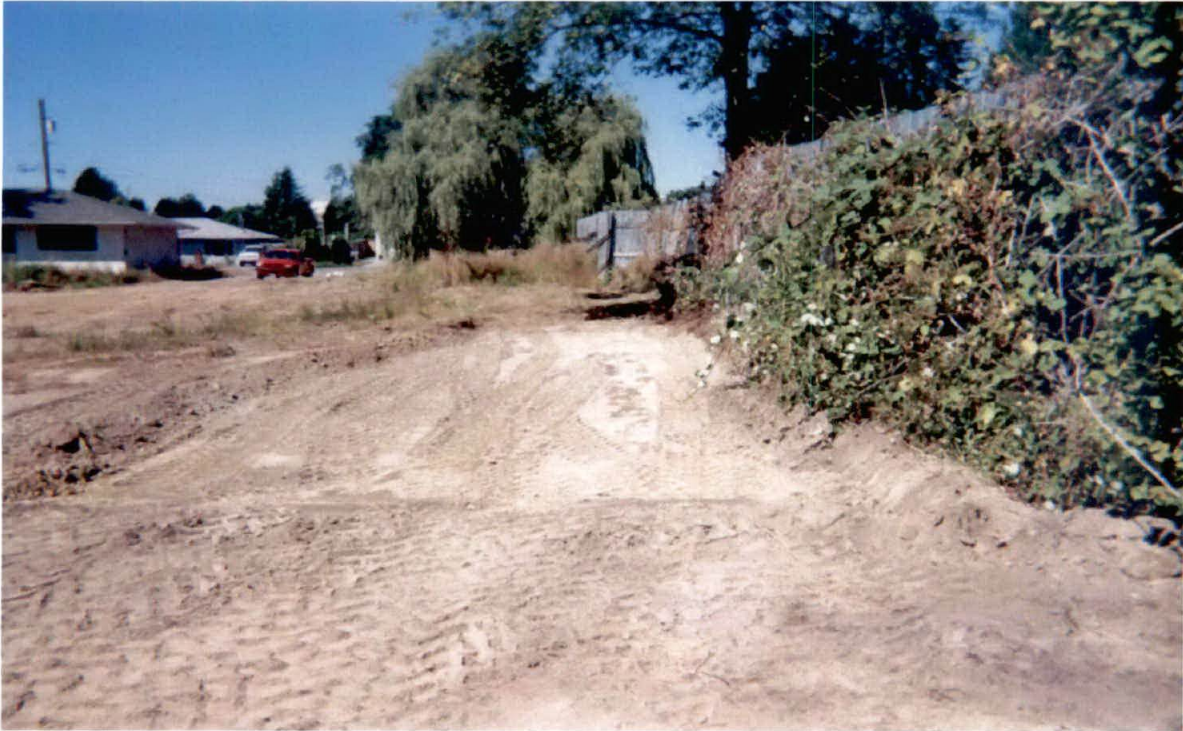
Photo 15 View North of Central Excavation, East Fence 7/26/2006
