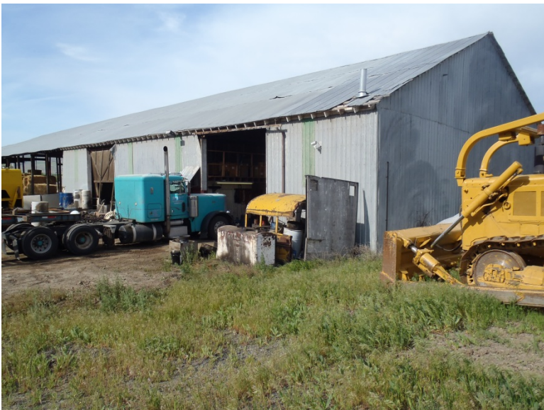
Area east of mechanical shop structure.
