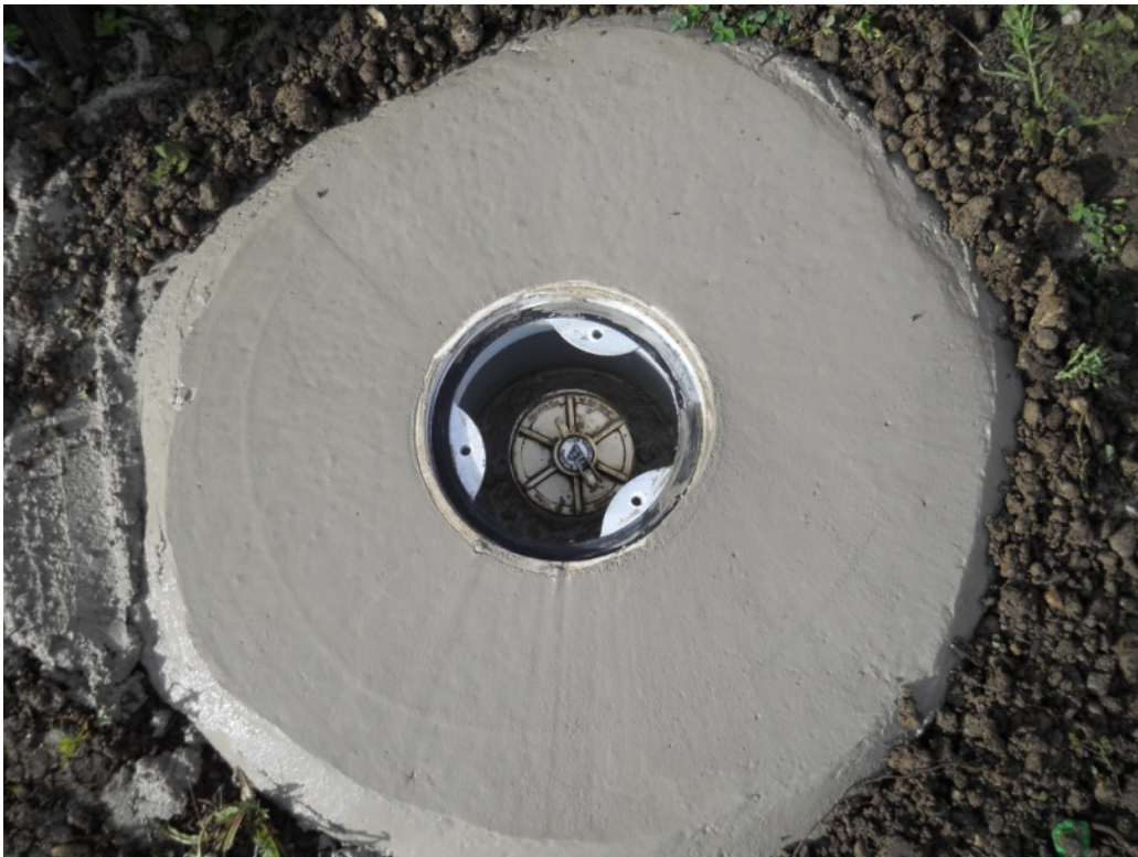
Photograph 2. Condition of well RW-2 after repair.
