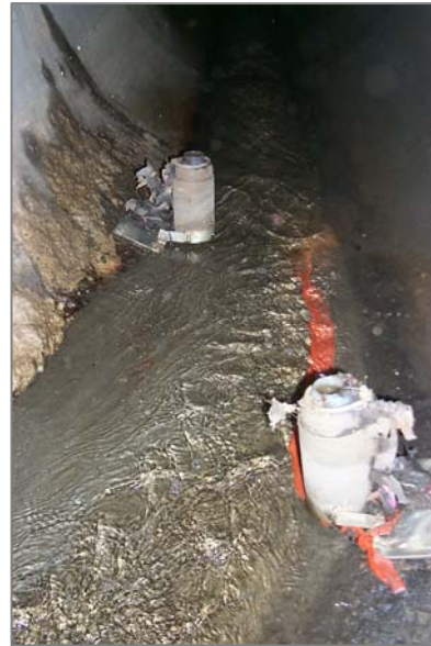
Figure 2: Typical sediment trap installation.
