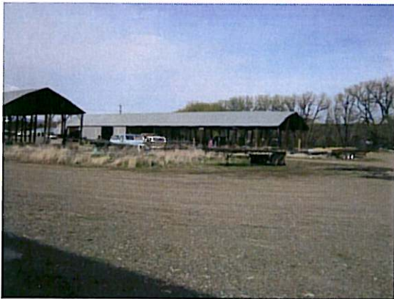
Overview of barn showing open hay storage at south end 2012
