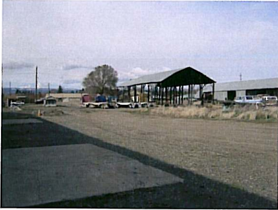
Hay storage shed facing north with diesel garage/barn in background 2012
