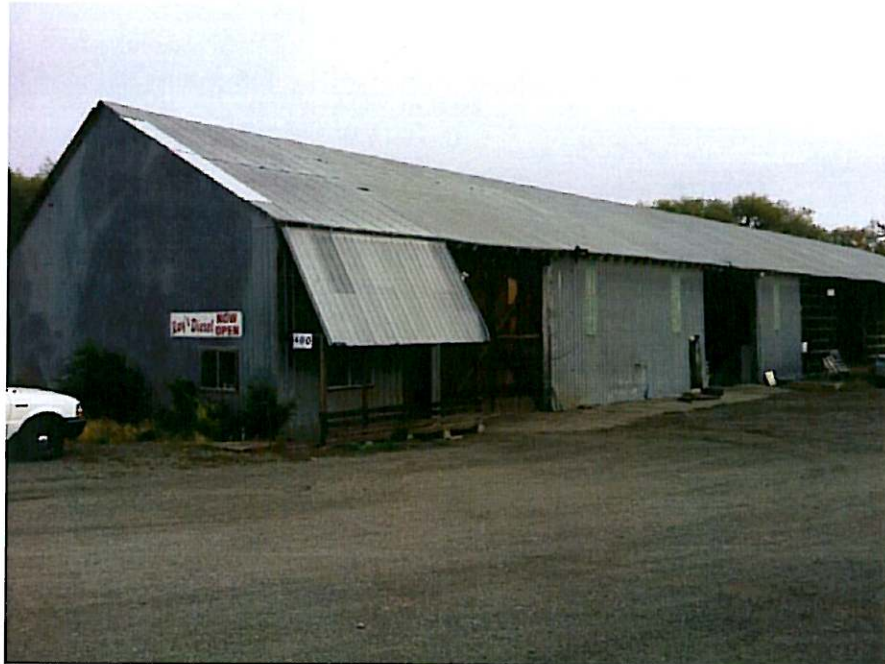
Figure 8. View of the west elevation of this barn and diesel repair shop located east of scale house/residence.
