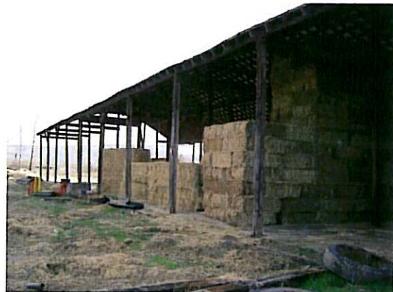
West elevation of barn showing hay storage area 2012
