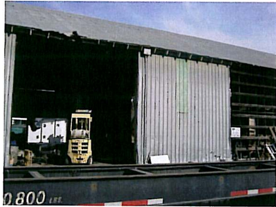
East side of barn showing sliding doors 2012
