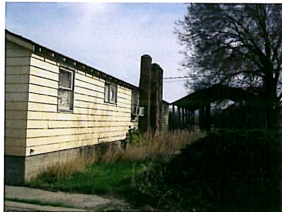
Close up of west elevation 2012
