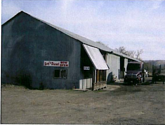
North elevation of diesel garage and barn building 2012
