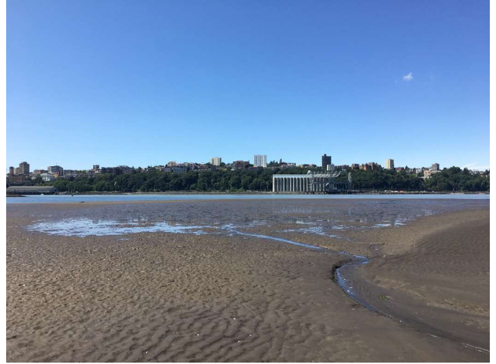
Photo 6: Eastern edge of cap at Jetty looking West toward downtown Tacoma. Natural runnel, pooling and rills apparent.
