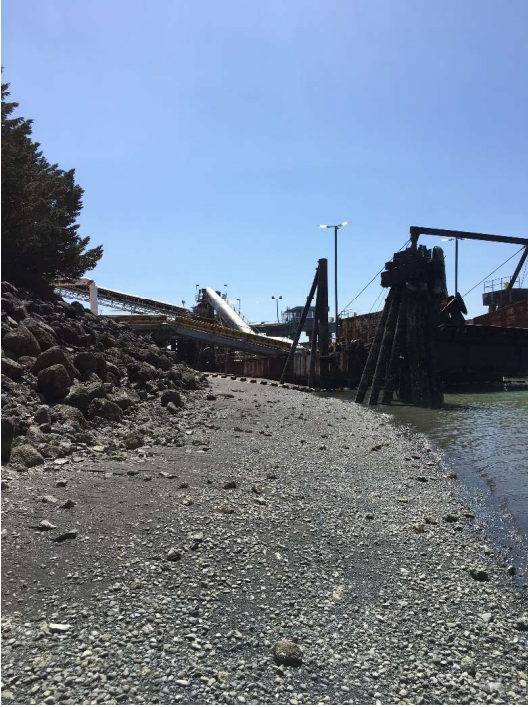
Photo 13: Western extent of cap at dolphins.
