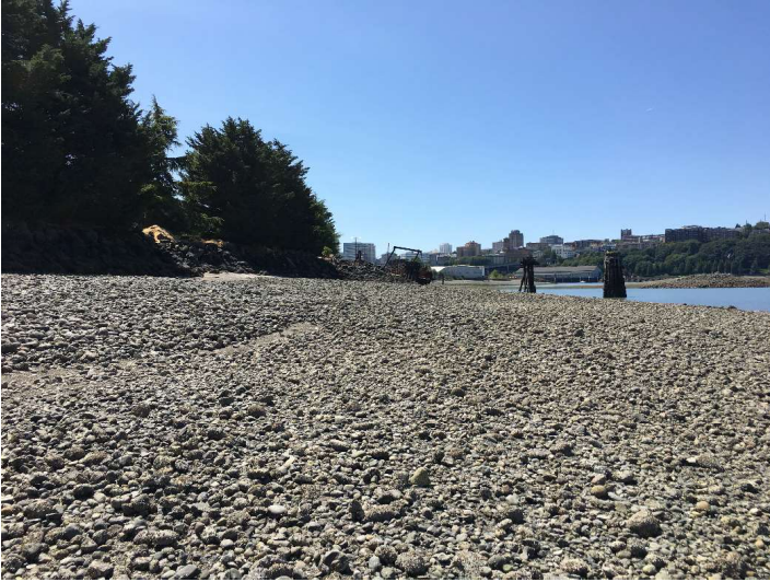
Photo 11: Looking West, western extent of cap located at dolphins. Shoreline beach is predominantly cobbles overlying finer-grained material. A sandy fine-grained material zone is apparent in the grooved area of the beach.
