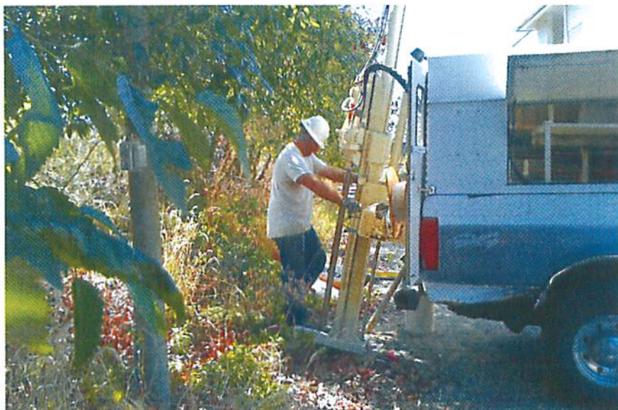
Borehole B-9 (View north)
