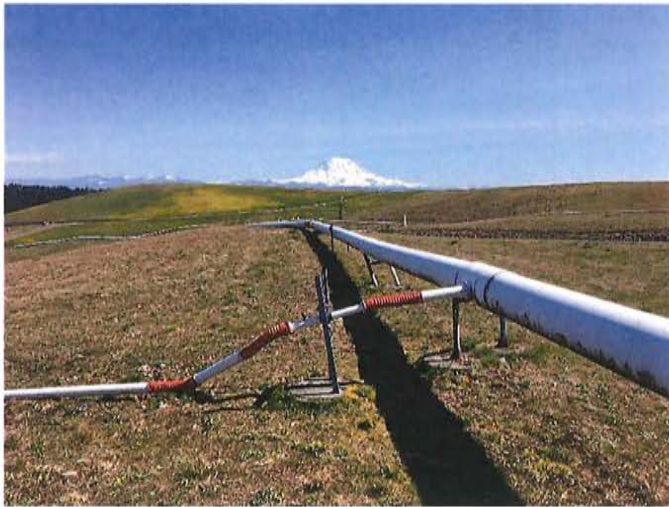
N-12 after 12"x3" Tee Replacement
