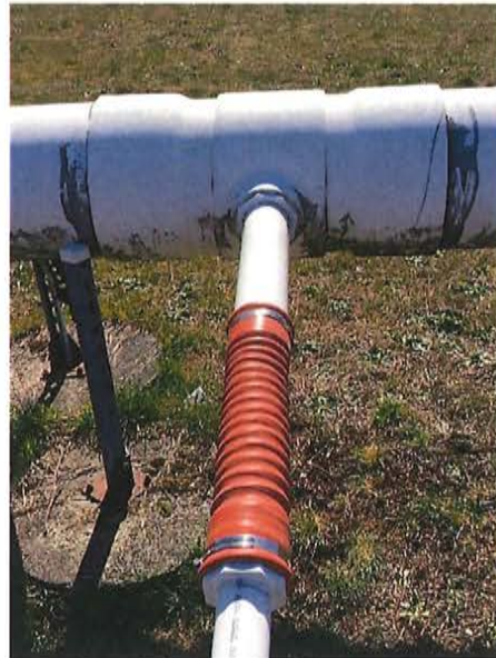
N-12 after 12"x3" Tee Replacement
