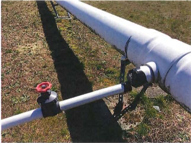
N-12 prior to 12"x3" Tee Replacement
