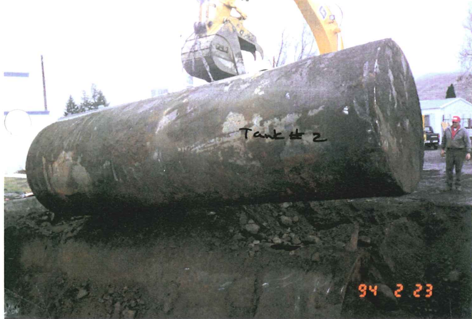
Site Photograph 4 - Removing Tank #2
