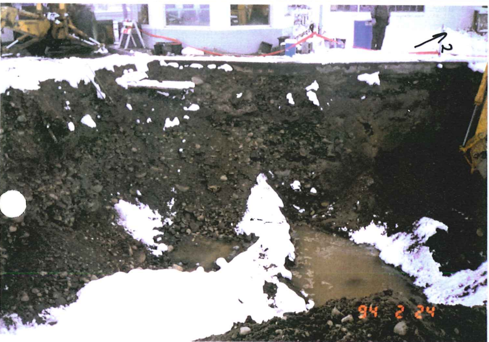
Site Photograph 5 - Excavation site looking west, shows groundwater.
