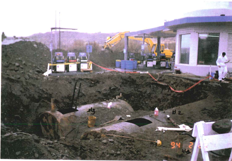
Site Photograph 2 - Looking South-West
