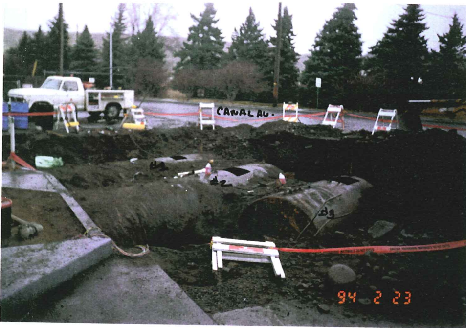
Site Photograph 1 - Looking North-East. Tanks before removal.
