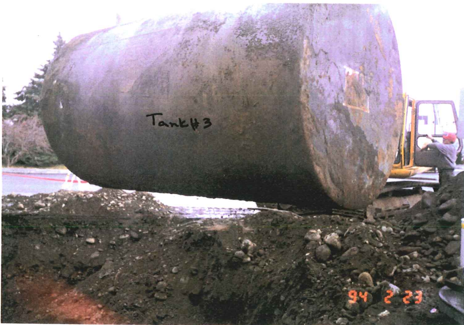
Site Photograph 3 -Removing Tank #3
