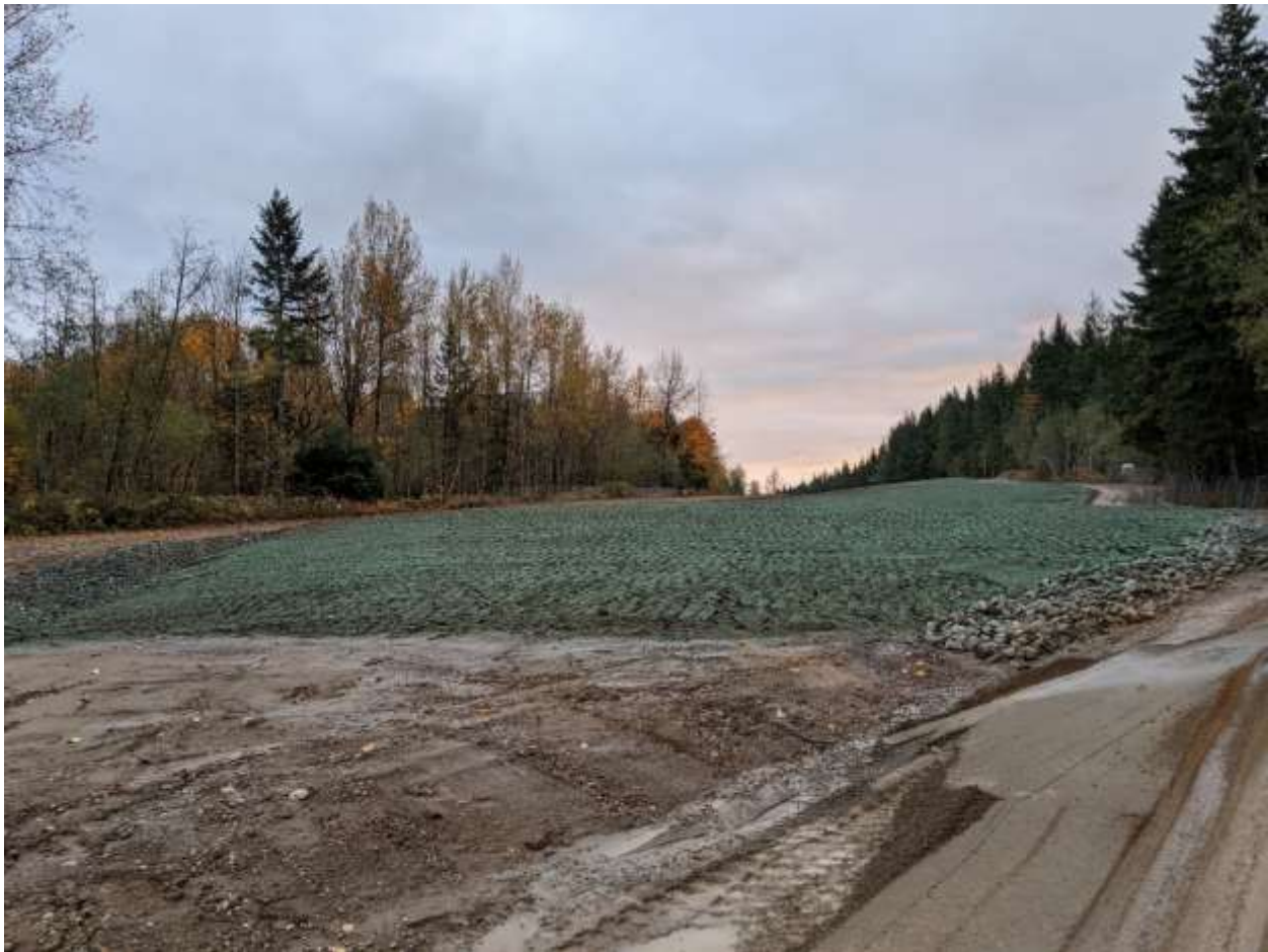
Photograph 10 – View of hydroseeding being completed at Areas 7/8.
