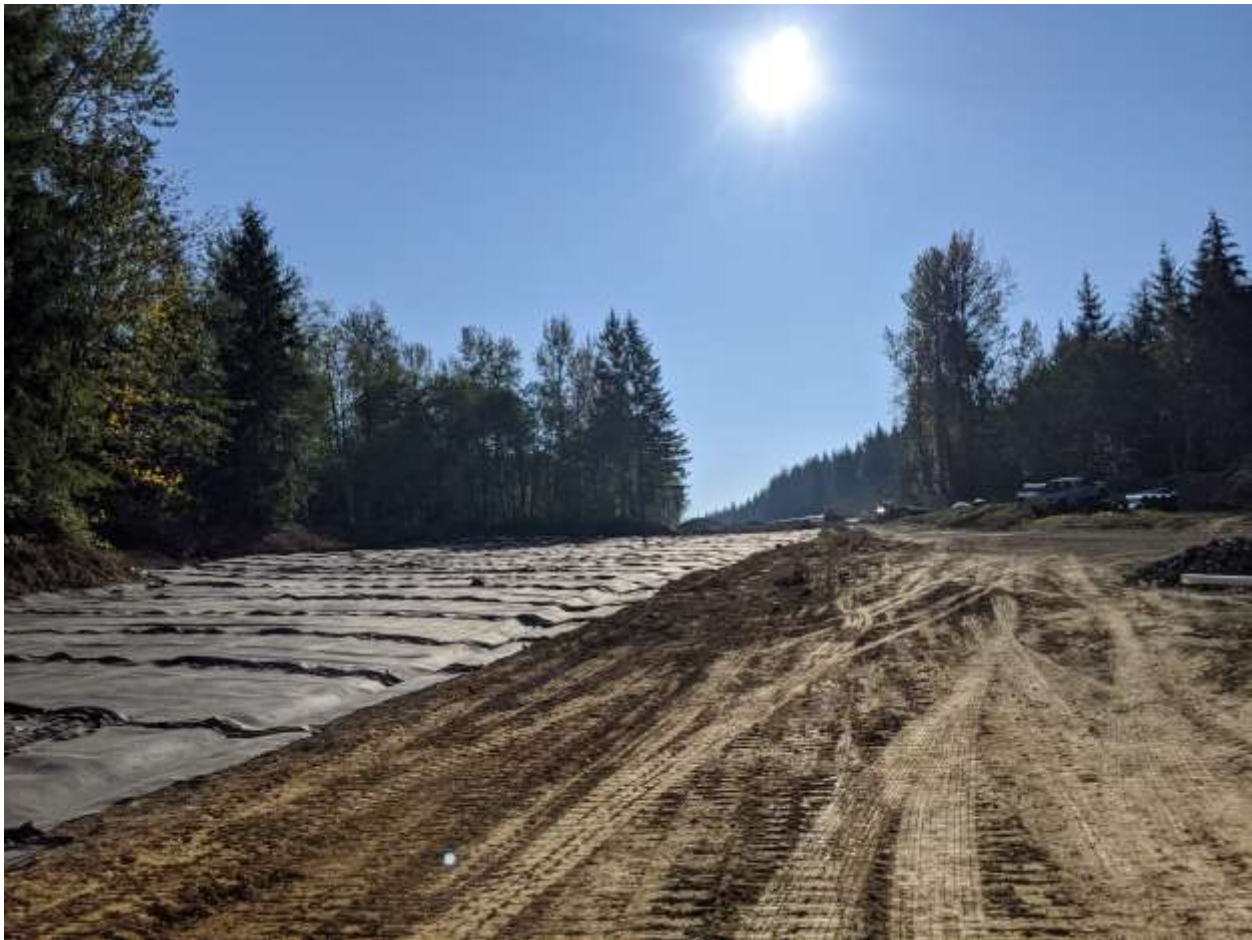
Photograph 1 – View of geomembrane and geocomposite installed at Area 9.
