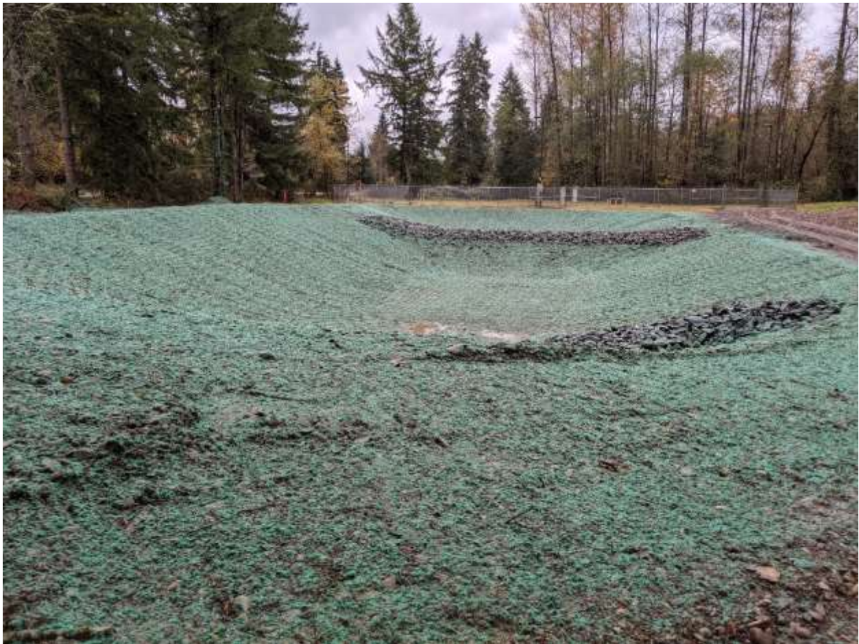
Photograph 8 – View of Infiltration Pond after hydroseeding.
