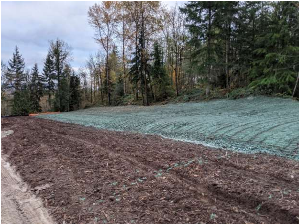
Photograph 9 – View of hydroseeding completed at Area 9.
