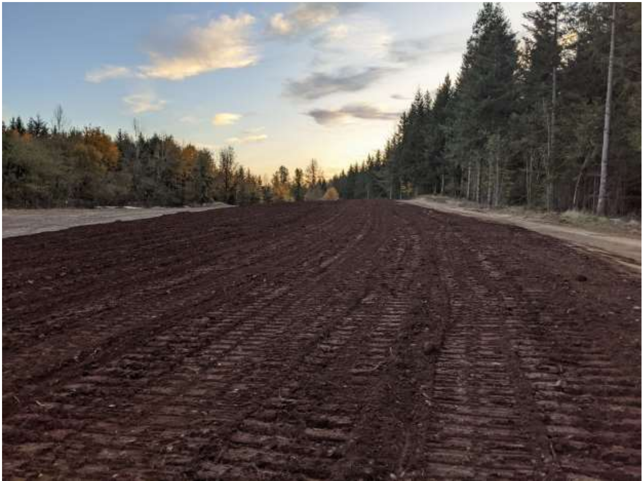
Photograph 6 – View of topsoil installed at Areas 7/8.
