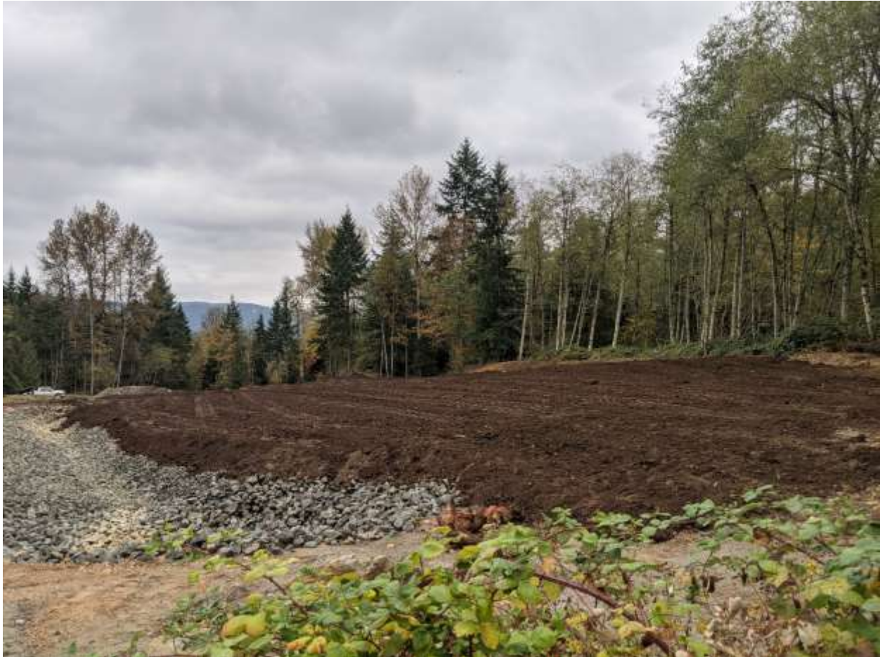
Photograph 5 – View of Area 9 with topsoil installed. Note the rock-lined ditch that is installed west of Area 9.
