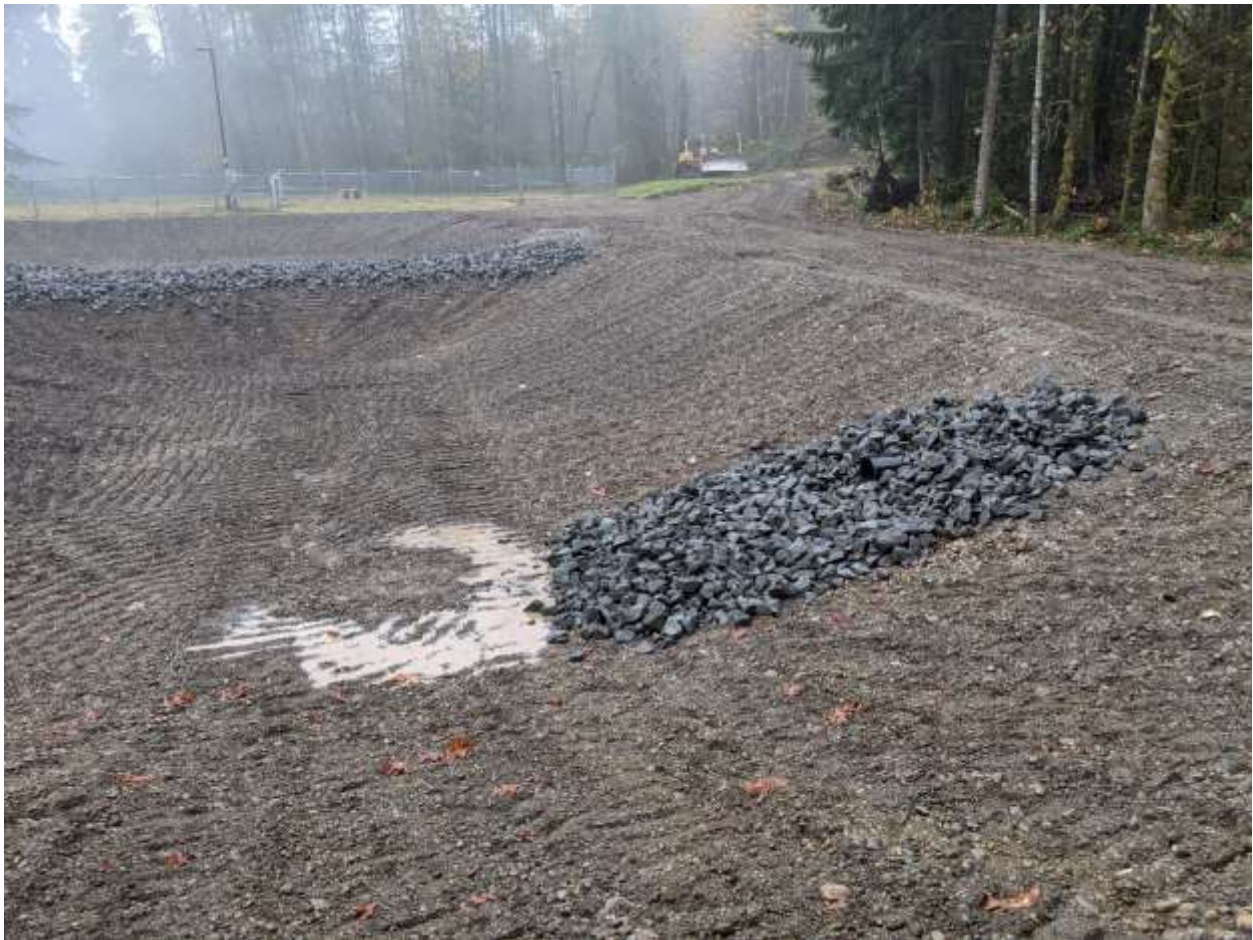
Photograph 7 – View of Infiltration Pond installed at the North End.
