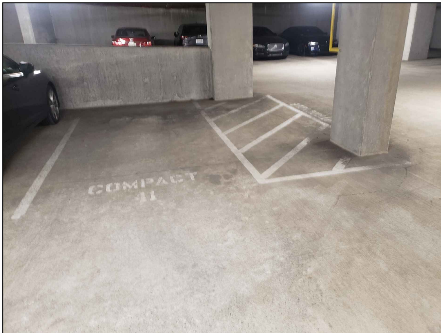
Photograph 4: View looking south at the garage floor slab overlying Area 2.
