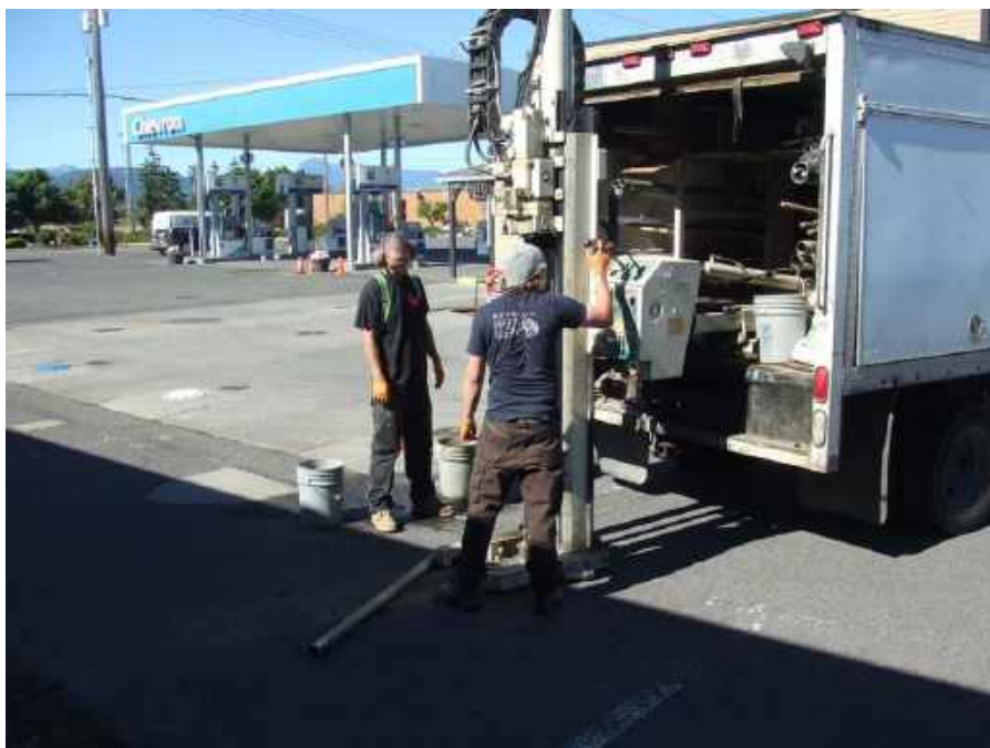
Photo 10. A view of the soil boring – B2.
