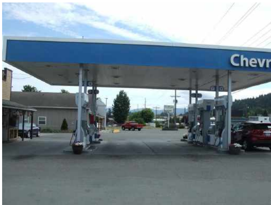
Photo 3. A view of the canopy and dispensers looking southeast.
