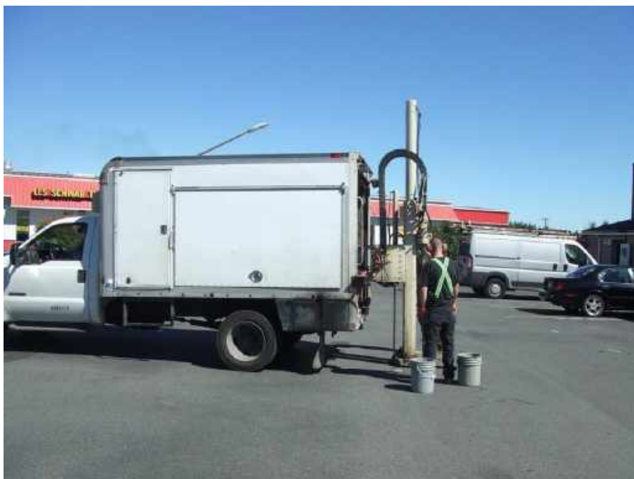
Photo 14. A view of the soil boring – B6.
