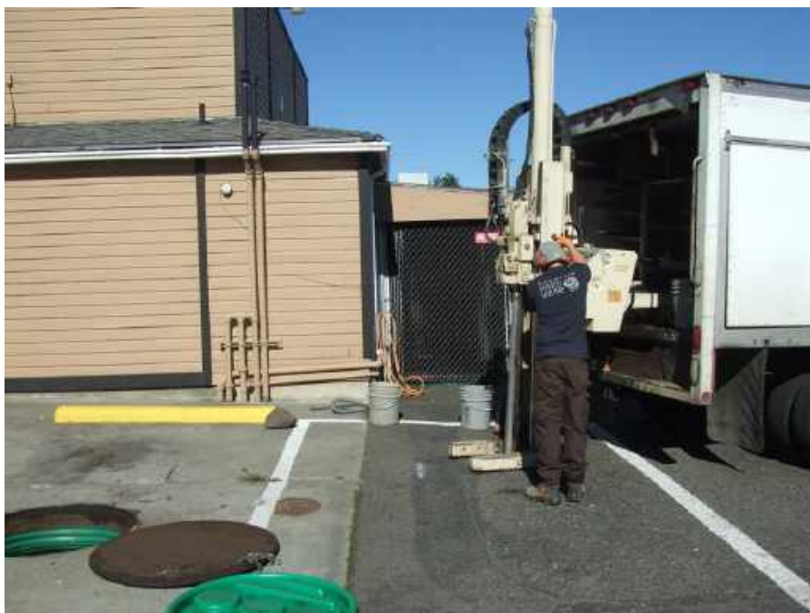
Photo 9. A view of the soil boring – B1.
