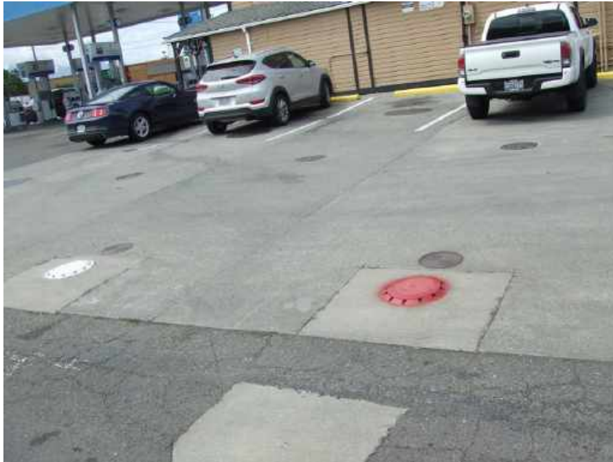
Photo 5. A view of the UST pad looking northwest.
