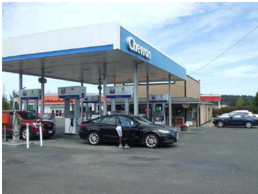
Photo 2. A front view of the Subject Property looking northeast.
