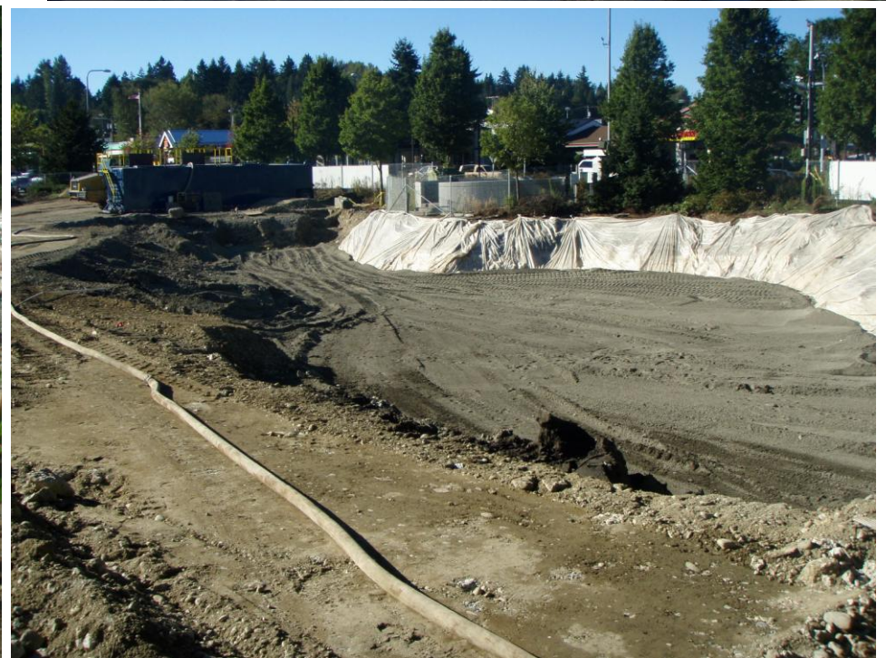
DURING EXCAVATION (TOP) & DURING BACKFILL AND ORC + VISQUEEN BARRIER APPLICATION (BOTTOM)
