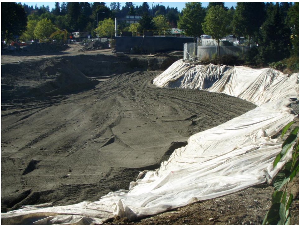
DURING EXCAVATION (TOP) & DURING BACKFILL AND ORC + VISQUEEN BARRIER APPLICATION (BOTTOM)
