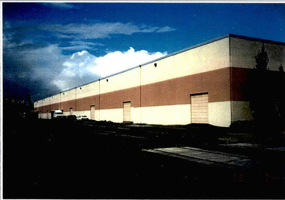
Photo A. West side of Building C looking north.
