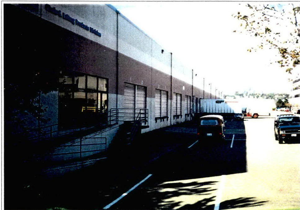
Photo B. East side of Building C looking north.
