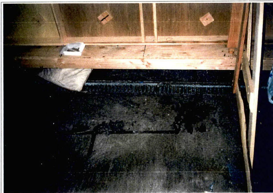
Photo G. Floor drains in vacant half of Building E, formerly occupied by U.S. West.
