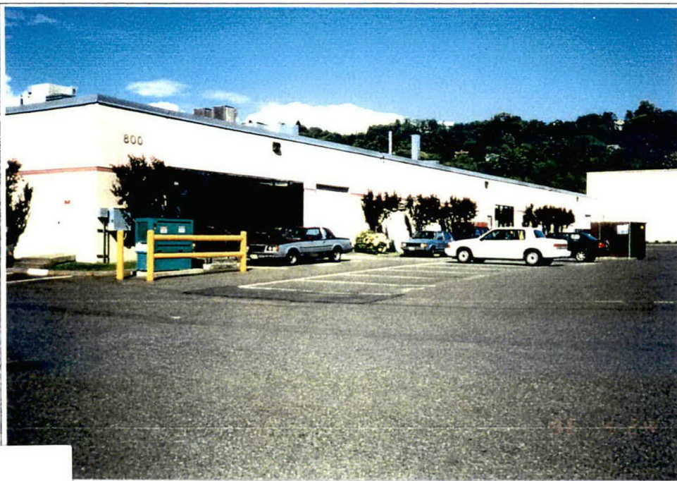
South side of Building D looking northeast. Probe P-5 is located near the white car.
