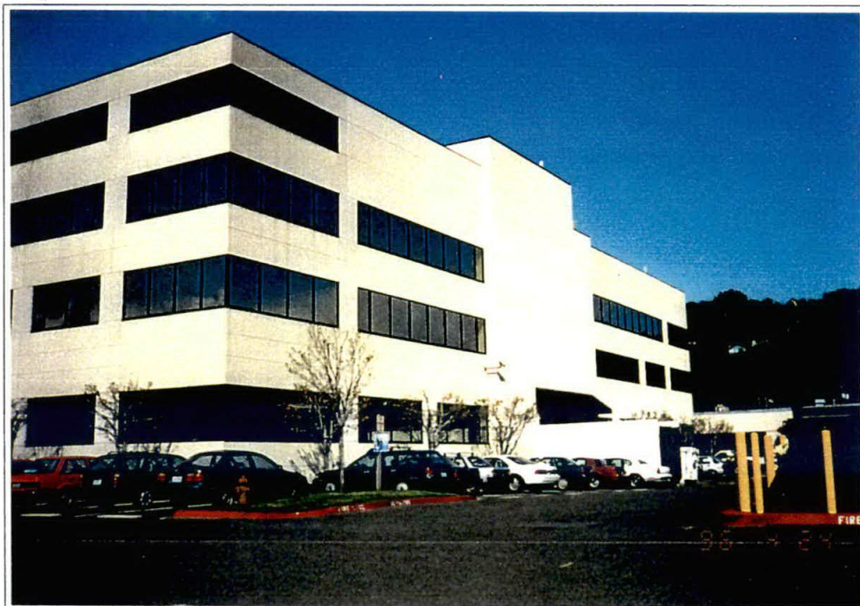
Photo D. South side of Building A looking northeast.
